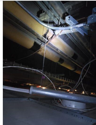
8" Tan Pipe – Asbestos containing black tar wrapping
