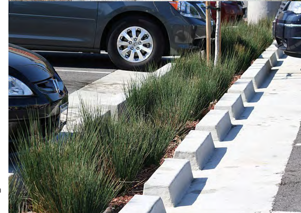
Figure 3.9 Cut curb swale design
