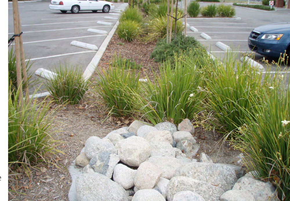
Figure 3.8 Parking lot swale
