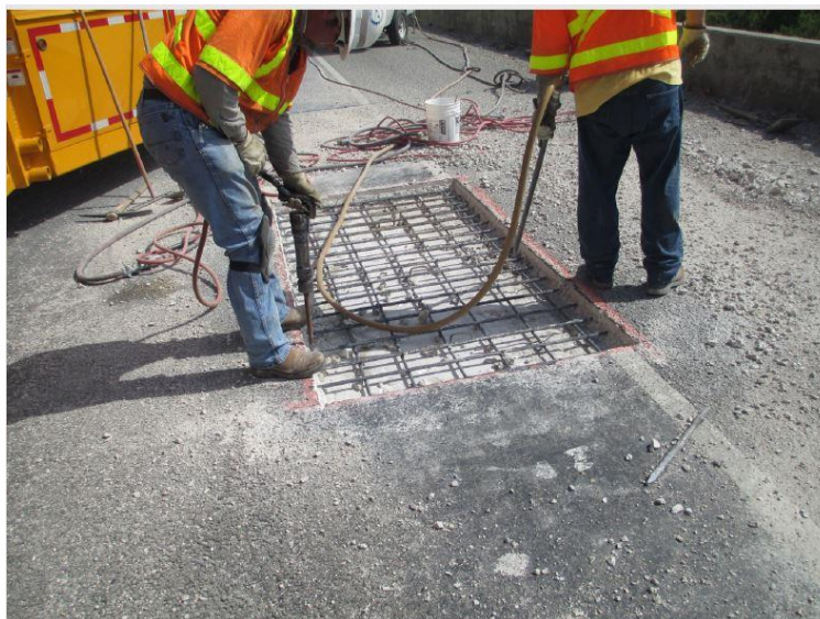
Figure 9.18 Bridge Deck Repair Procedure
