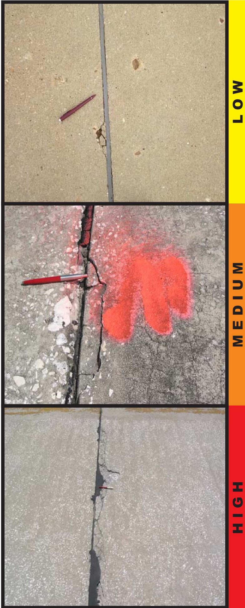
74 SPALLING, JOINT
