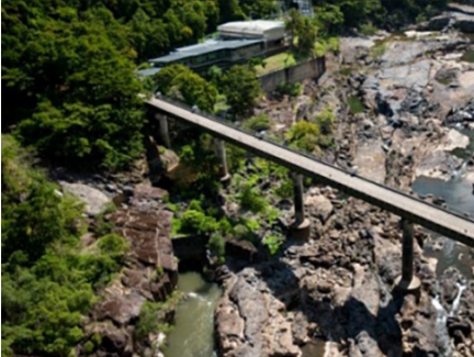
BARRON GORGE HYDRO POWER STATION
