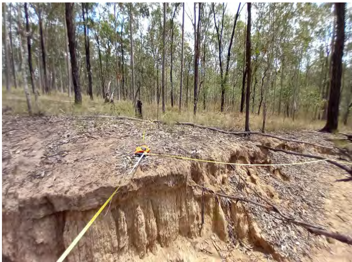
Plate 3 Erosion 1 south view.
