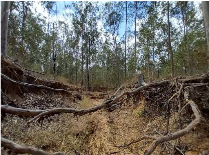
Plate 7 Erosion 2 east view.
