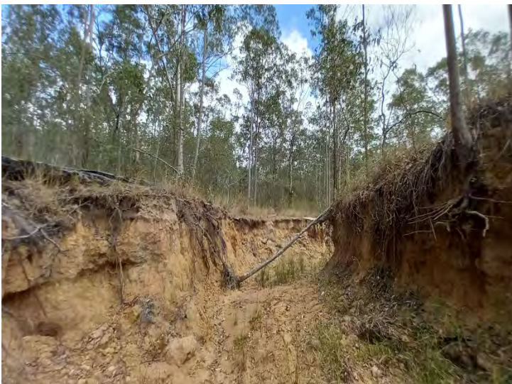
Plate 9 Erosion 2 west view.
