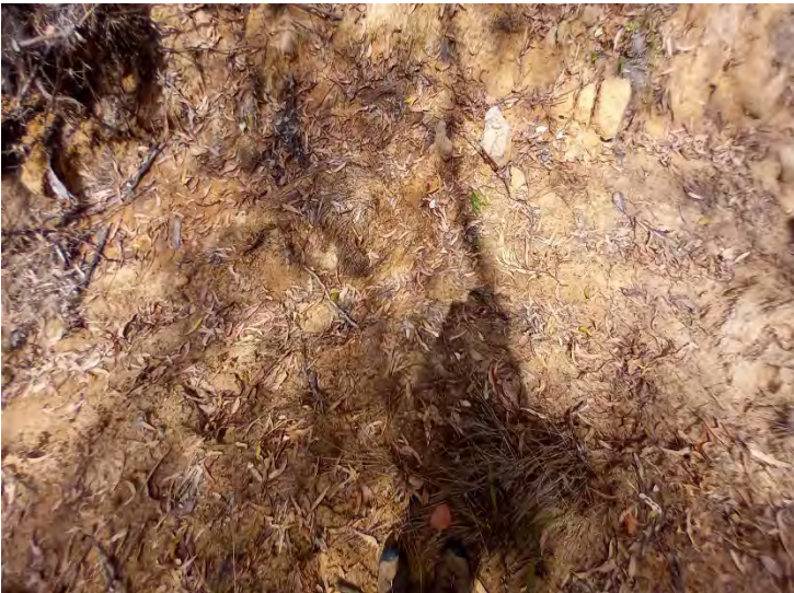
Plate 15 View of soil at Erosion 3.
