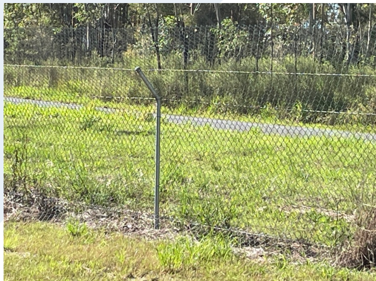
Fence after weed treatment (17 March 2025)
