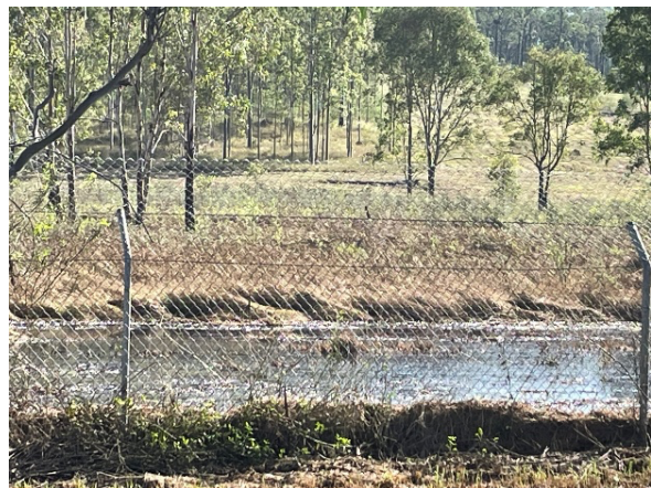
Standing water on pipeline easement within property – taken from Ford’s Road
