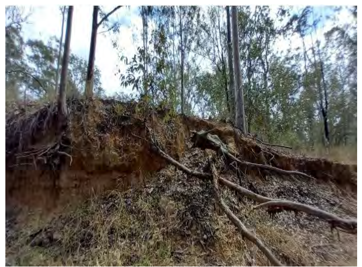
Plate 6 Erosion 2 north view.
