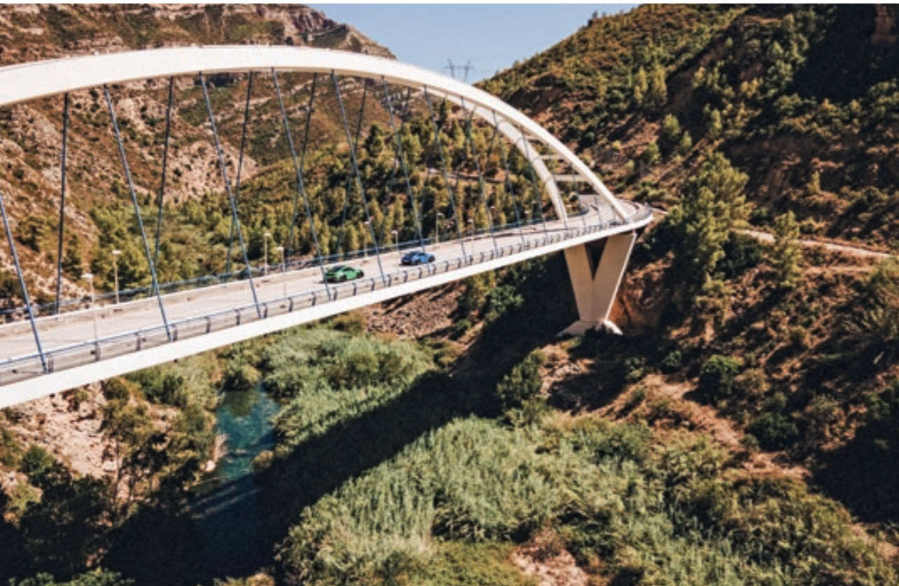
Aesthetic bridging: Not far from the town of Dos Aguas, modern street architecture merges into a wild landscape.
