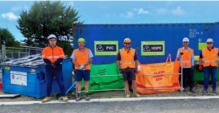
Construction waste diversion at Casebrook construction site
