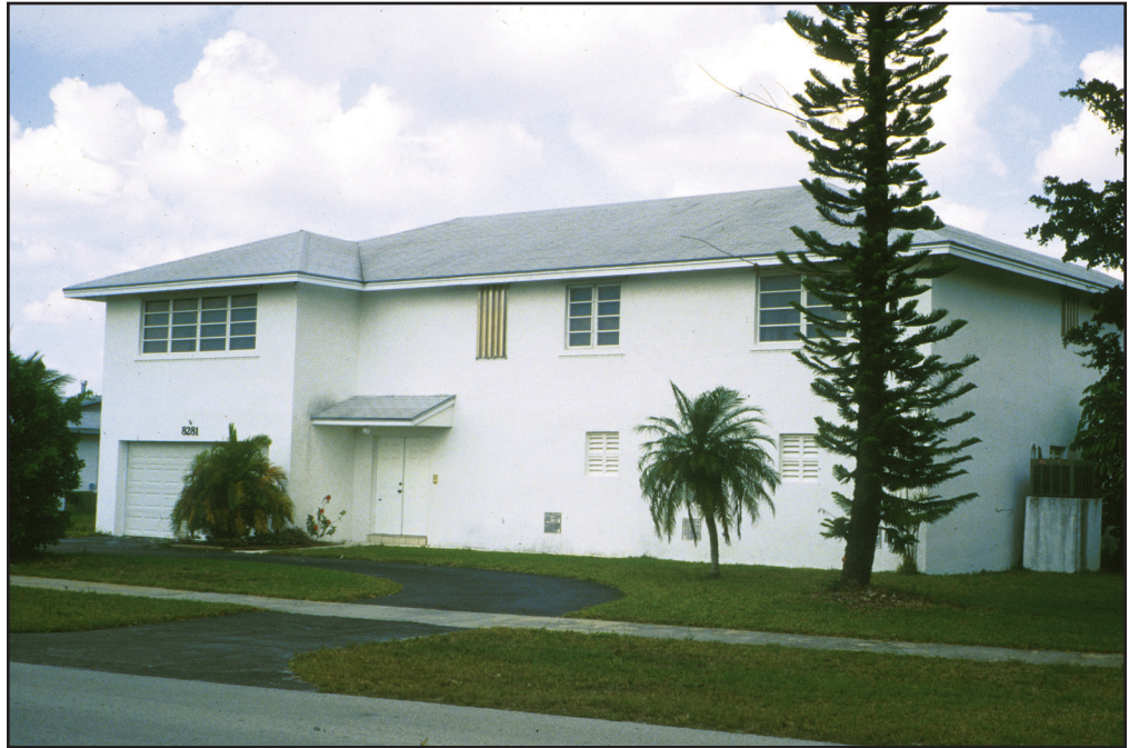
Figure 64 From the outside, the completed house, with its stucco walls, looks like a conventional masonry house.
