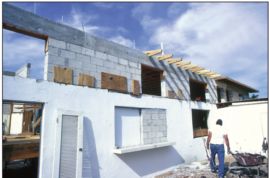
Figure 67 The extended first-story walls.
