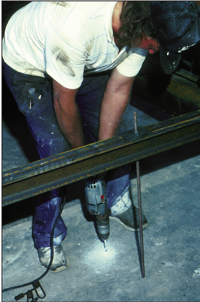
Figure 77 ... install anchors ...
