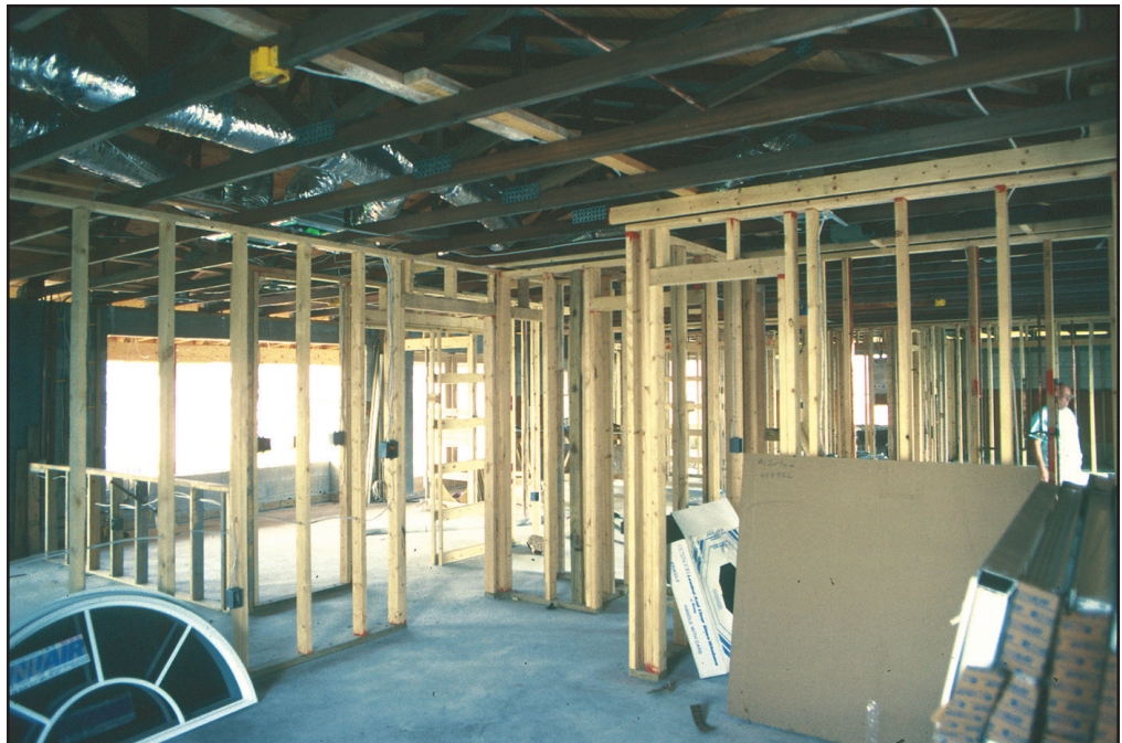
Figure 30 Interior partition walls and utilities are added.
