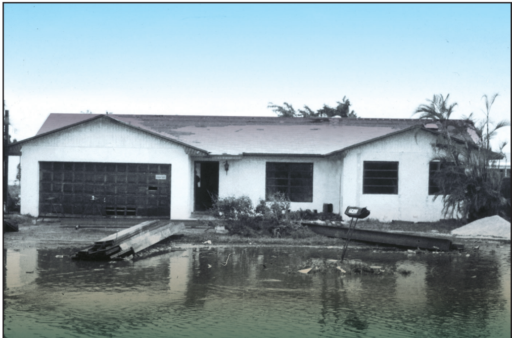
Figure 73 Like the houses shown previously, this one-story house, with its concrete block walls, concrete slab foundation, and attached garage, is typical of the houses in the area affected by Hurricane Andrew.
