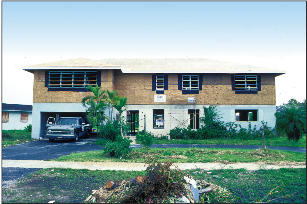
Figure 62 After the wood framing was completed, the roof and exterior wall sheathing were added.
