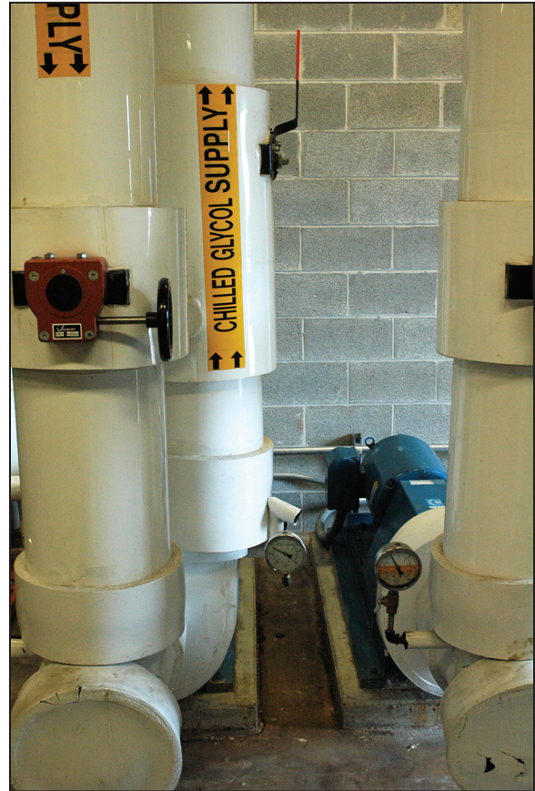
Figure 5-4. Chilled water pump, Georgetown, Delaware.
