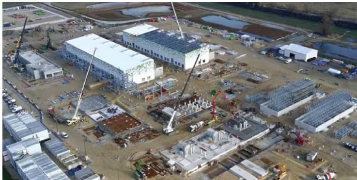
AIR LIQUIDE Saint-Jean-de-Folleville - France Execution of the electricity and instrumentation package for a 200 MW electrolyzer for green hydrogen production. By Snef
