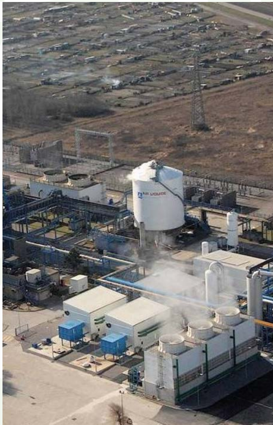
AIR LIQUIDE France Basic engineering studies (FEED) to extend the service life of existing units by at least 15 years. By Ekium
