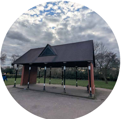
Cale Green Park Pavilion
