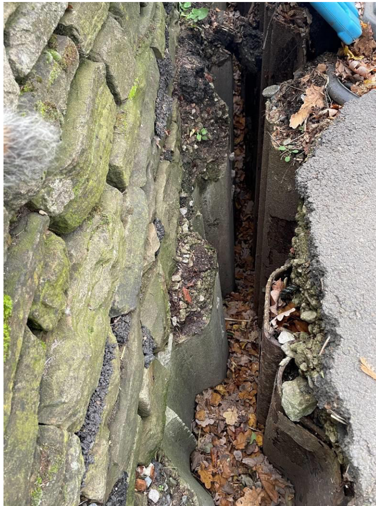
View looking down gap between sheet piles and RC wall, January 2023
