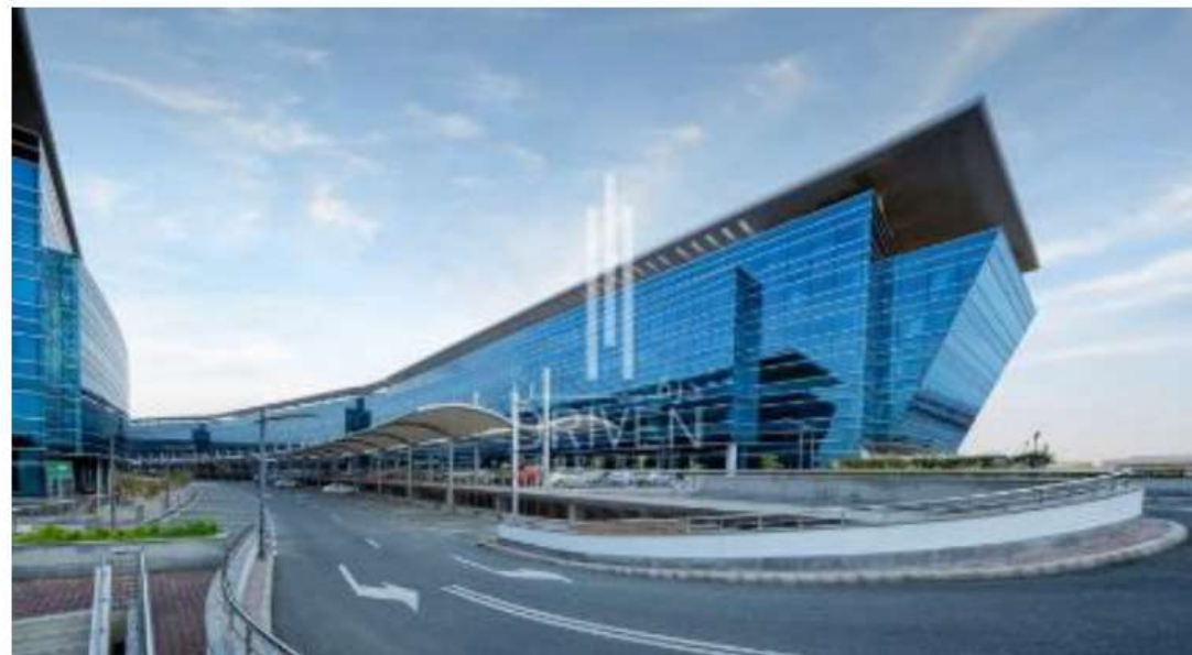
Fig. 25: Existing Business Center at Dubai South
