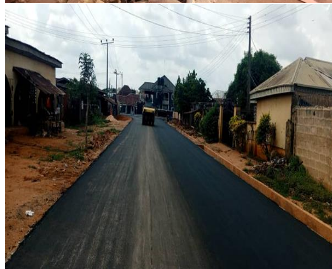
Construction of 19 th Street, Ugbowo B/C
