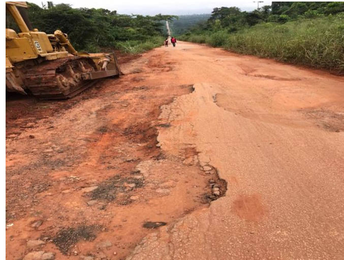
Reconstruction of Ujiogba-Ogwa Road
