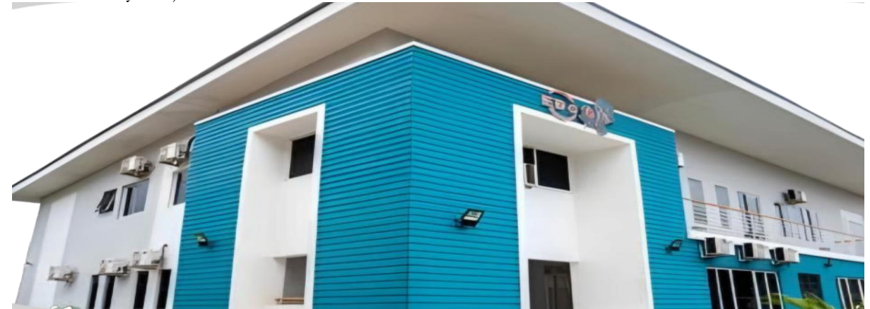
EdoGIS Administrative Building
