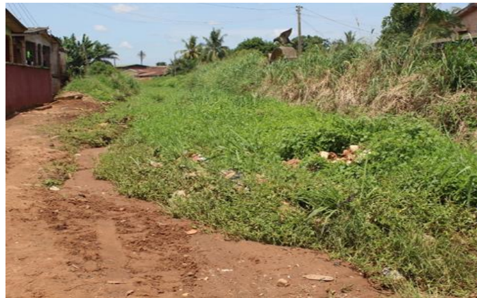
Construction of Textile Mill Road, B/C
