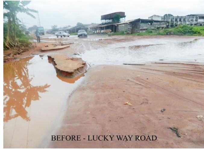
Construction of Lucky Way, Ikpoba-Hill, B/C
