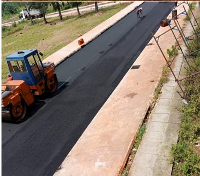
Construction of Gstc Internal Roads, B/C
