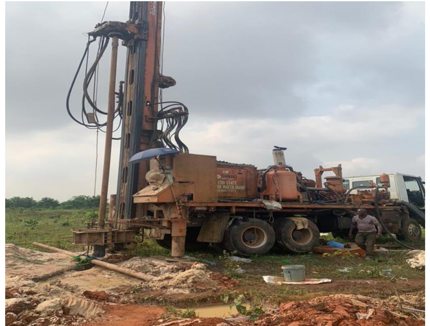
Construction of 2Nos. Industrial Boreholes at Emotan Garden Estate
