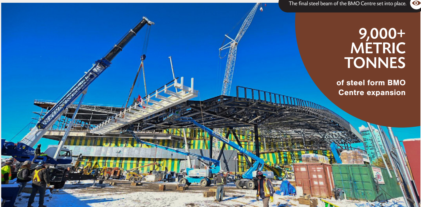
The final steel beam of the BMO Centre set into place.
