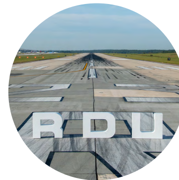
Replacement of Runway 5L/23R
