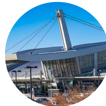
Terminal 2 Landside Expansion
