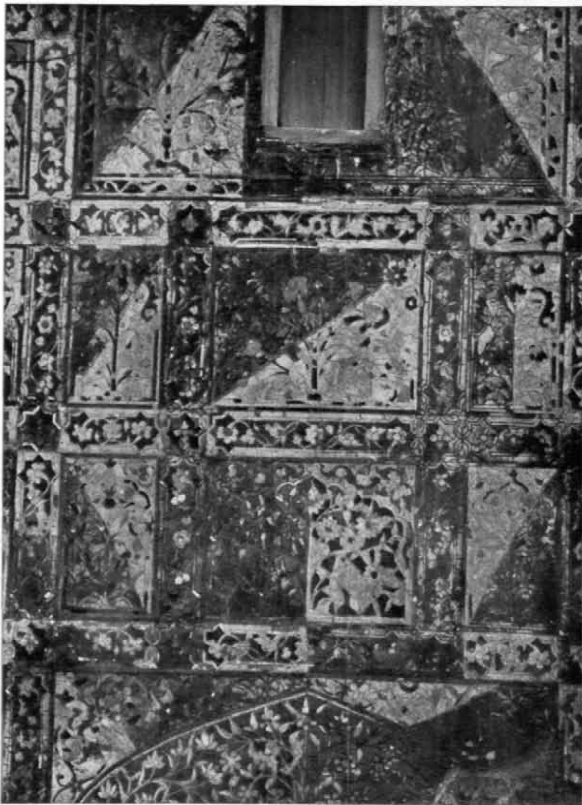
Agra : Chini-Ka- Rauza, tilework on eastern wall, during treatment. See p. 147
