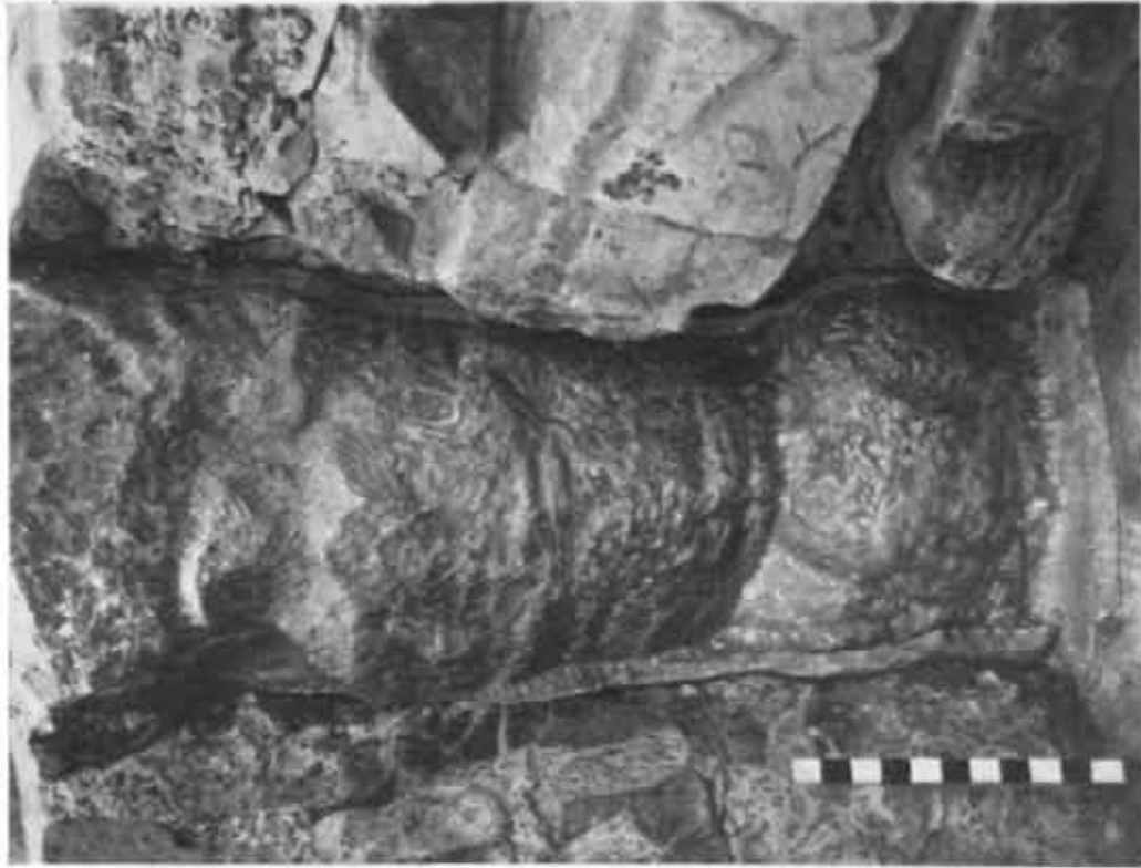
Delhi : Quwwatu'l-Islam mosque, iron pillar, base, A, after preservation, and B, details of lead sheet inserted at base. See p. 124
