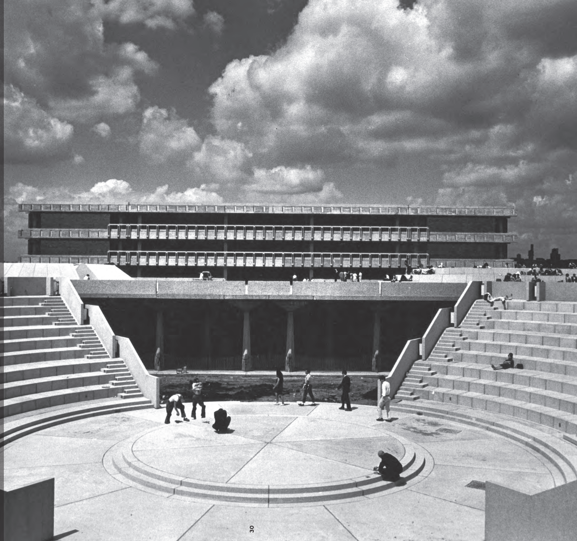
THE CAMPUS DESIGN BY ARCHITECT WALTER NETSCH, IS BASED ON THE METAPHOR OF A STONE DROPPED IN A POND OF WATER WHERE THE CIRCLE FORUM AND LECTURE CENTERS REPRESENT THE CENTER OF LEARNING, THE PLACE WHERE STUDENTS AND THEIR TEACHERS GATHER TO DISCUSS IDEAS. PHOTO: ORLANDO CABANBAN
