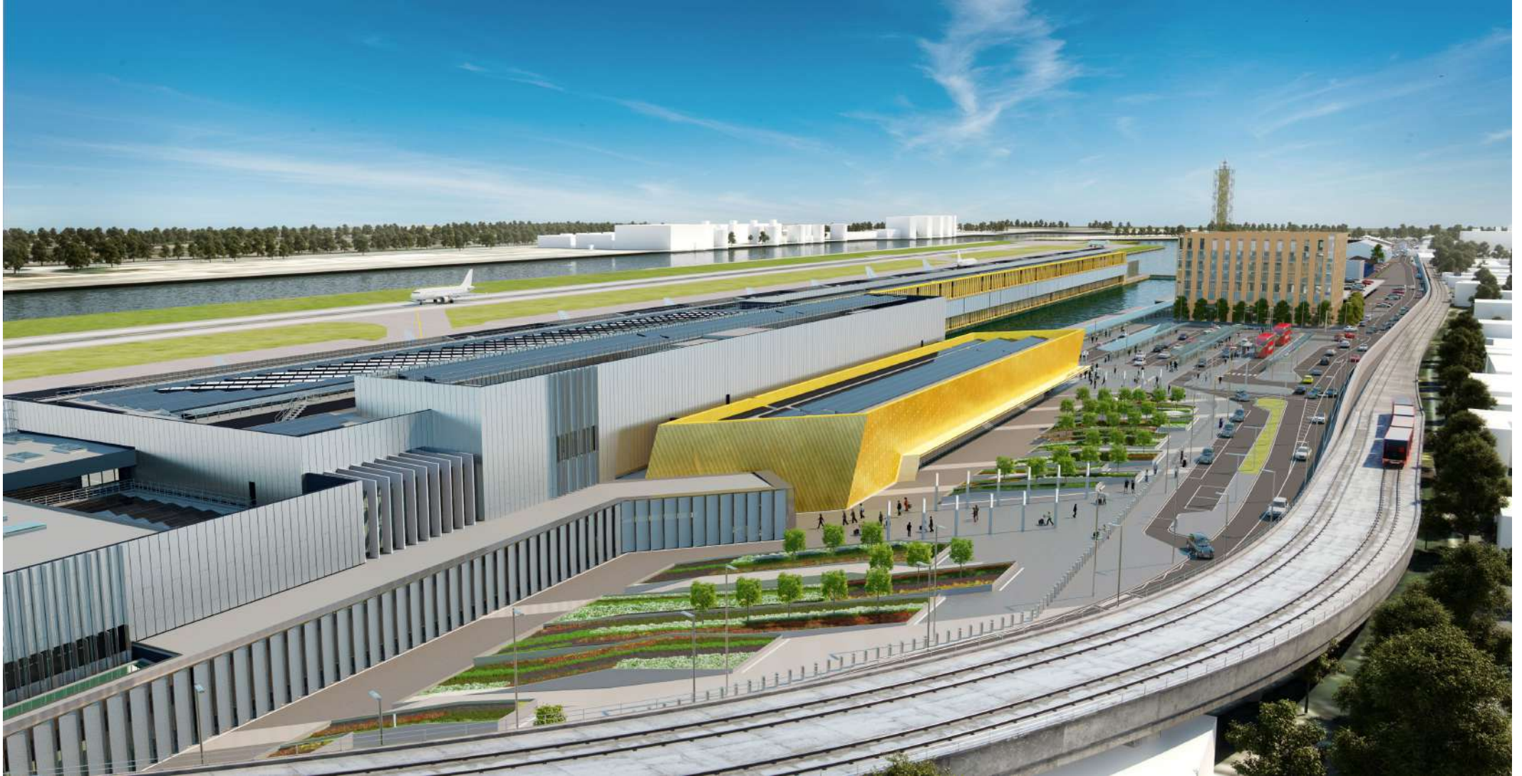
Figure 1.4.3: View of CADP terminal and new passenger forecourt
