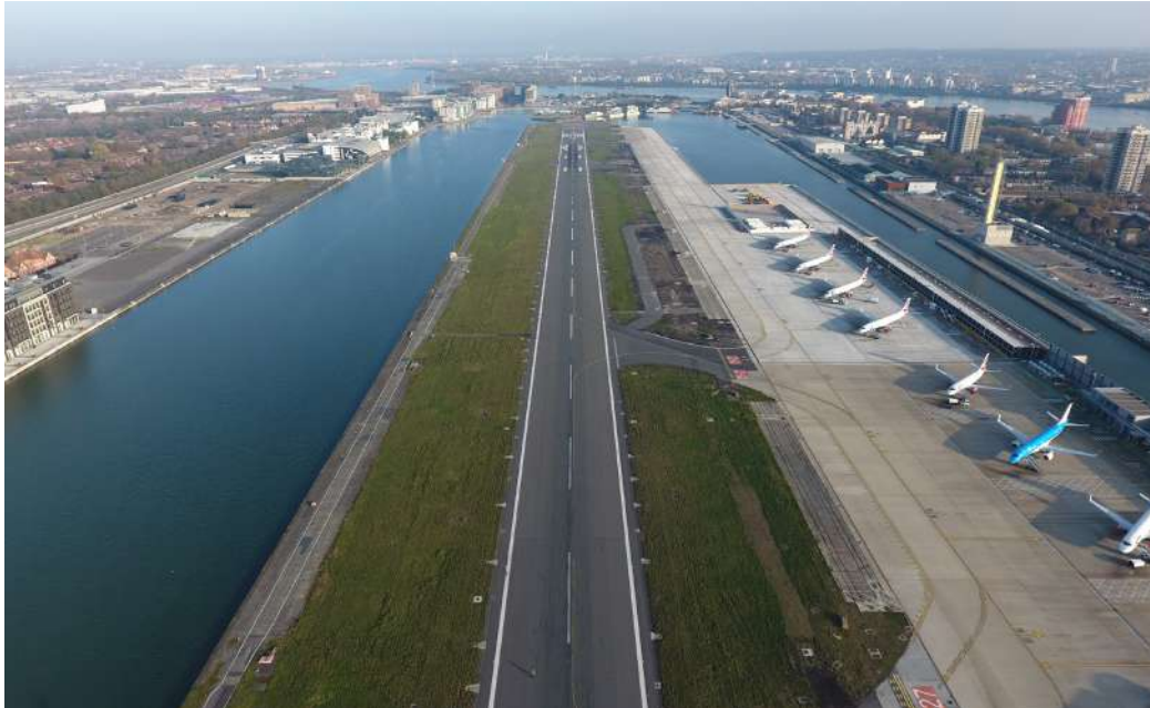
Figure 1.4.1: Aerial view of recently completed parallel taxiway and larger aircraft stands
