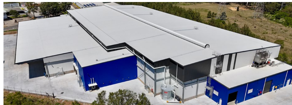
Minchinbury, New South Wales, Australia
