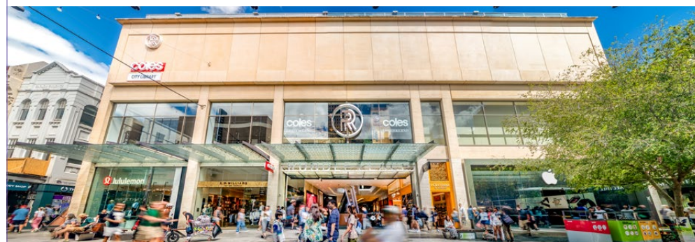
Rundle Place, Adelaide, South Australia
