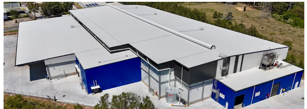
Minchinbury, New South Wales, Australia
