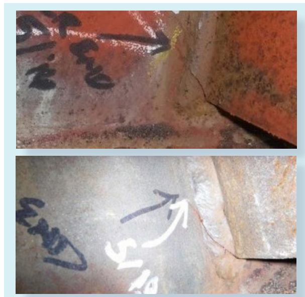
Figure 11: Examples of Base Metal Cracks on Existing Flyovers
