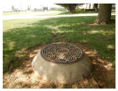
Photo 16: Sanitary sewer utility manhole located near the CAE Dallas West Training Center and is representative of the type of utilities located near the eastern terminus.
