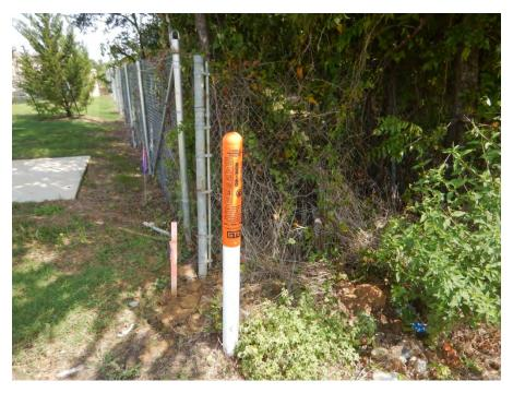
Photo 6: Buried cable indicator pole located at the western project terminus, on the north side of Glade Road.
