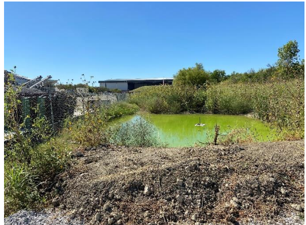
Photograph 22. Detention area within Staging Area 1 north of East 28 th Street and East Airfield Drive.
