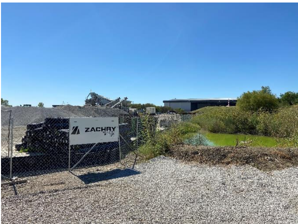
Photograph 23. Staging Area 1 fence and detention area.
