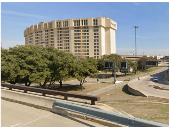
Photograph 5. Photograph image of the Terminal C Garage roadway.
