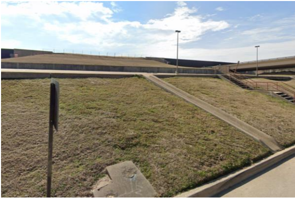
Photograph 7. Photograph image of the cross under south of Terminal E.
