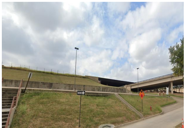
Photograph 6. Photograph image of the cross under south of Terminal E.
