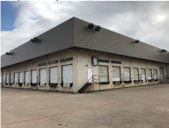
Photograph 5 - Evergreen Facility, View to the Southeast
