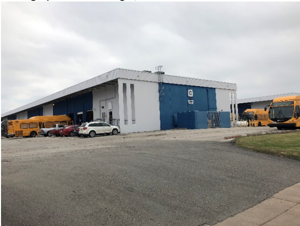
Photograph 47 – Building C, View to the Southeast
