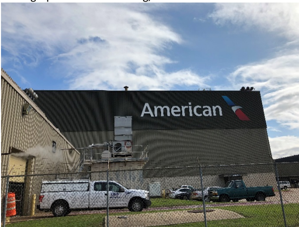
Photograph 21 – AA Hangar, View to the East
