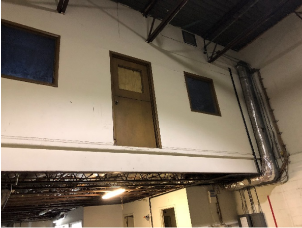
Photograph 59 – Building C, Interior
