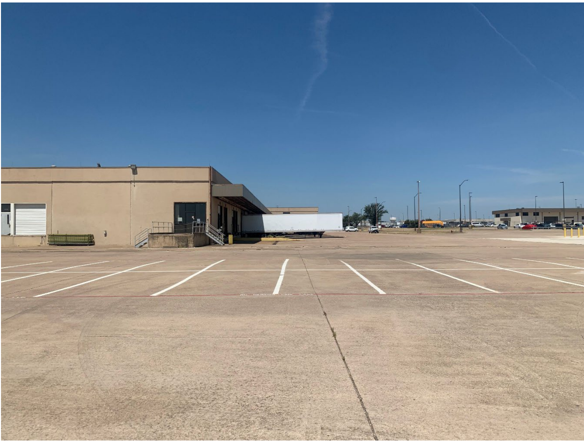
Photograph 9: American Airlines West Warehouse, north and east elevations, facing west.
