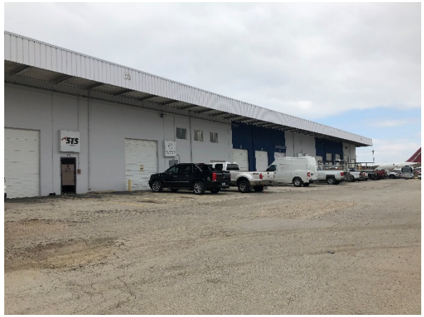
Photograph 50 – Building C, View to the Southeast
