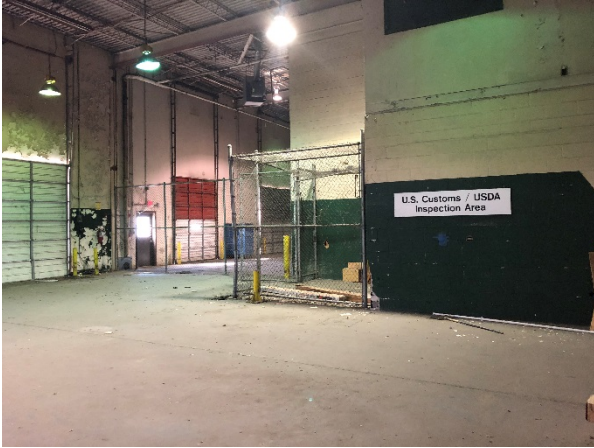
Photograph 19 – Evergreen Facility, Interior
