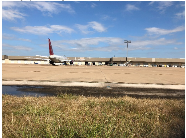
Photograph 8 - Evergreen Facility, View to the North
