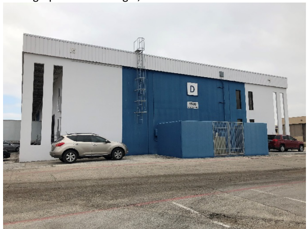
Photograph 62 – Building D, View to the East
