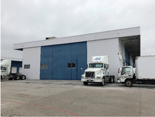
Photograph 27 – Building A, View to the West
