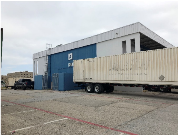
Photograph 25 – Building A, View to the Northeast
