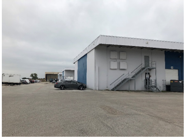
Photograph 36 – Building B, View to the South
