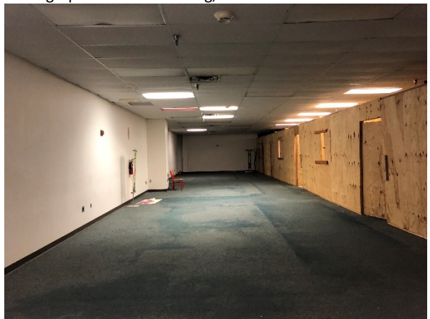
Photograph 16 – KHA Building, Interior
