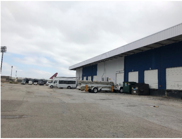
Photograph 49 – Building C, View to the Northeast
