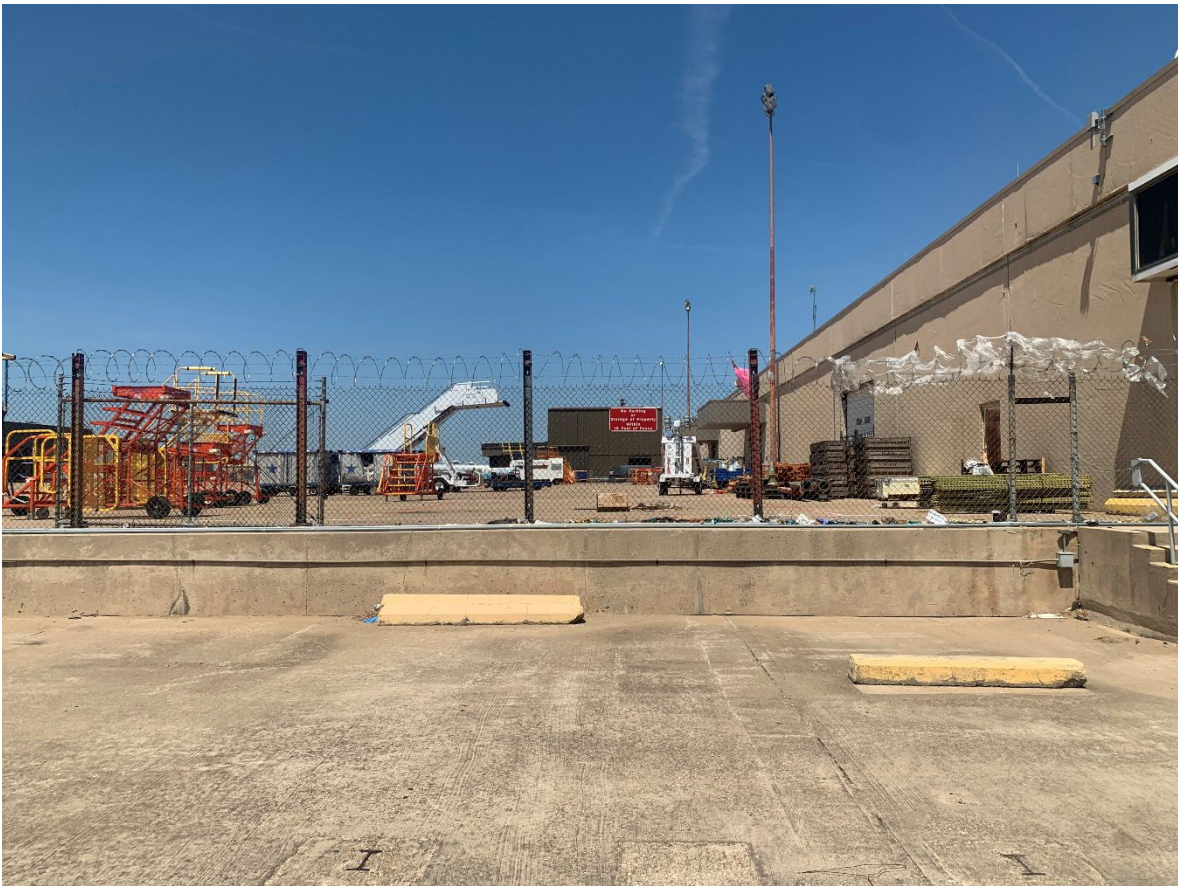
Photograph 12: American Airlines West Warehouse, south and east elevations, facing west.
