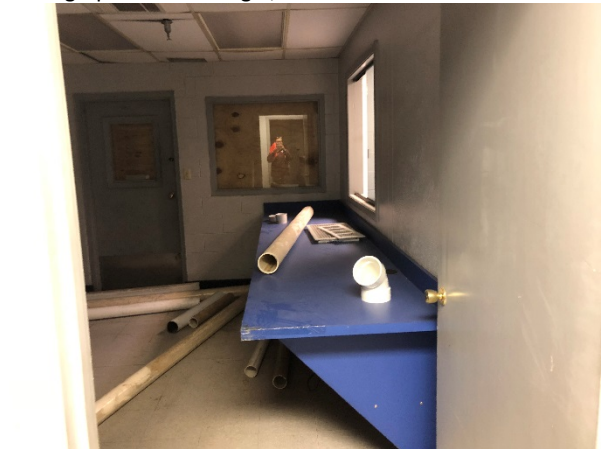
Photograph 46 – Building B, Interior
