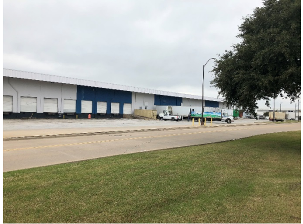
Photograph 28 – Building A, View to the South
