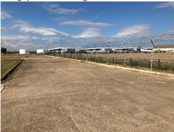
Photograph 13 – KHA Building, View to the West
