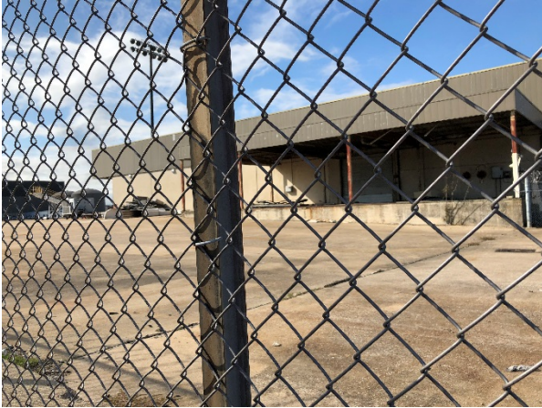
Photograph 11 - Evergreen Facility, View to the West
