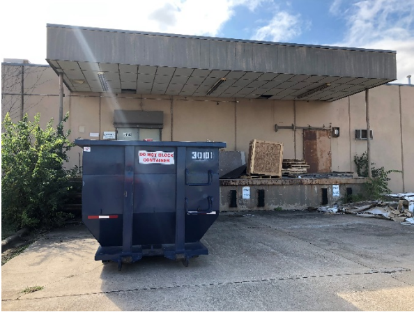
Photograph 11 – KHA Building, View to the South
