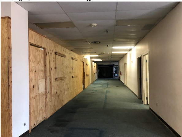
Photograph 15 – KHA Building, Interior
