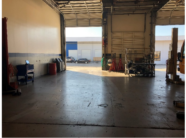
Photograph 52 – Building C, Interior
