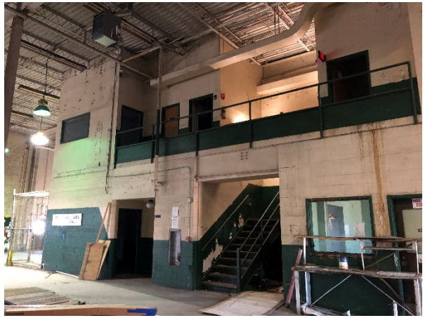
Photograph 18 – Evergreen Facility, Interior
