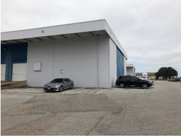
Photograph 35 – Building B, View to the North
