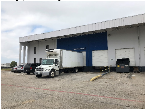
Photograph 64 – Building D, View to the North
