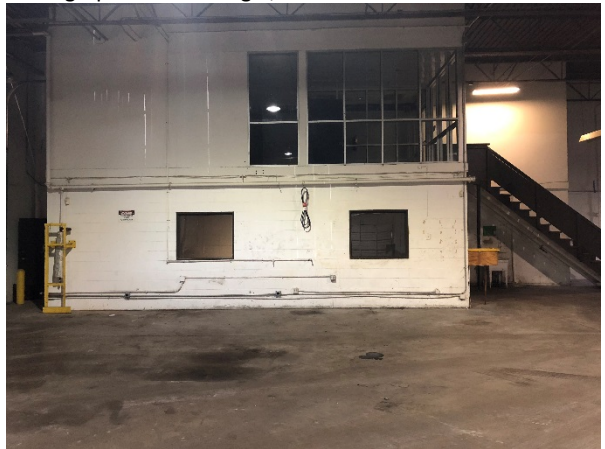
Photograph 56 – Building C, Interior
