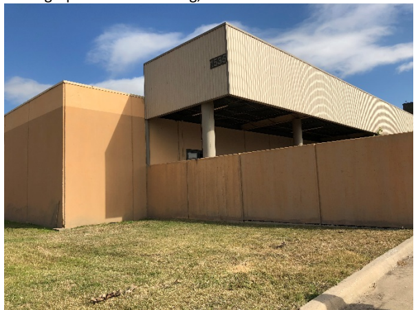
Photograph 6 – KHA Building, View to the Northeast
