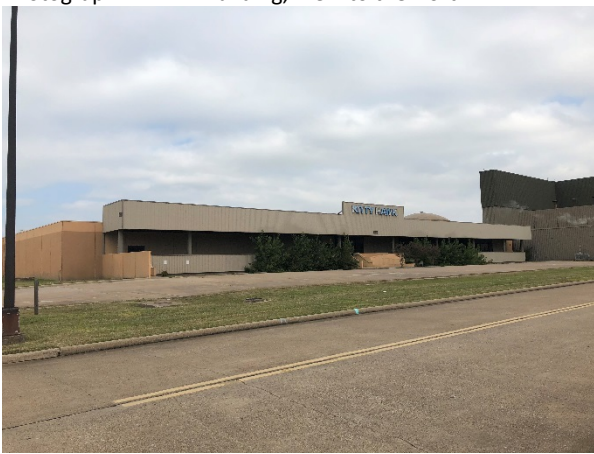
Photograph 3 – KHA Building, View to the Northeast
