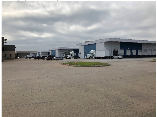
Photograph 24 – Building A, B, C, & D, View to the Southwest
