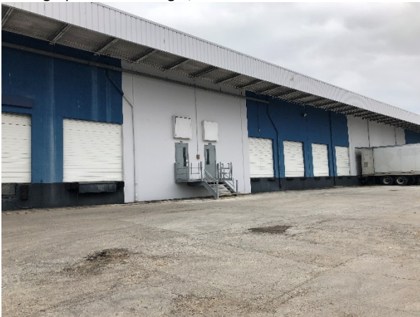
Photograph 37 – Building B, View to the South
