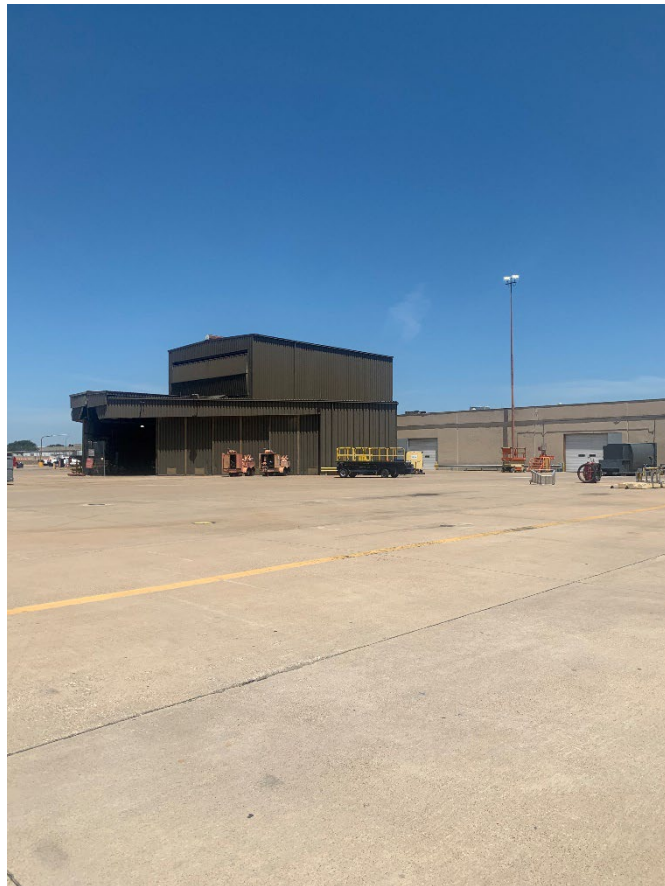
Photograph 16: American Airlines West Warehouse, south (western section) elevation, facing northeast.
