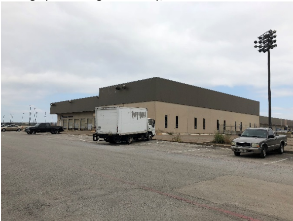
Photograph 7 - Evergreen Facility, View to the Northwest
