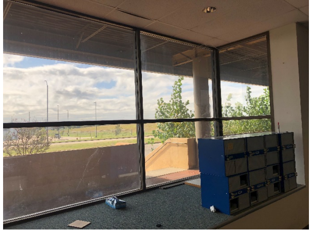
Photograph 20 – KHA Building, Interior
