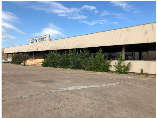
Photograph 2 – KHA Building, View to the Northwest
