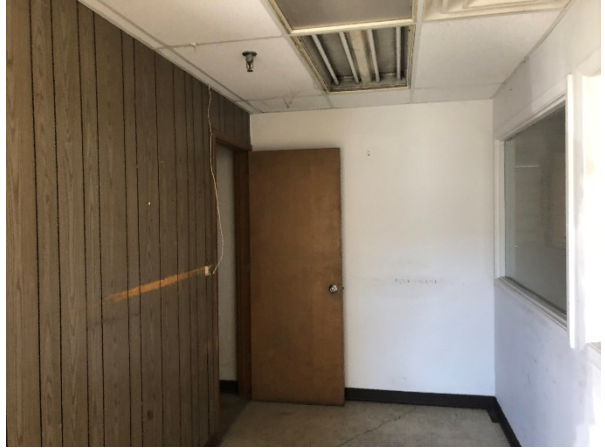
Photograph 60 – Building C, Interior
