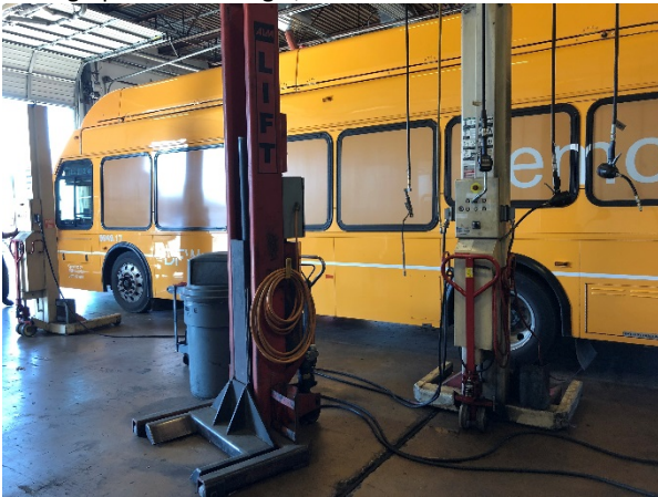
Photograph 53 – Building C, Interior
