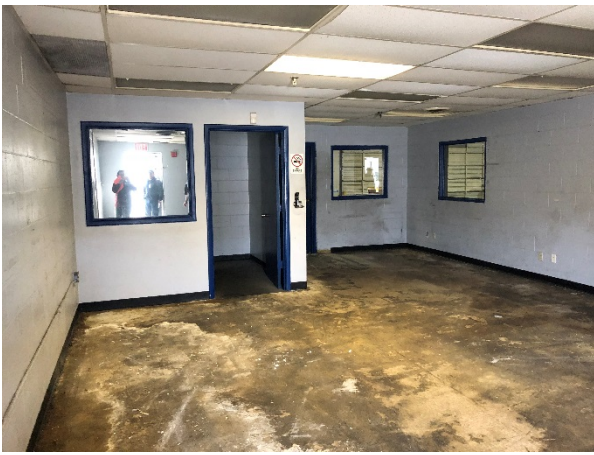
Photograph 57 – Building C, Interior
