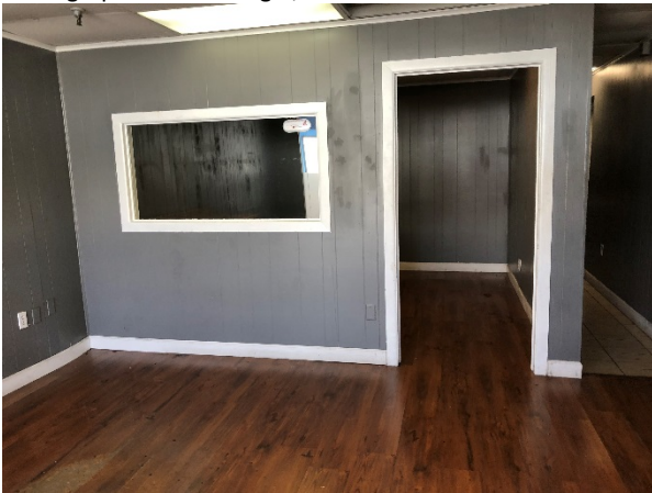
Photograph 39 – Building B, Interior
