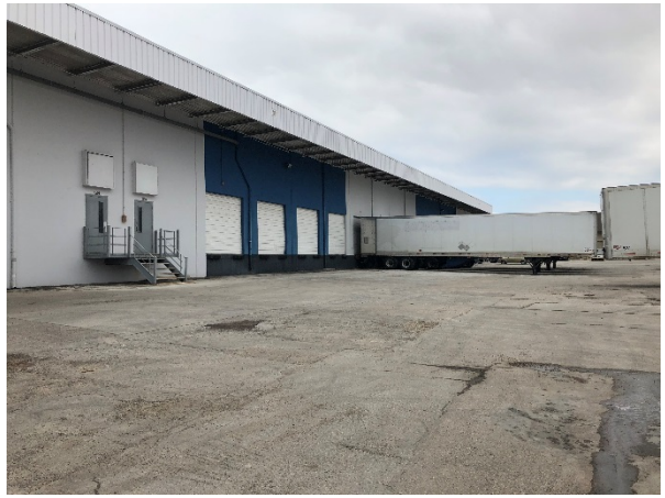
Photograph 26 – Building A, View to the East
