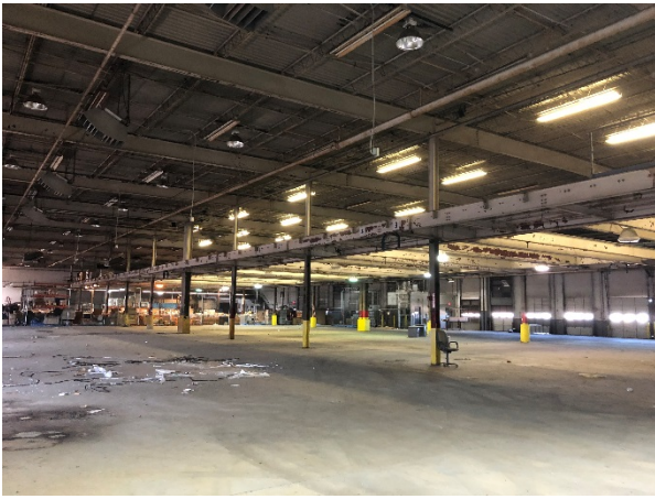
Photograph 17 – Evergreen Facility, Interior
