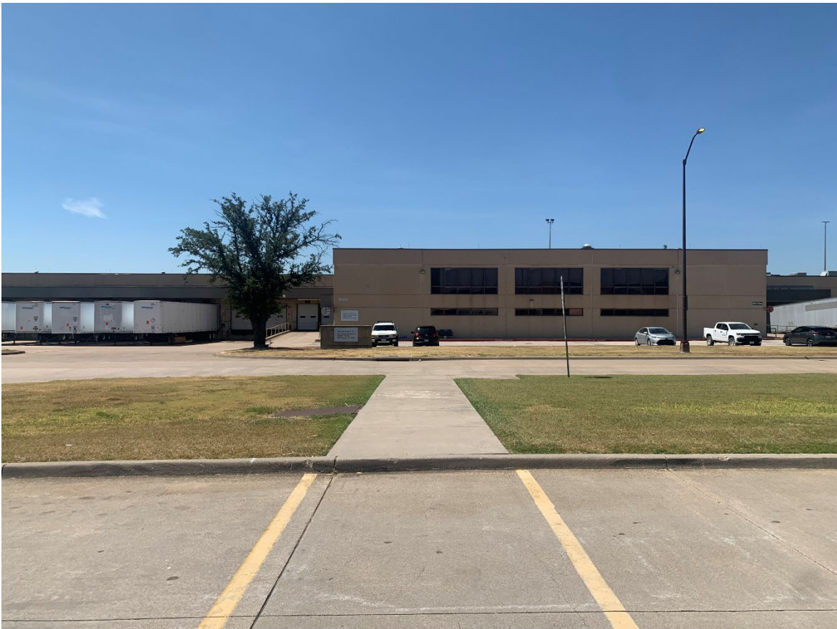
Photograph 6: American Airlines West Warehouse, north (center section) elevation, facing south.
