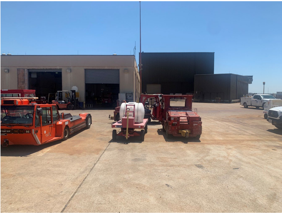
Photograph 17: American Airlines West Warehouse, south and west elevations, facing east.
