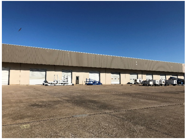
Photograph 10 - Evergreen Facility, View to the North
