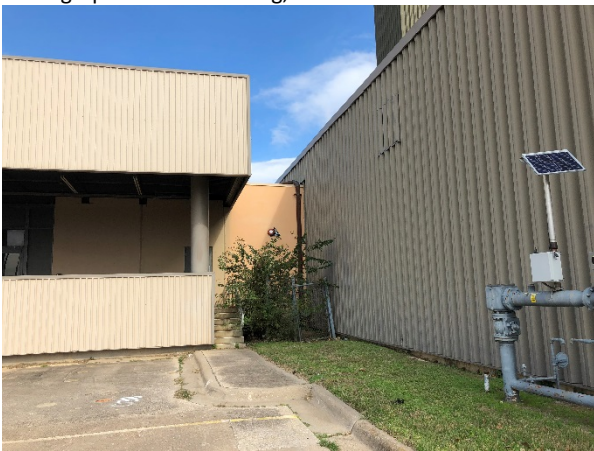
Photograph 5 – KHA Building, View to the North
