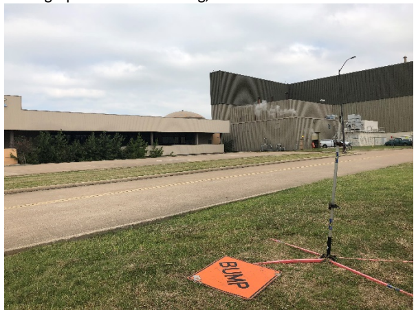
Photograph 22 – AA Hangar, View to the Northeast
