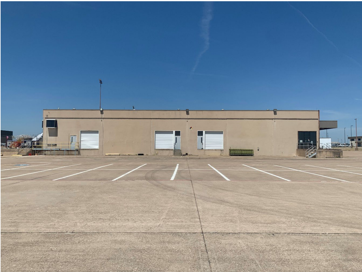
Photograph 10: American Airlines West Warehouse, east elevation, facing west.
