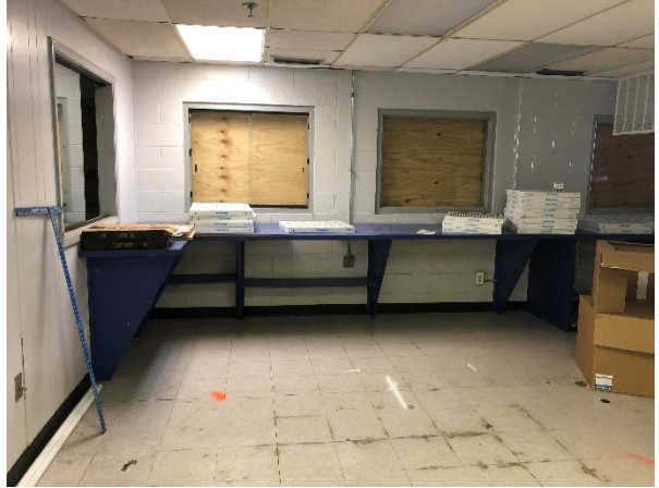
Photograph 44 – Building B, Interior
