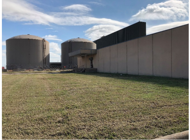
Photograph 12 – KHA Building, View to the Southeast
