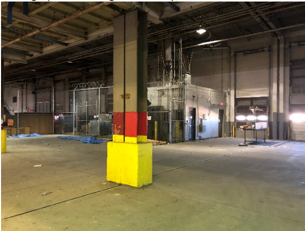
Photograph 15 - Evergreen Facility, Interior
