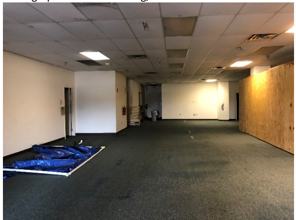
Photograph 14 – KHA Building, Interior
