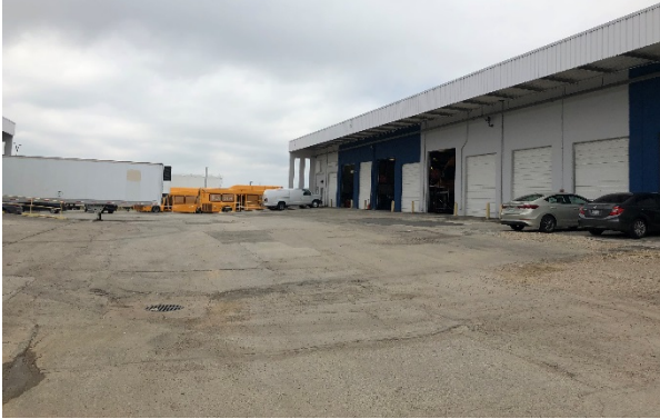
Photograph 51 – Building C, View to the Northwest
