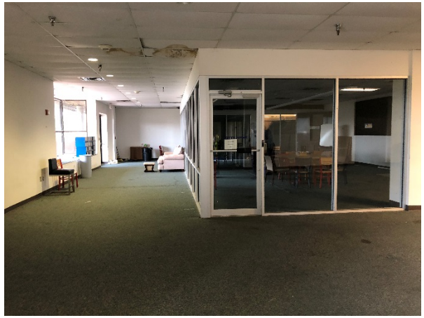
Photograph 18 – KHA Building, Interior
