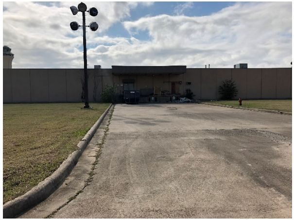
Photograph 10 – KHA Building, View to the South
