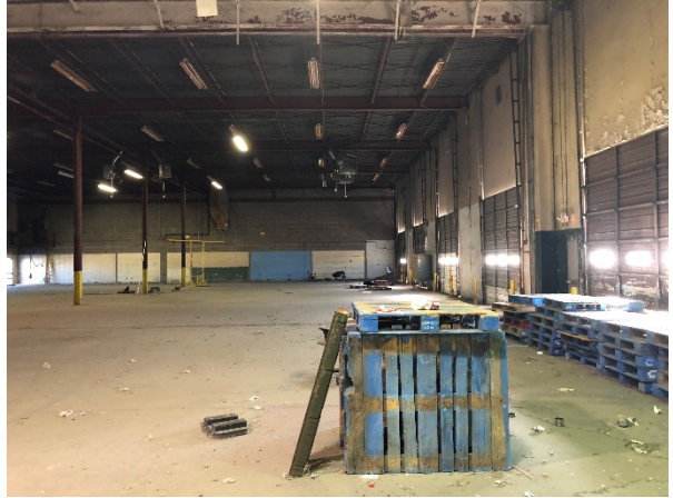
Photograph 20 – Evergreen Facility, Interior
