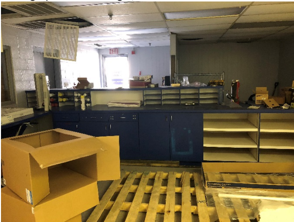
Photograph 45 – Building B, Interior
