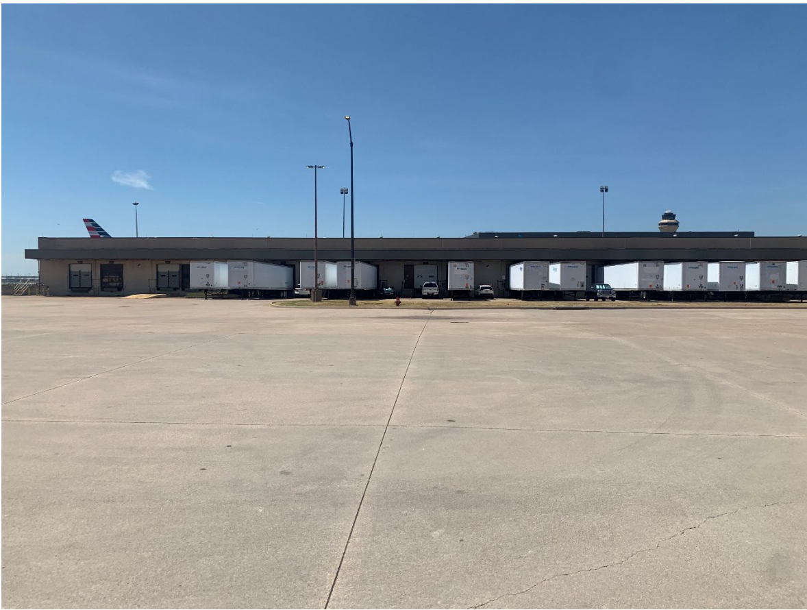
Photograph 7: American Airlines West Warehouse, north (eastern section) elevation, facing south.
