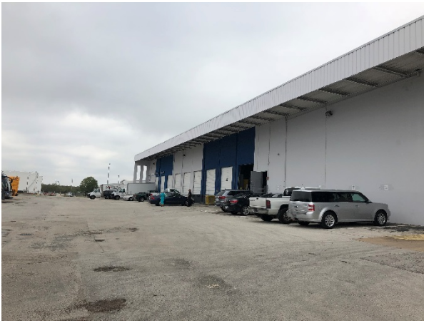
Photograph 33 – Building B, View to the Northwest
