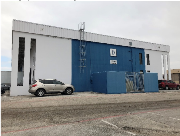
Photograph 23 – Building D, View to the East
