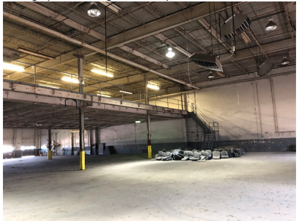
Photograph 16 - Evergreen Facility, Interior
