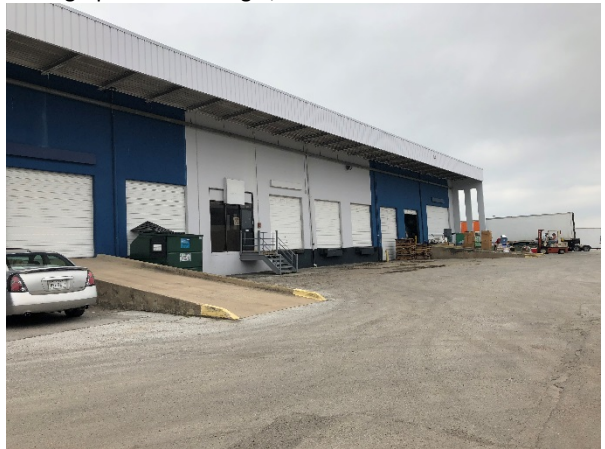
Photograph 38 – Building B, View to the Southwest
