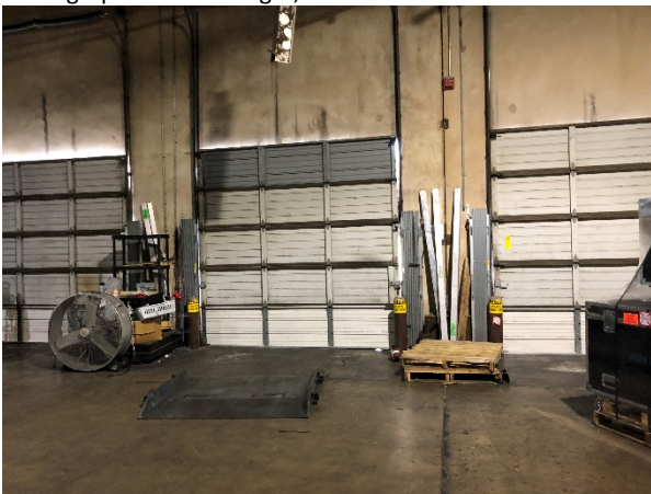
Photograph 69 – Building D, Interior
