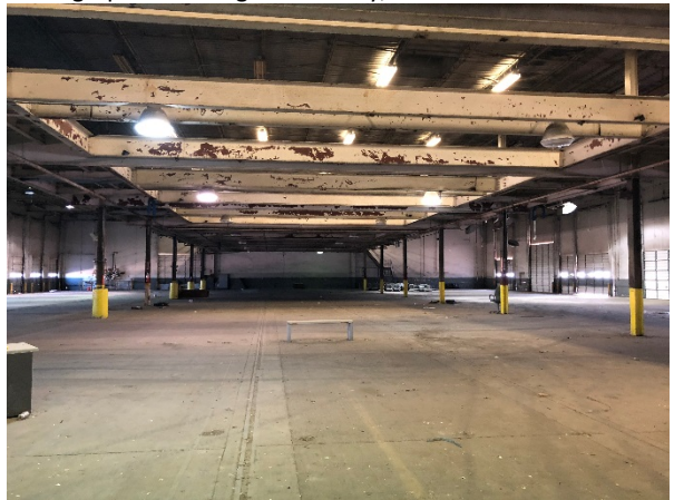
Photograph 14 - Evergreen Facility, Interior
