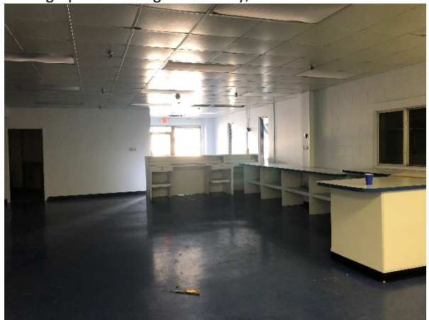
Photograph 22 – Evergreen Facility, Interior
