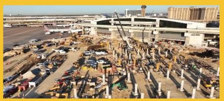
4/2/25: DFW's inno vative mindset and the use of modular construction has taken core construction activity away from the busy DFW Terminals to a separate pre-fabrication site where the construction teams have made major headway on building the expansions coming to both Terminal C and Terminal A. When ready, these modules will be transported across the airfield, and set into place at the terminals.
