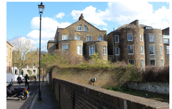
2 - Cleaver Square Rear facade with curved bay windows. 5 Storeys
