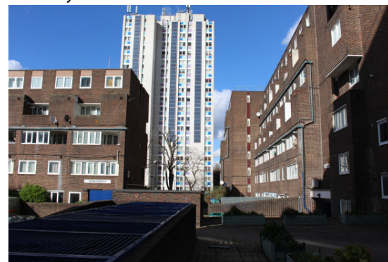
5 - Ethelred Estate 60s/70s public housing in dark brown brick and arranged in stacked maisonettes with 3 point blocks over 20 storeys
