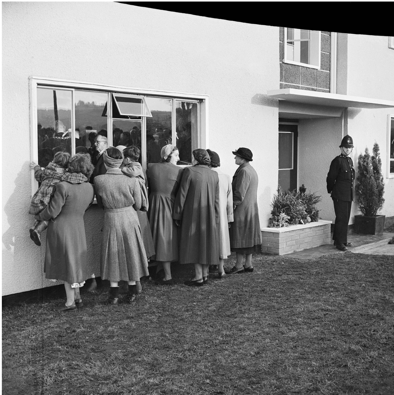
↑ All of the sites are existing 'Easiform' housing constructed after WWII. The walls are uninsulated, load bearing concrete which has presented issues including thermal performance and internal condensation build up.
