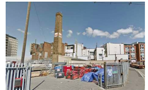
View 3 - Yard and Chimney of No.10 Sugar House Lane
