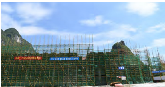
Fengshan County No.2 Senior Middle School Construction Project
