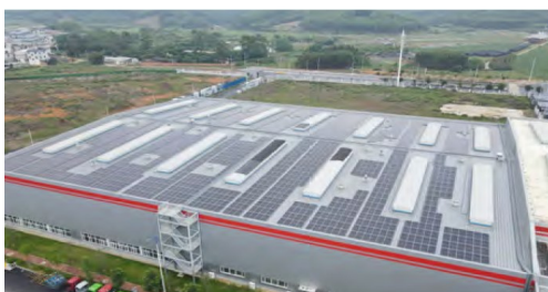
Photovoltaic project at FAW Jiefang Liuzhou Factory
