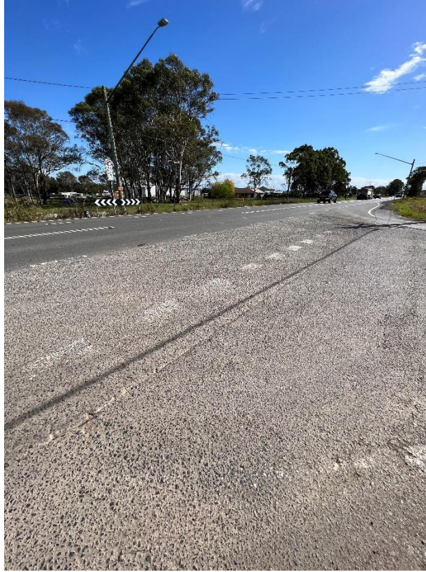
Figure 315 – Crack propagation to the driveway.
