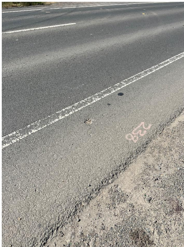
Figure 144 – Crack propagation to the road.
