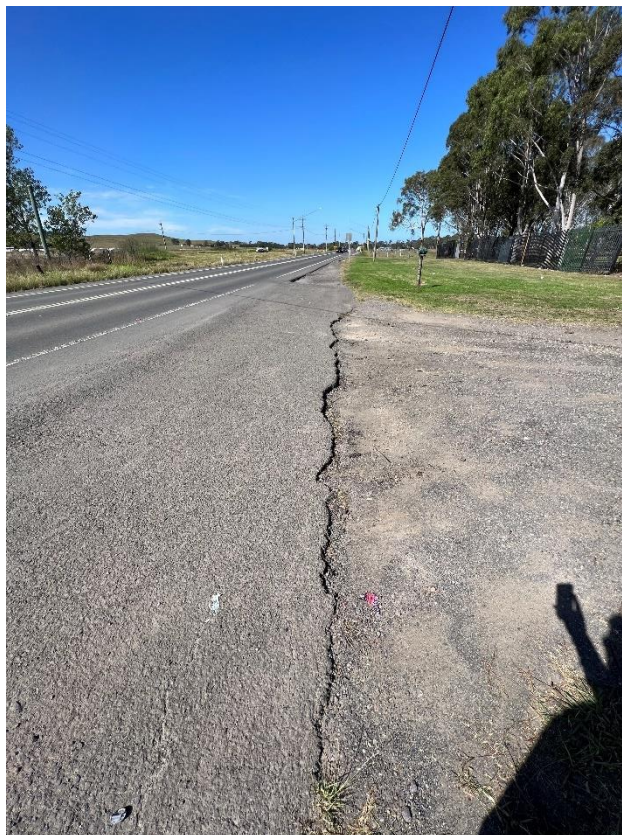
Figure 22 – Crack propagation to the driveway.
