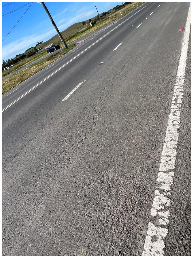
Figure 38 – Crack propagation to the road.
