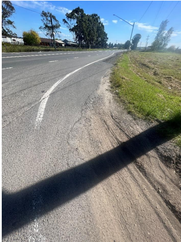
Figure 1 – Crack propagation to the road.
