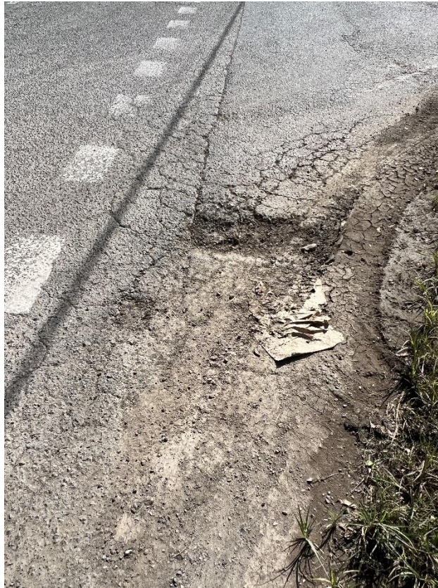
Figure 311 – Crack propagation to the driveway.
