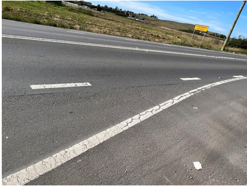
Figure 53 – Crack propagation to the road.
