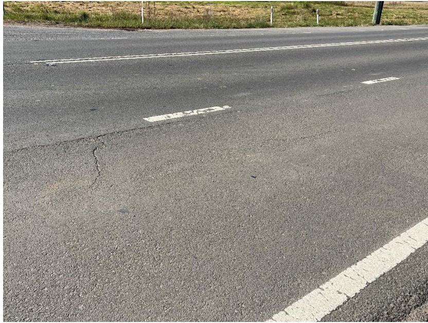
Figure 45 – Crack propagation to the road.
