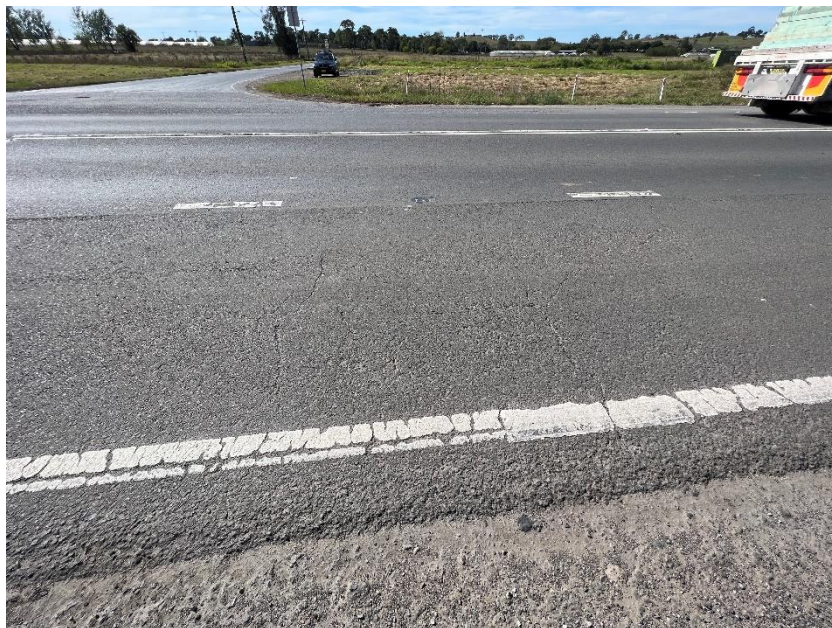
Figure 48 – Crack propagation to the road.
