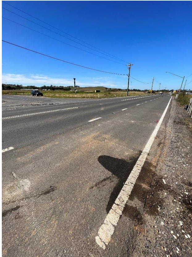
Figure 41 – Crack propagation to the road.
