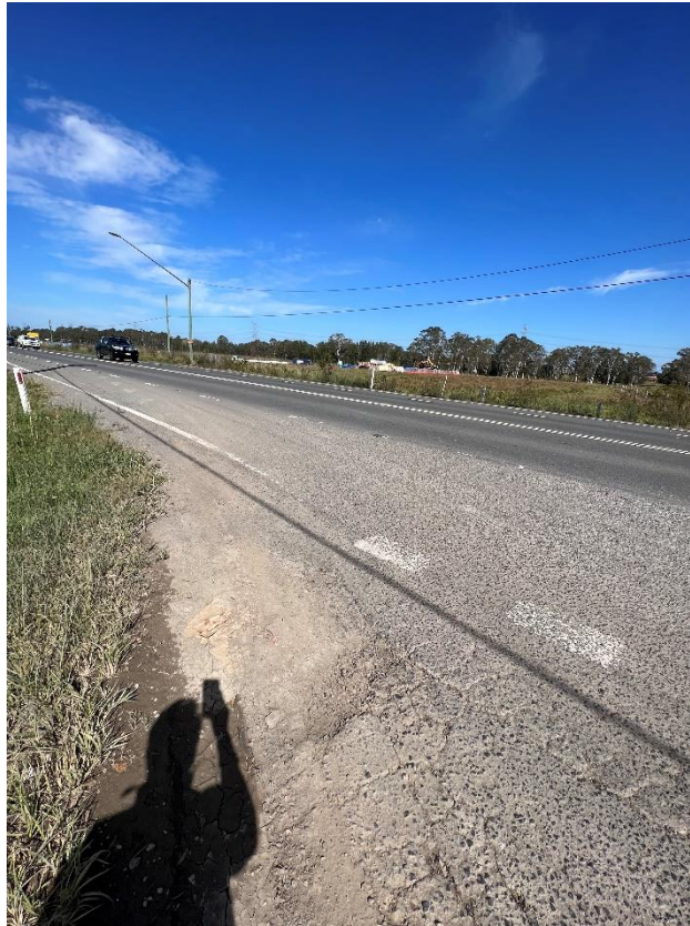
Figure 313 – Crack propagation to the driveway.
