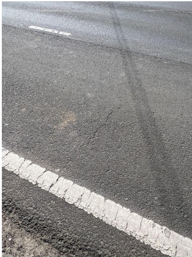
Figure 44 – Crack propagation to the road.
