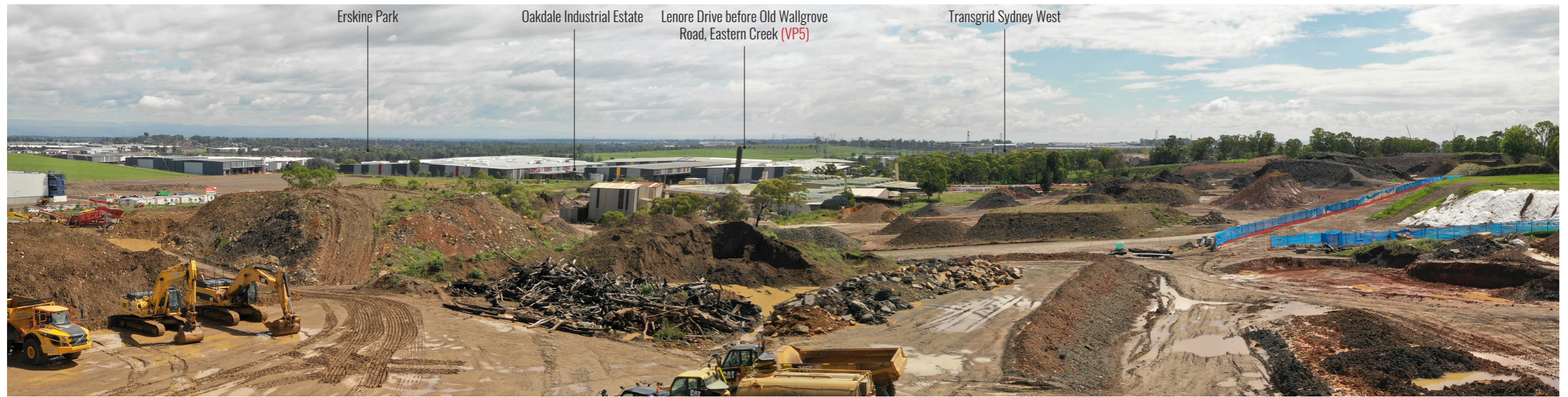
Figure 7: Drone at 104.5m RL Position 2 - Looking North
