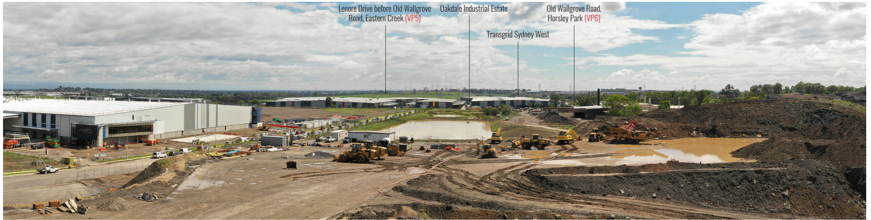
Figure 3: Drone at 98.6m RL Position 1 - Looking North
