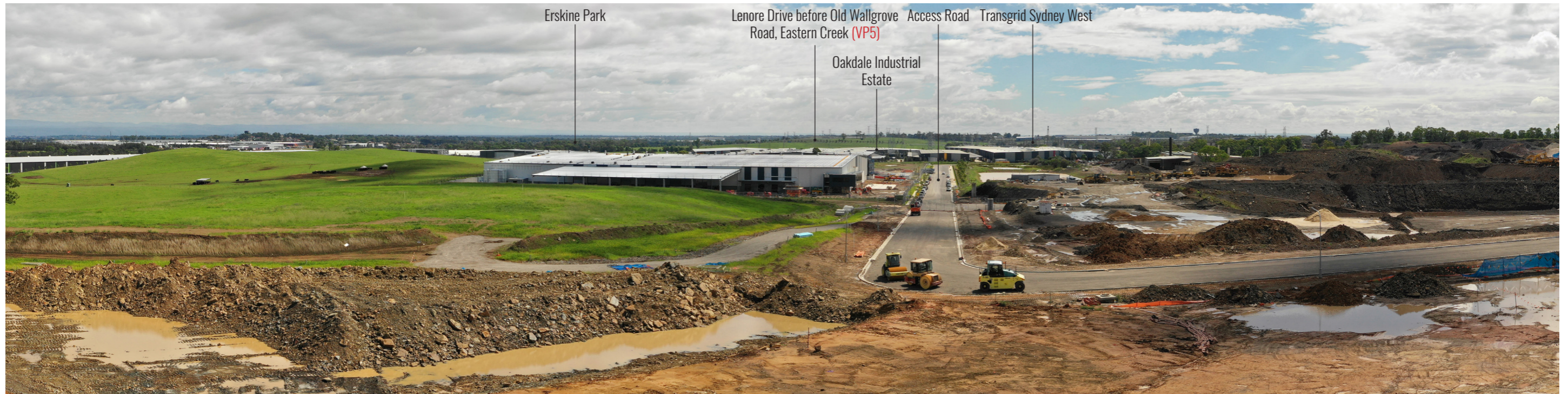
Figure 11: Drone at 101.5m RL Position 3 - Looking North
