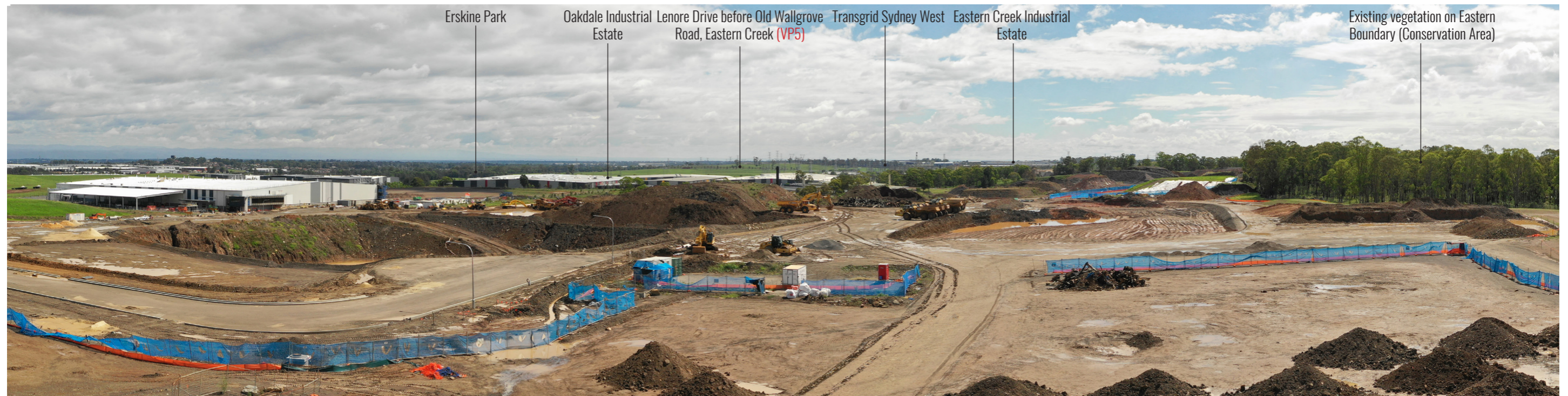
Figure 15: Drone at 104.1m RL Position 4 - Looking North
