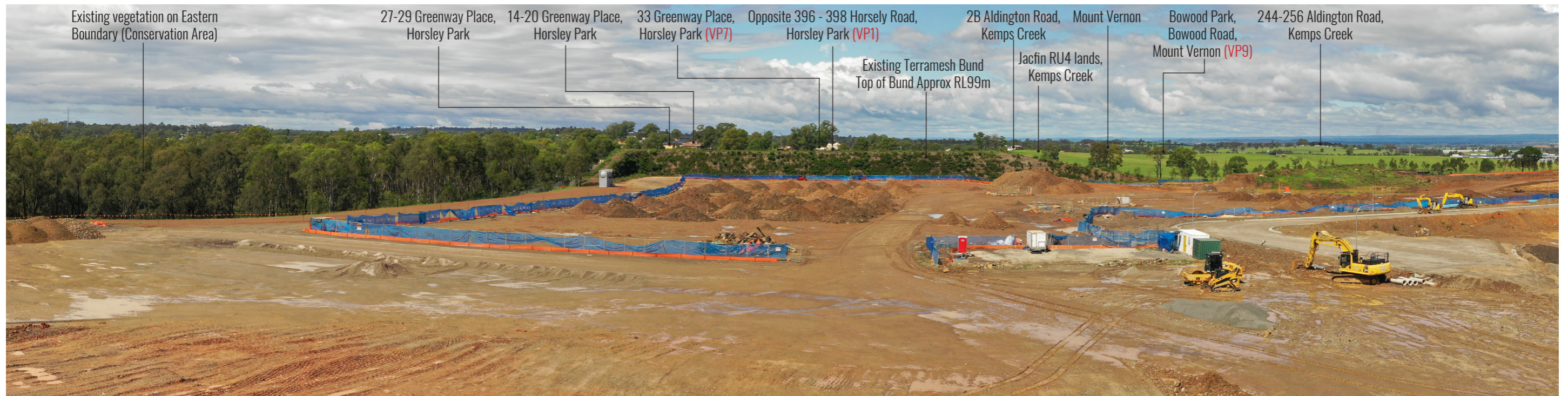
Figure 9: Drone at 104.5m RL Position 2 - Looking South
