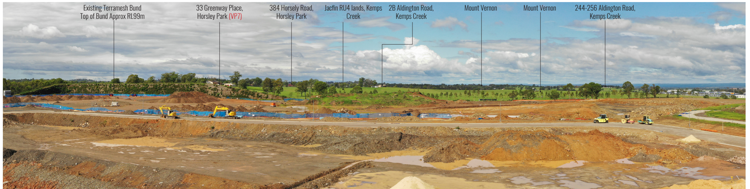
Figure 5: Drone at 98.6m RL Position 1 - Looking South
