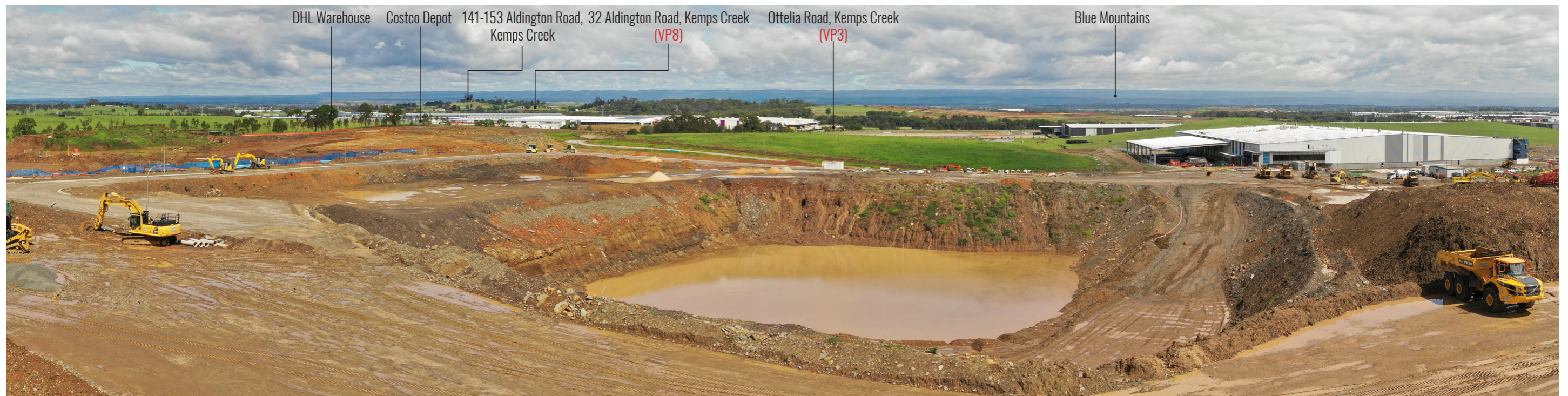
Figure 10: Drone at 104.5m RL Position 2 - Looking West
