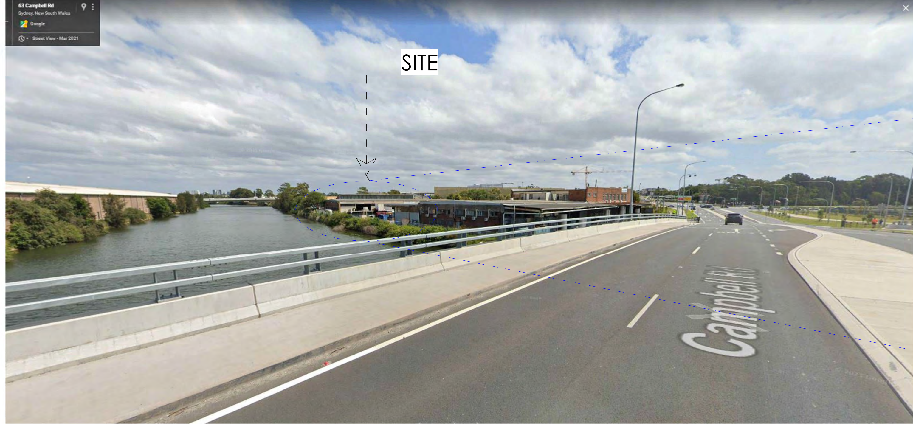
VIEW FROM NEW CAMPBELL BRIDGE TO SITE
