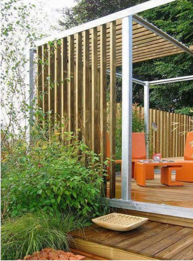
Exposed timber batton pergola
