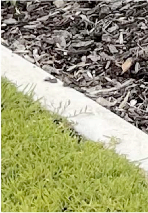
Flush concrete kerbs
