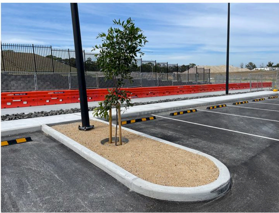
Tree planted & staked, steel rings installed ready for with aggregate
