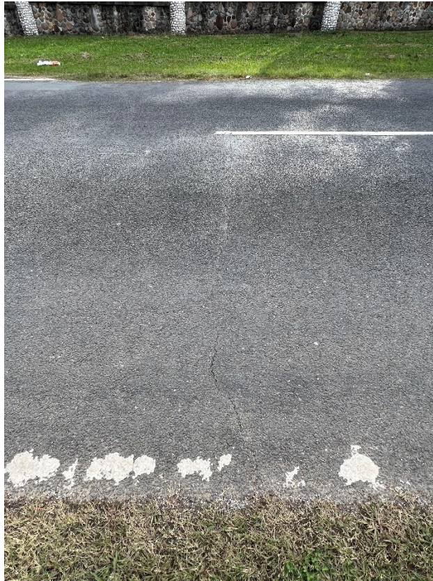
Figure 91 – Crack propagation to the road.
