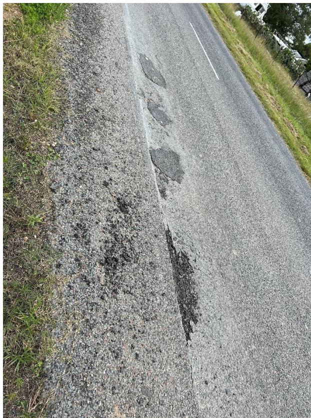
Figure 62 – Crack propagation to the road.
