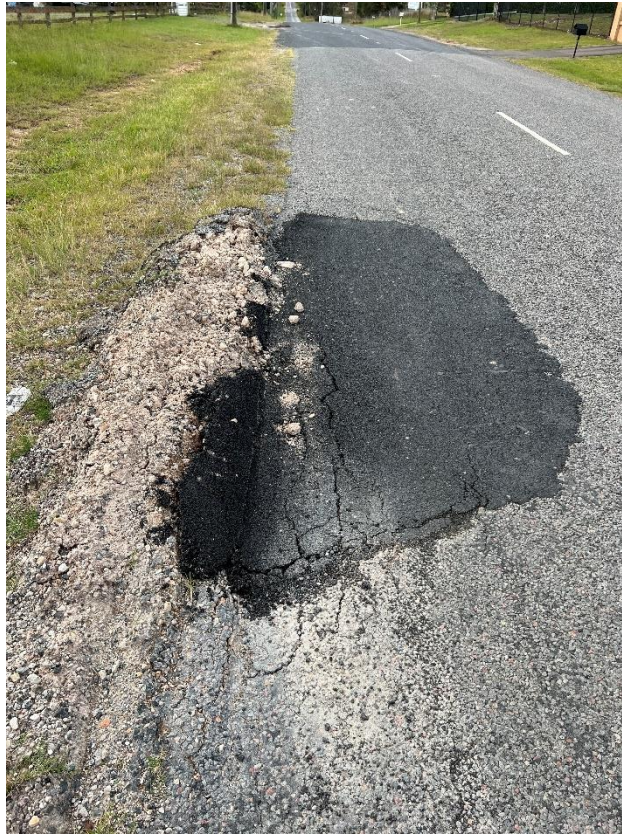
Figure 33 – Crack propagation to the road.
