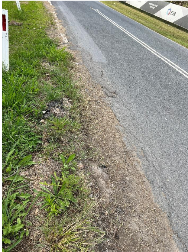
Figure 3 – Crack propagation to the road.
