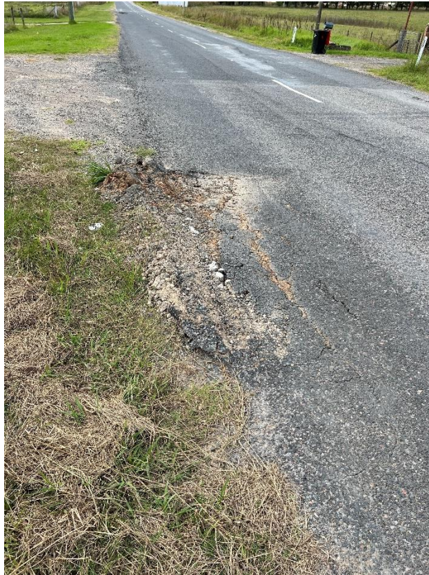
Figure 49 – Crack propagation to the road.
