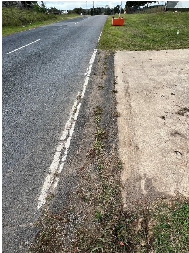
Figure 25 – Crack propagation to the road/driveway.
