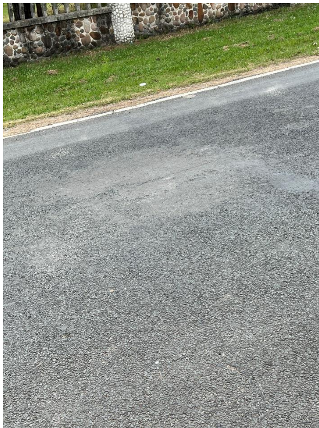
Figure 92 – Crack propagation to the road.
