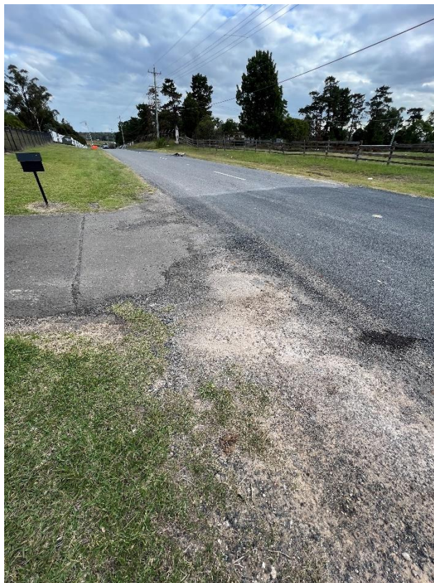
Figure 76 – Crack propagation to the driveway.
