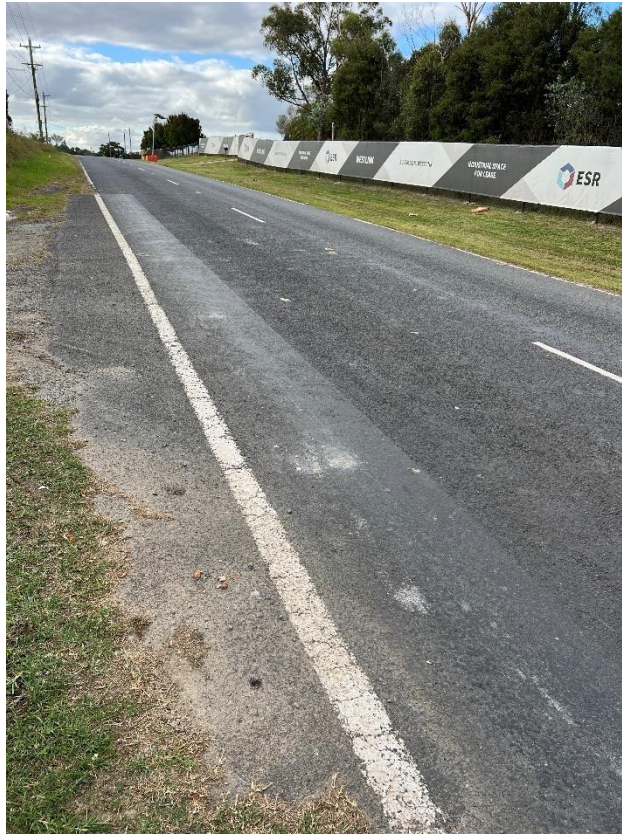
Figure 19 – Crack propagation to the road.
