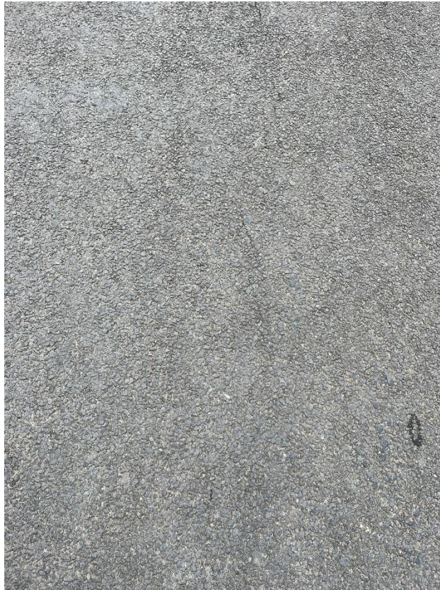
Figure 15 – Crack propagation to the road.
