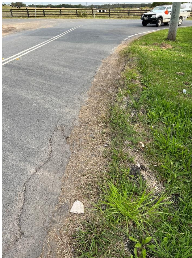
Figure 4 – Crack propagation to the road.
