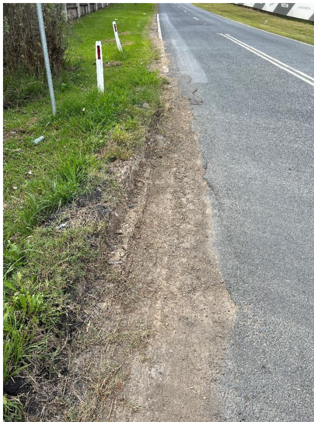
Figure 2 – Crack propagation to the road.
