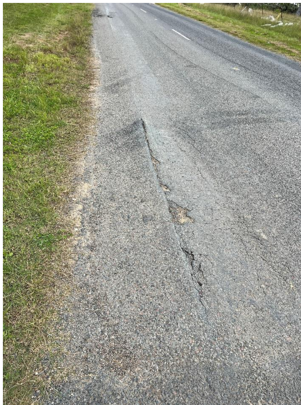
Figure 58 – Crack propagation to the road.
