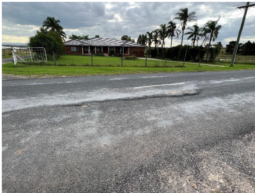
Figure 54 – Crack propagation to the road.
