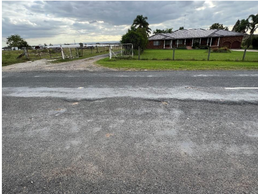
Figure 55 – Crack propagation to the road.
