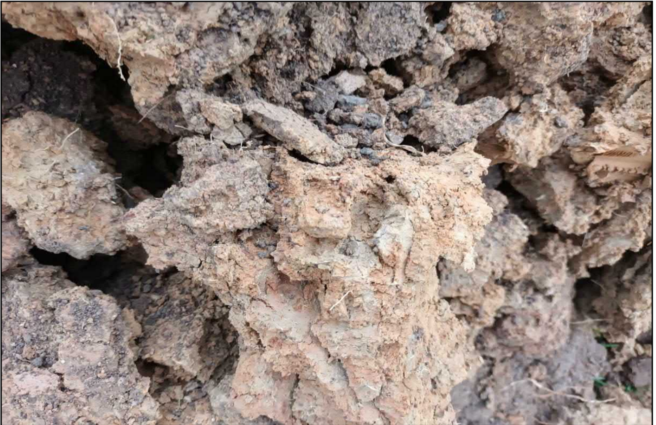
Photograph 17. Encountered natural clay materials in TP235. Date: 27.03.2023.
