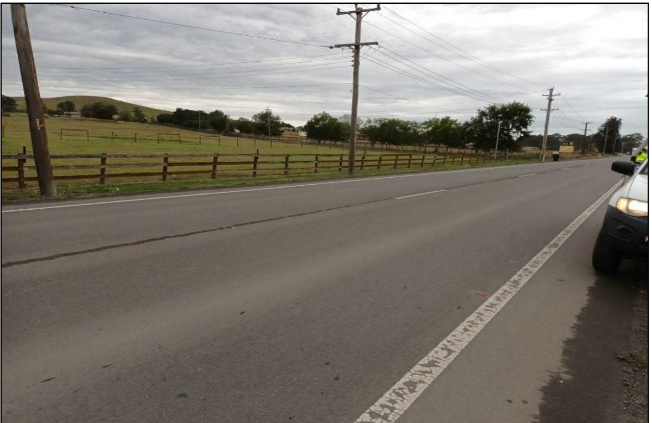
Photograph 6. South-eastern facing view of site from TP234. Date: 27.03.2023.
