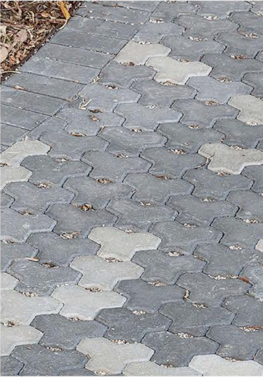
Permeable paving (Ecohitrex pavers)
