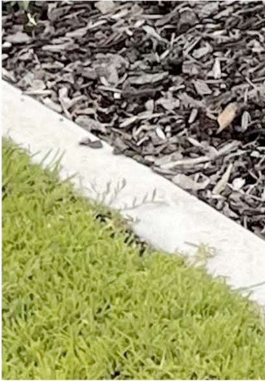
Flush concrete kerbs
