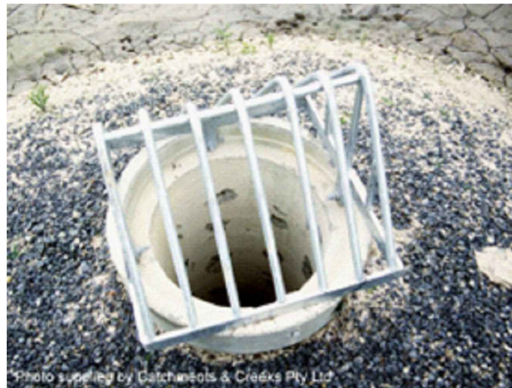
RISER PIPE WITH AGGREGATE FILTER
