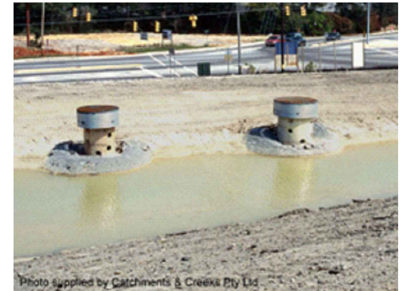
RISER PIPES UNDER CONSTRUCTION
