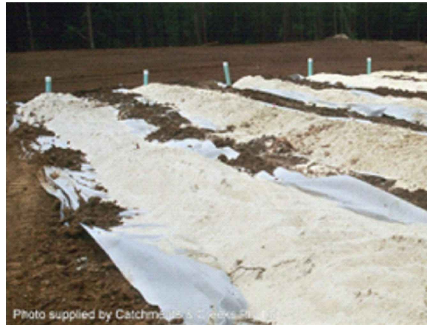
SAND FILTER OUTLET
