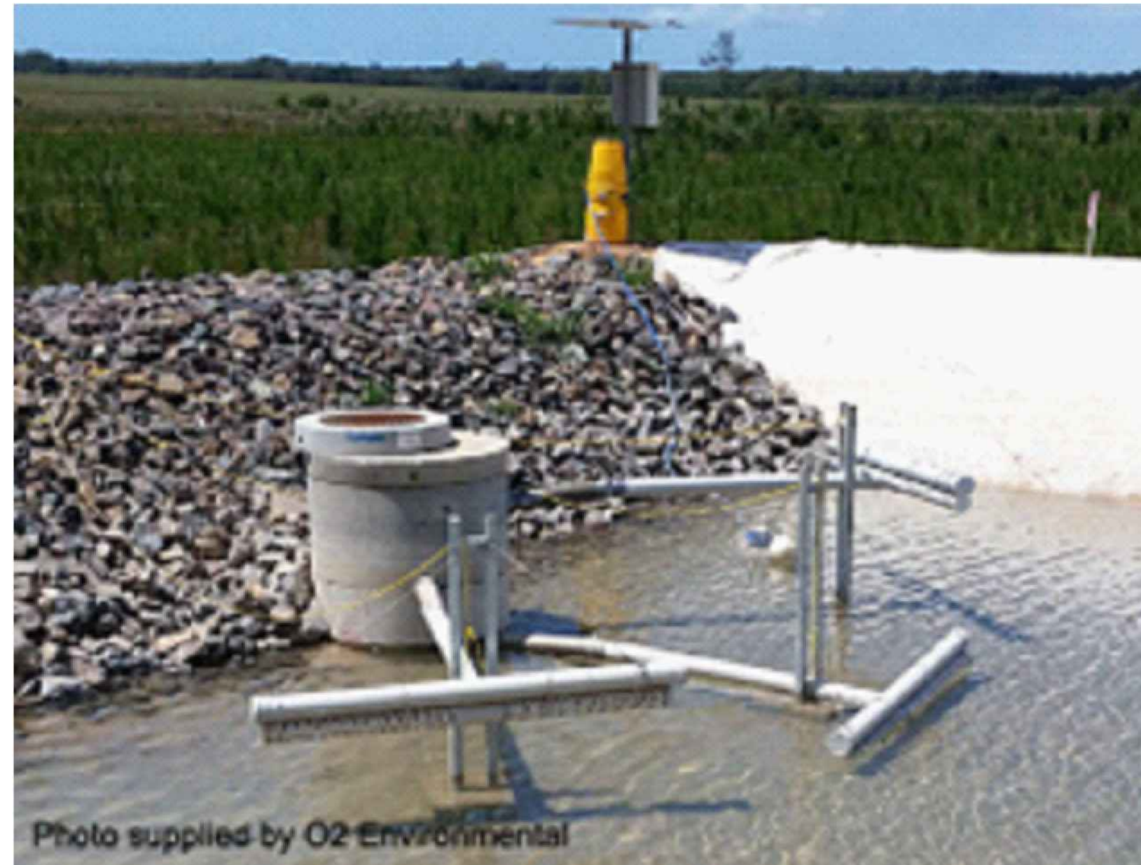
TYPE A DECANT AT LOW WATER LEVEL
