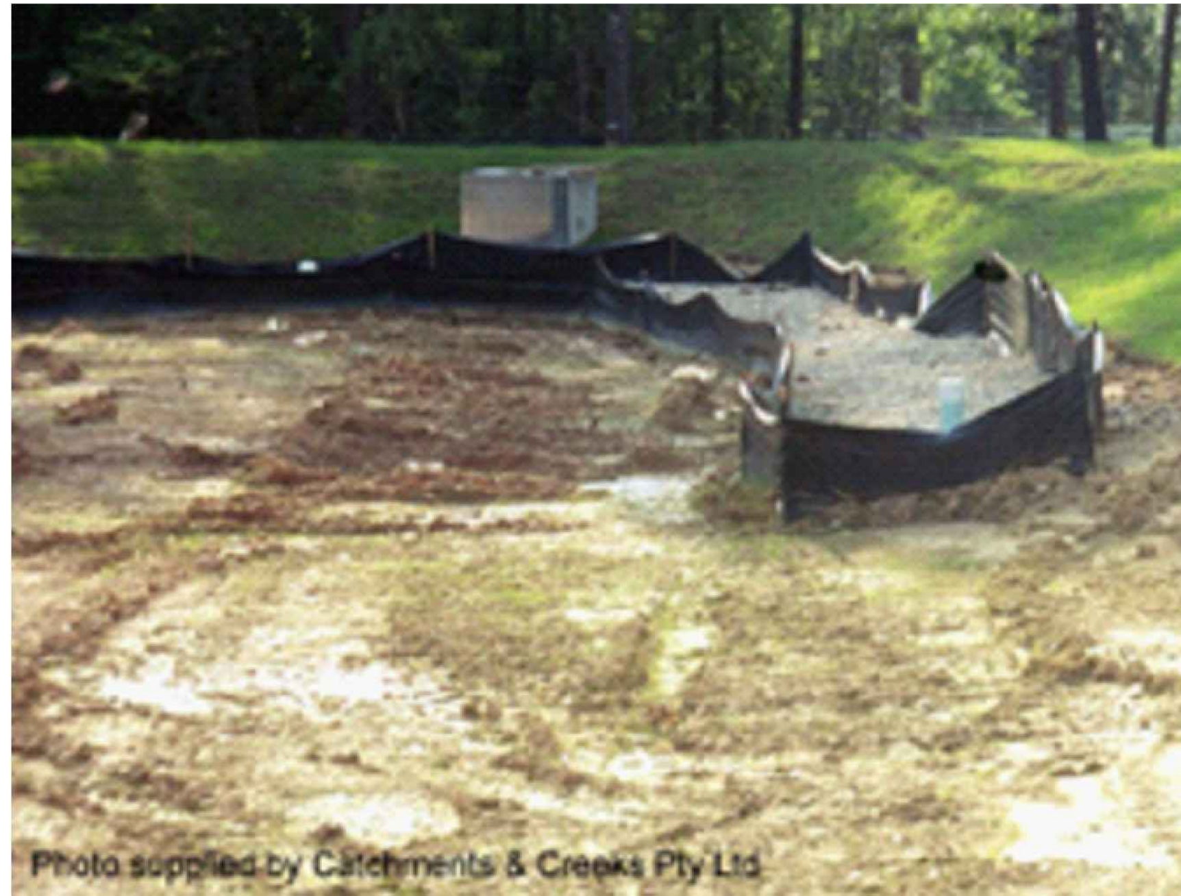
SAND FILTER OUTLET
