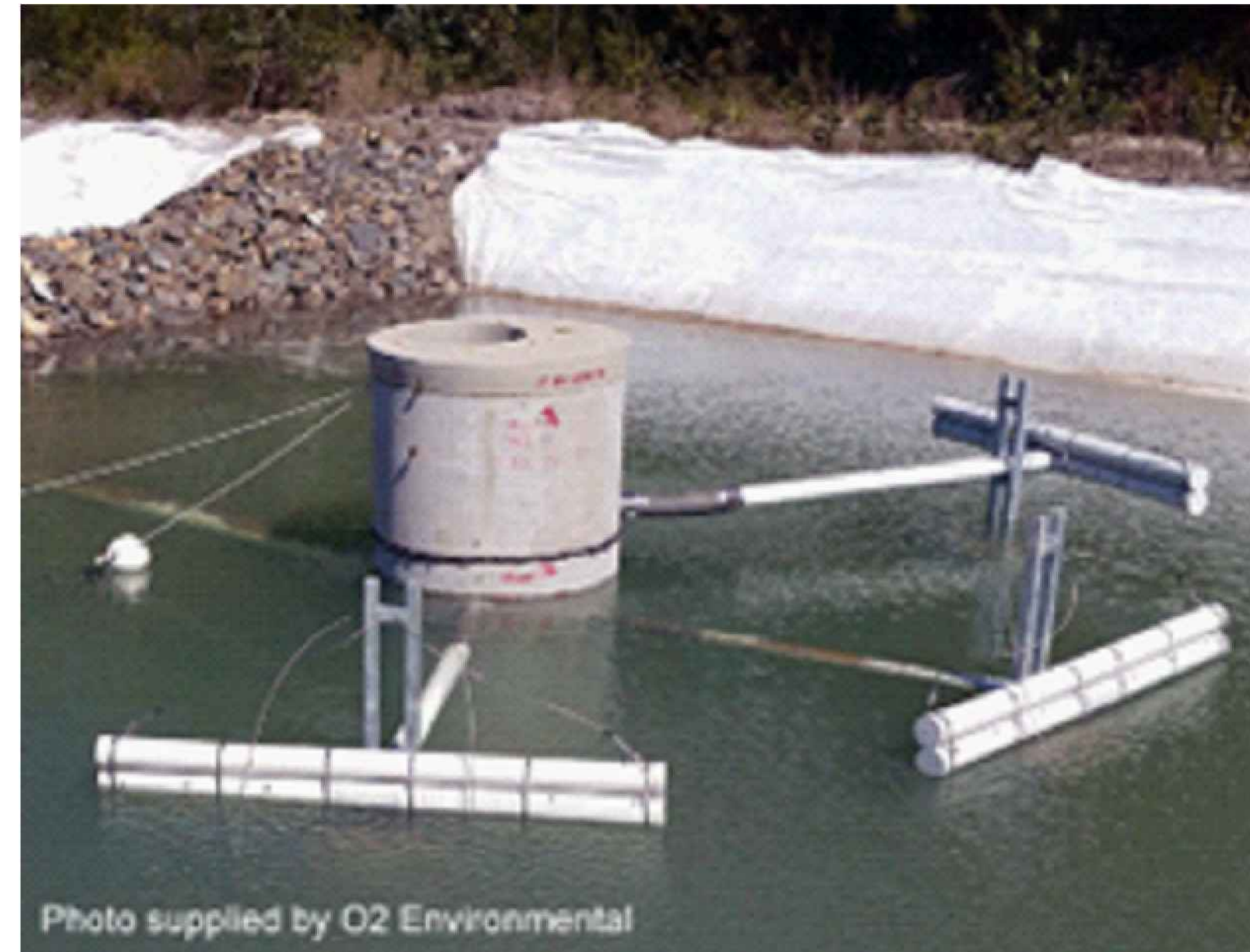
FLOATING ARM DECANT SYSTEM
