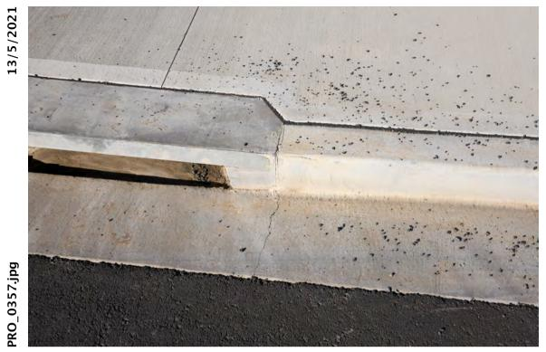
Johnston Crescent. Area adjacent to 6 Johnston Crescent (to the north of the site). Heading south along the eastern side of the Crescent. Area between light pole ID 957686 and 957687. Storm water drain. Cracked gutter.
