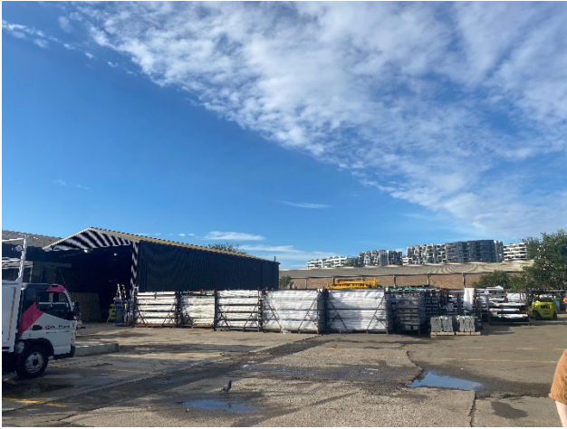
Picture 3 Existing structures and hardstand at 28 Burrows Road
