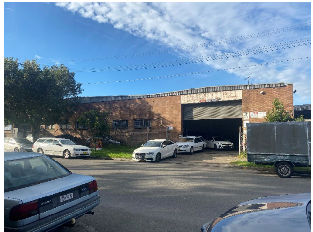
Picture 8 Industrial buildings at 30 Burrows Road
