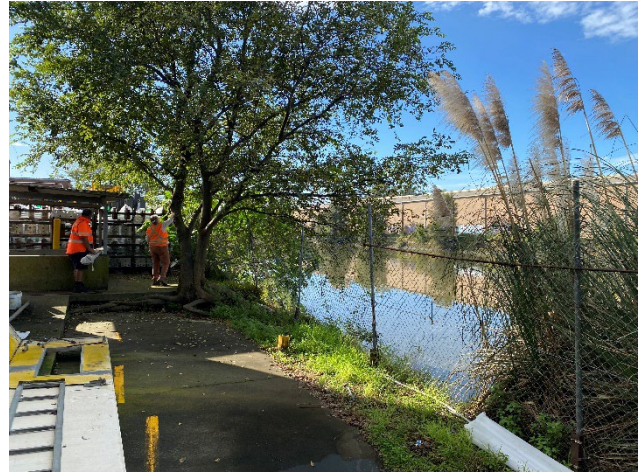
Picture 4 Frontage to Alexandra Canal
