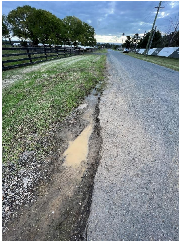
Figure 37 – Crack propagation to the road.
