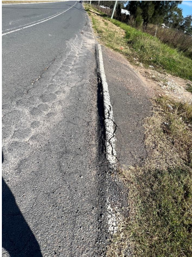
Figure 103 – Crack propagation to the road/driveway.
