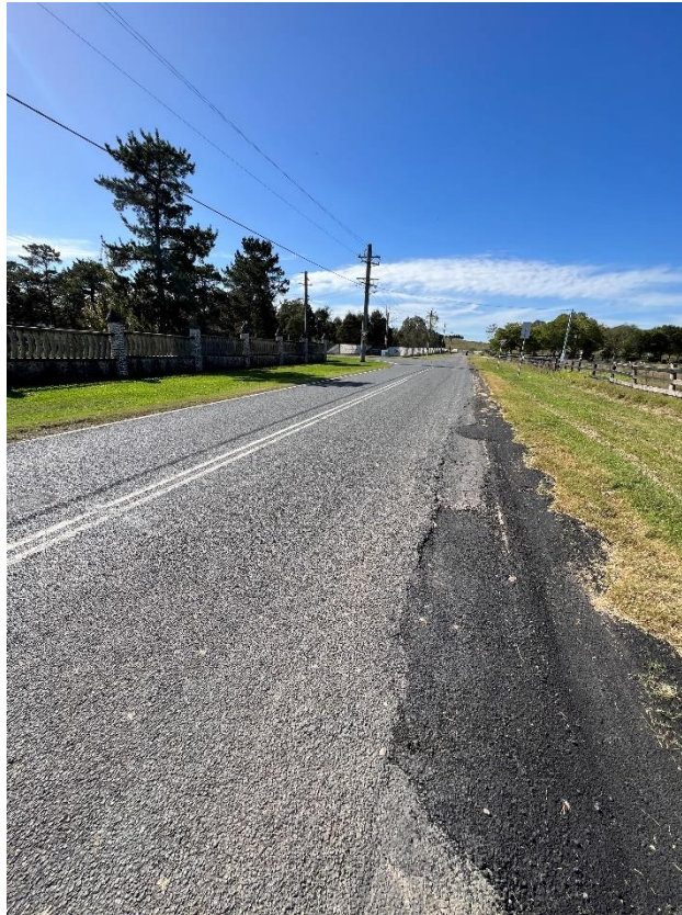
Figure 201 – Crack propagation to the road.
