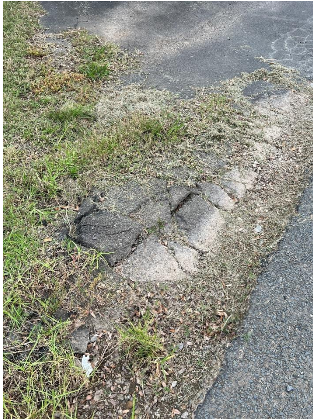
Figure 43 – Crack propagation to the driveway.
