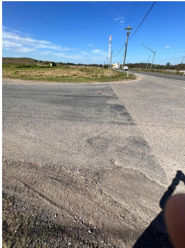
Figure 126 – Crack propagation to the road.
