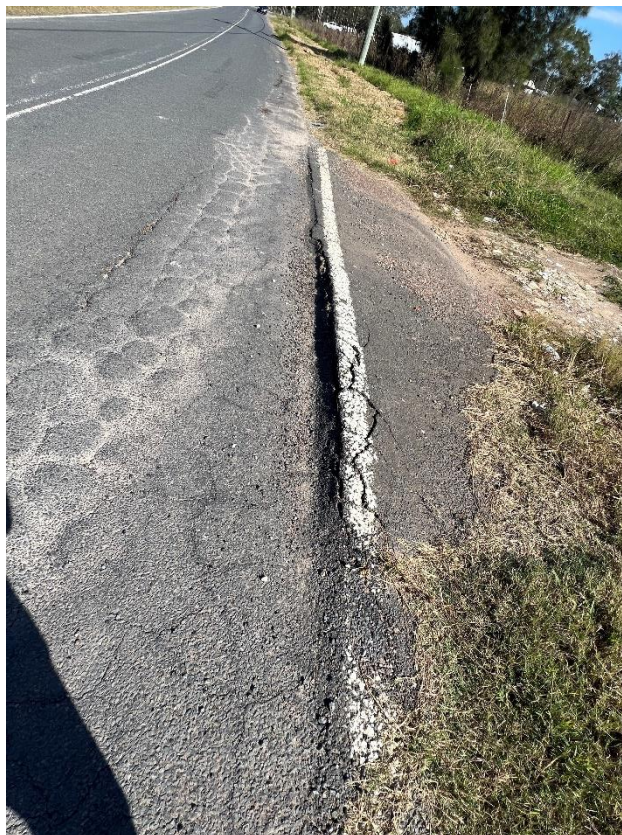
Figure 104 – Crack propagation to the road/driveway.
