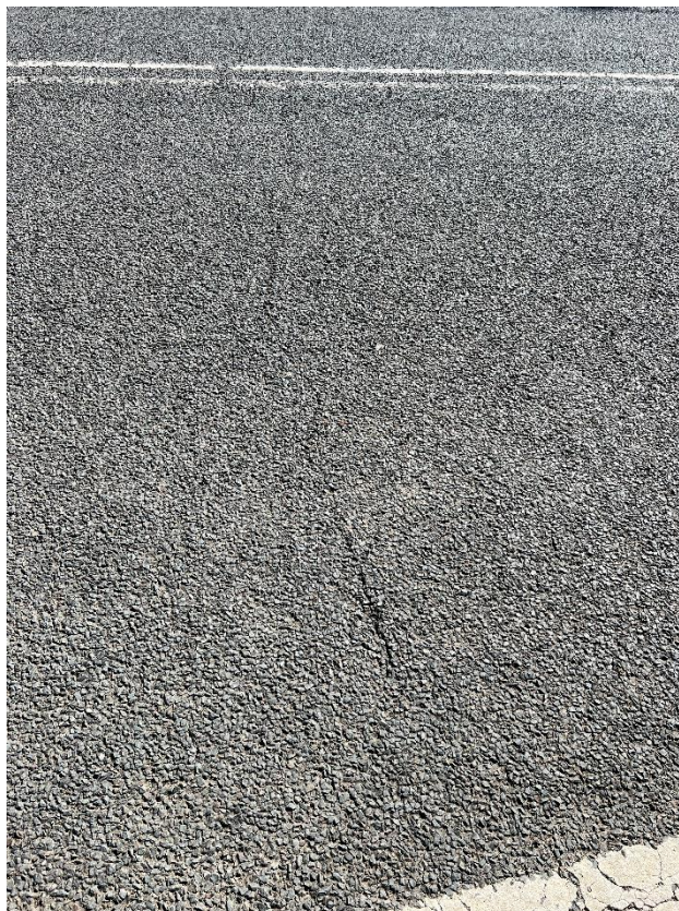
Figure 156 – Crack propagation to the road.
