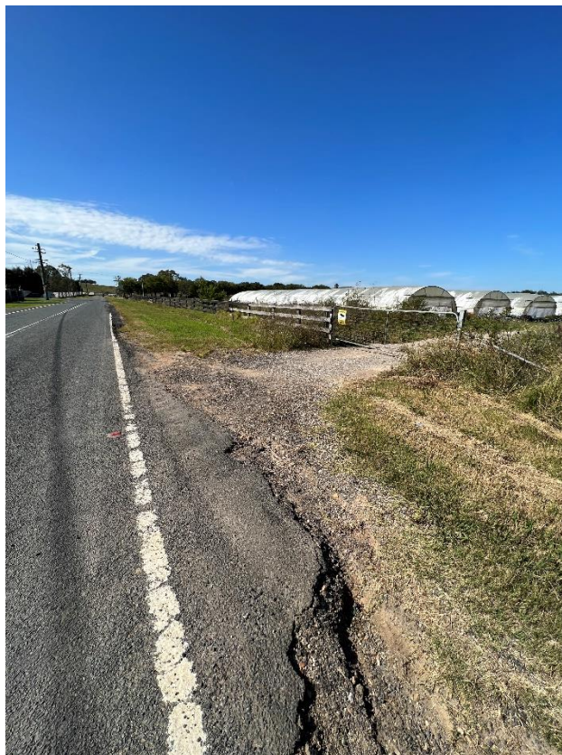
Figure 194 – Crack propagation to the road.
