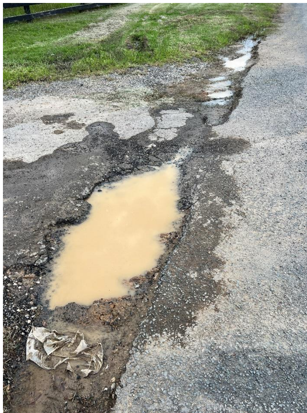
Figure 34 – Crack propagation to the driveway.
