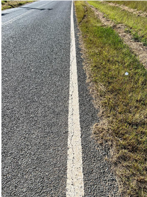
Figure 155 – Crack propagation to the road.
