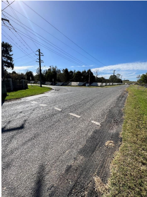
Figure 209 – Crack propagation to the road.
