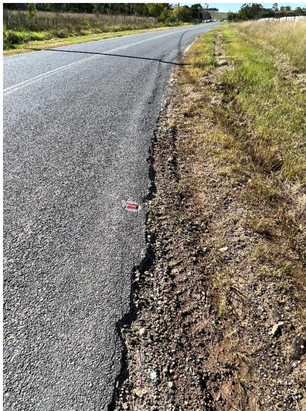
Figure 164 – Crack propagation to the road.
