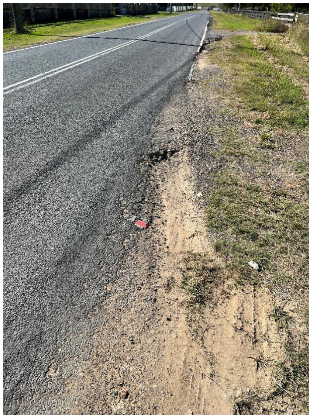
Figure 188 – Crack propagation to the road.
