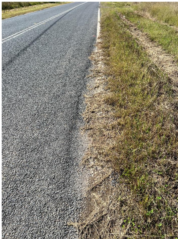
Figure 170 – Crack propagation to the road.
