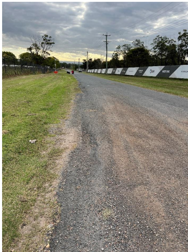
Figure 24 – Crack propagation to the road.
