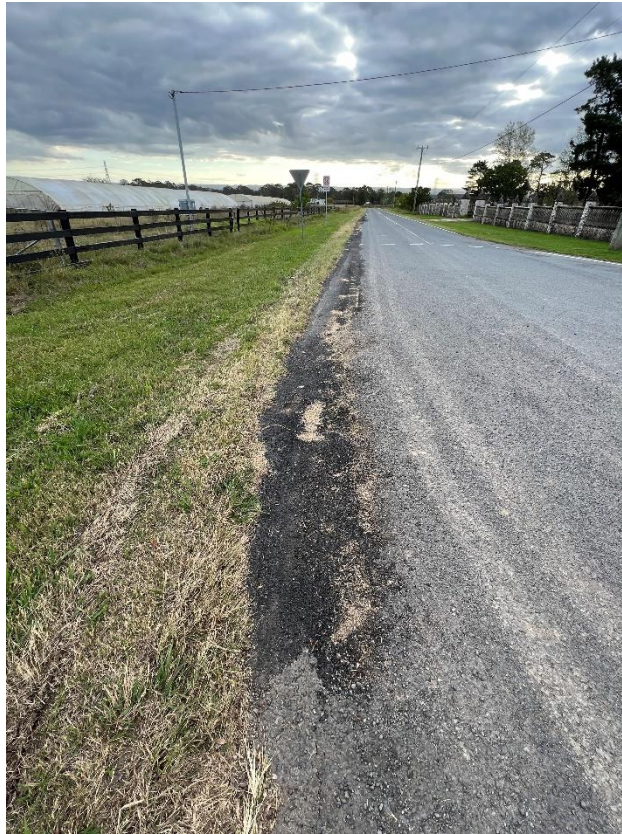
Figure 51 – Crack propagation to the road.
