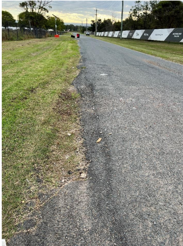
Figure 25 – Crack propagation to the road.
