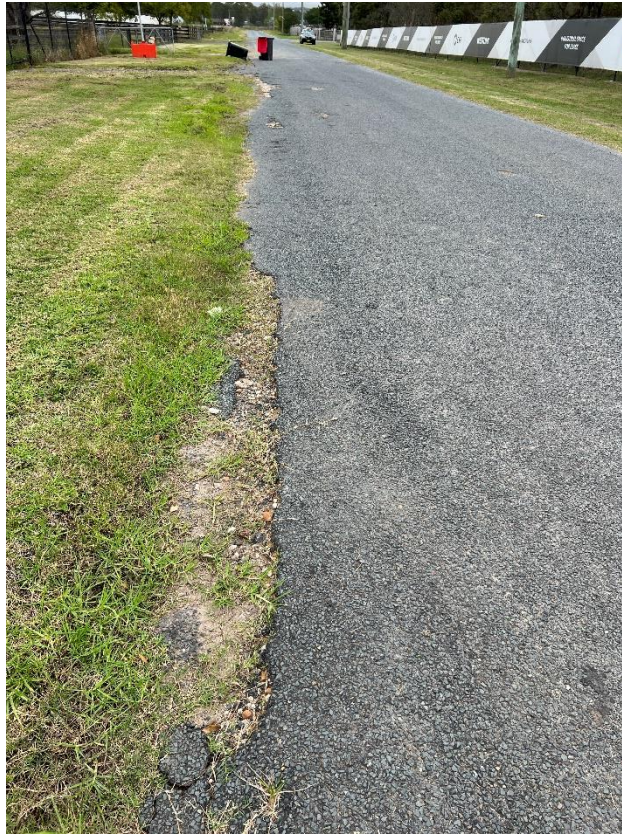
Figure 27 – Crack propagation to the road.
