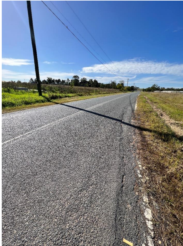
Figure 167 – Crack propagation to the road.
