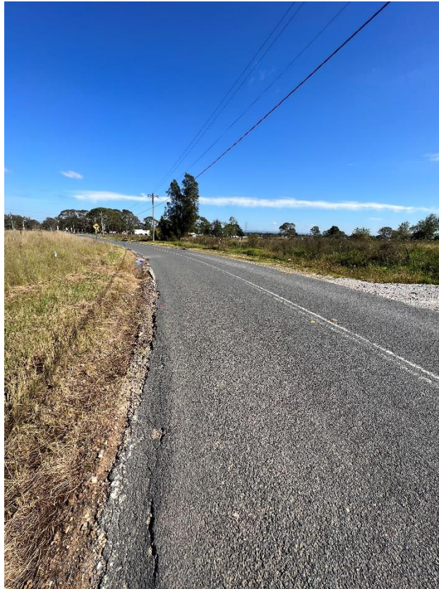
Figure 165 – Crack propagation to the road.
