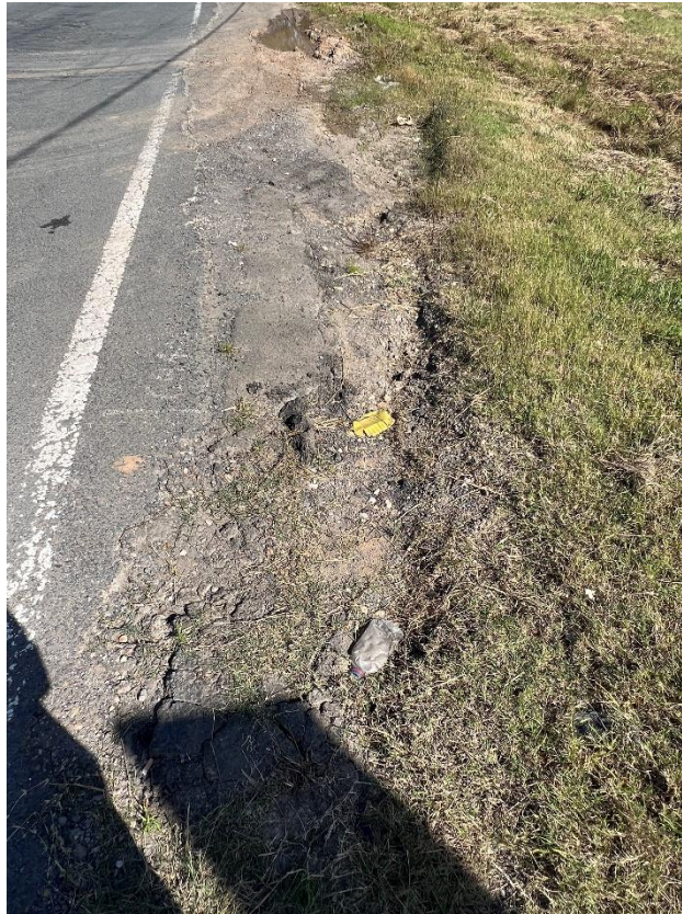
Figure 117 – Crack propagation to the road.
