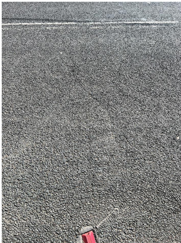
Figure 158 – Crack propagation to the road.
