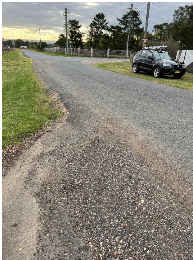
Figure 46 – Crack propagation to the driveway.
