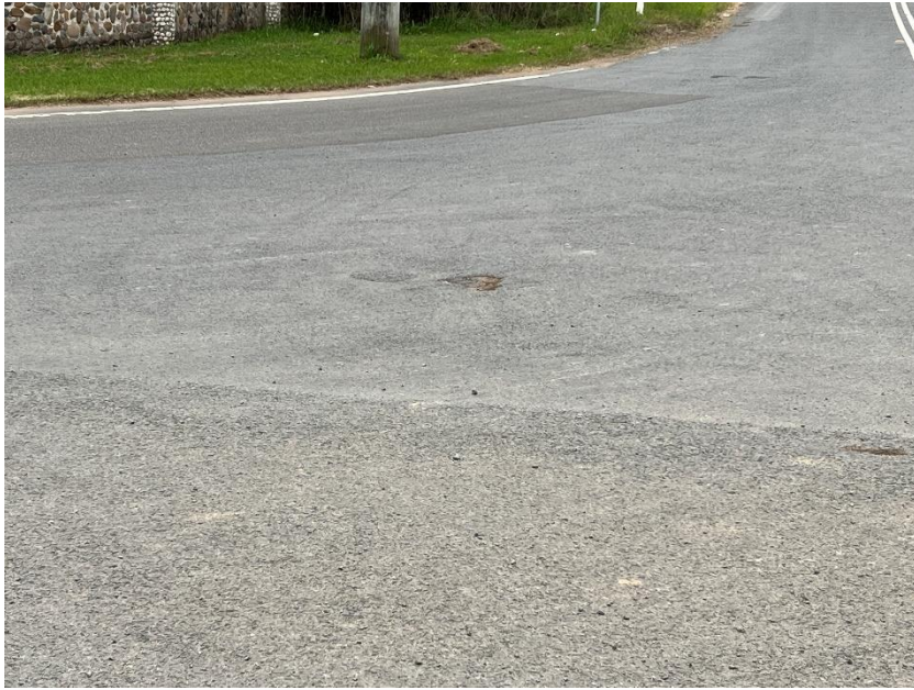
Figure 53 – Crack propagation to the road.
