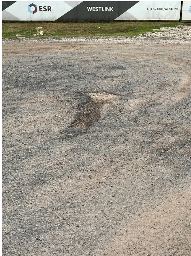
Figure 23 – Crack propagation to the road.
