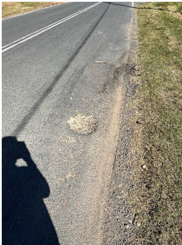
Figure 114 – Crack propagation to the road.
