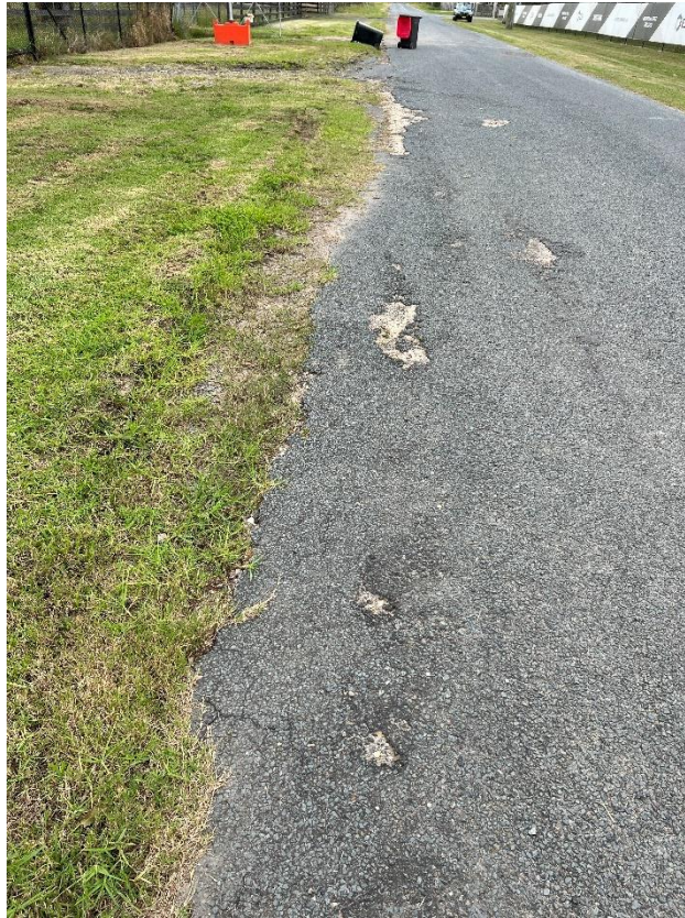
Figure 29 – Crack propagation to the road.
