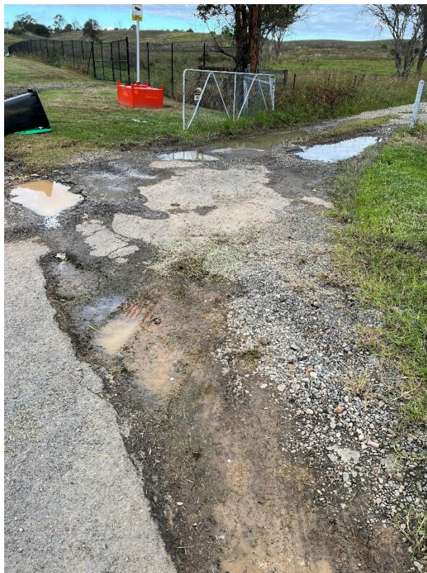
Figure 36 – Crack propagation to the driveway.
