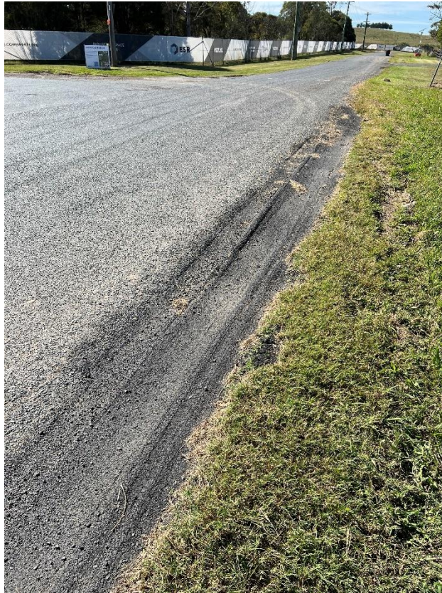
Figure 211 – Crack propagation to the road.
