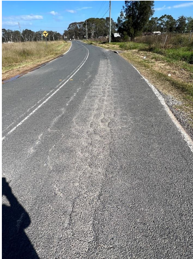
Figure 99 – Crack propagation to the road.
