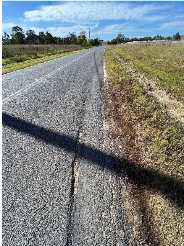
Figure 169 – Crack propagation to the road.
