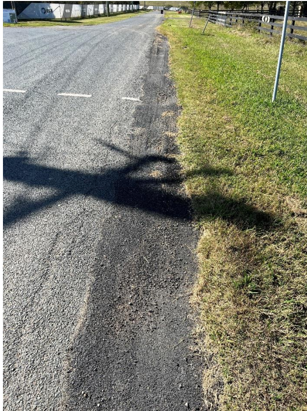
Figure 207 – Crack propagation to the road.
