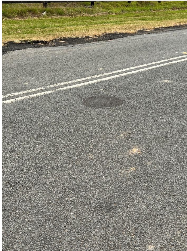
Figure 63 – Crack propagation to the road.
