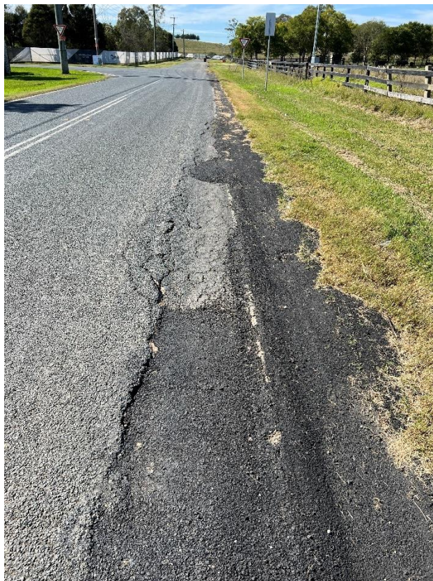
Figure 202 – Crack propagation to the road.
