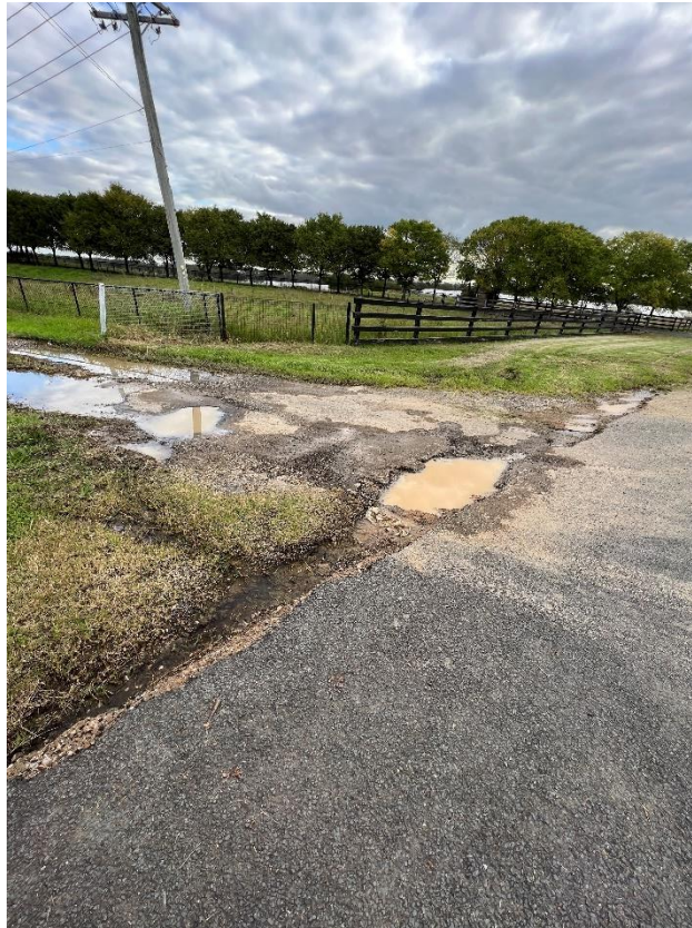
Figure 33 – Crack propagation to the driveway.
