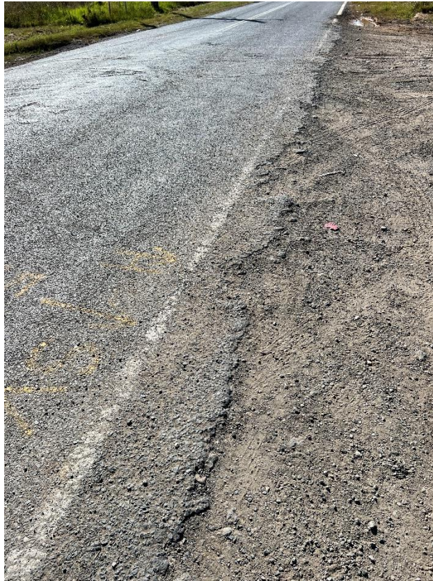
Figure 141 – Crack propagation to the road.
