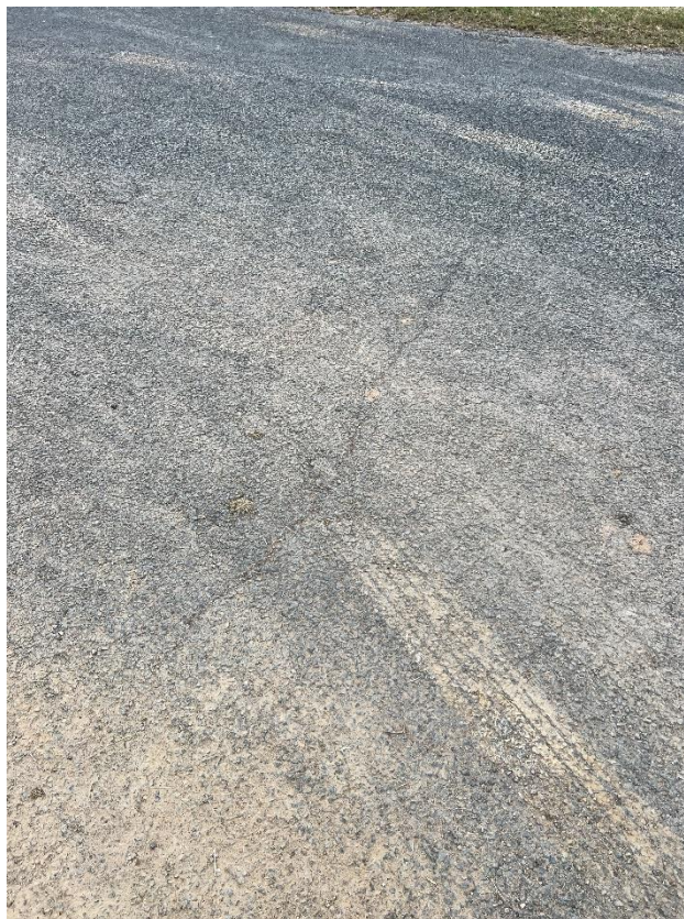
Figure 38 – Crack propagation to the road.
