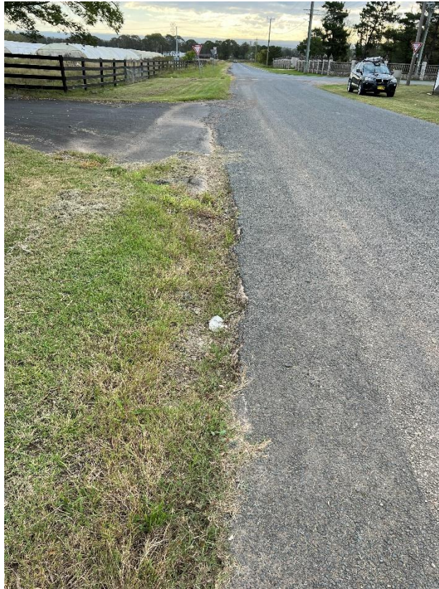
Figure 41 – Crack propagation to the road.
