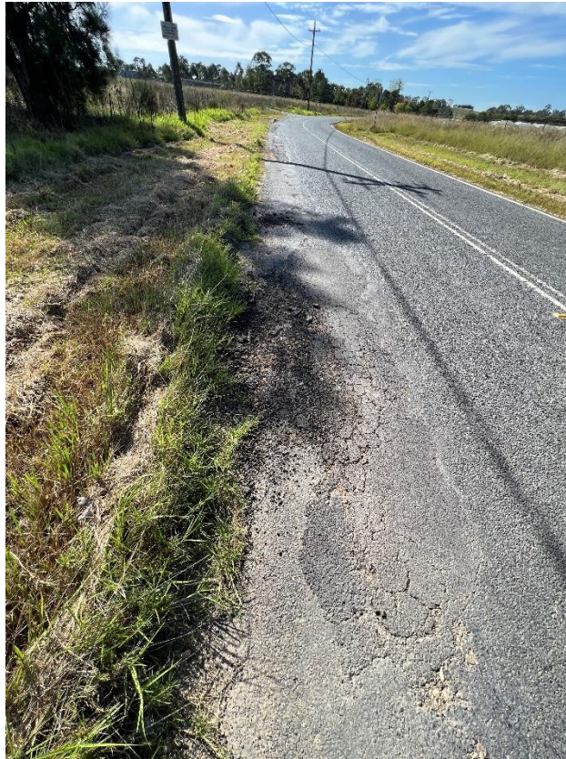
Figure 111 – Crack propagation to the road.
