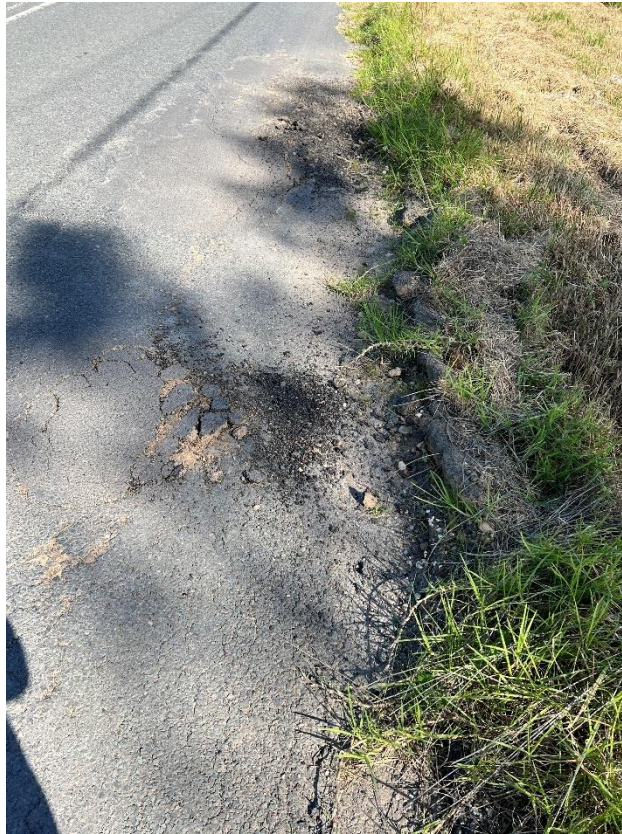
Figure 109 – Crack propagation to the road.
