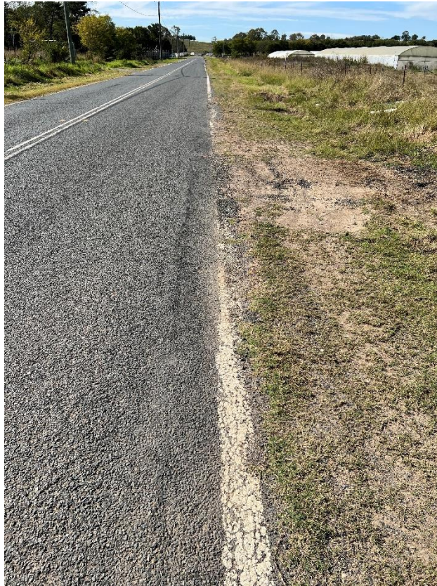
Figure 175 – Crack propagation to the road.
