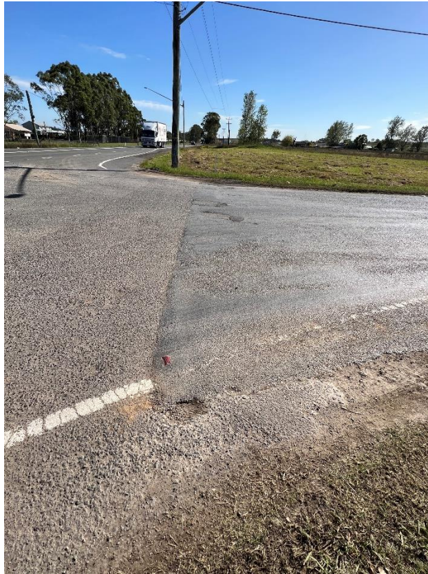
Figure 133 – Crack propagation to the road.
