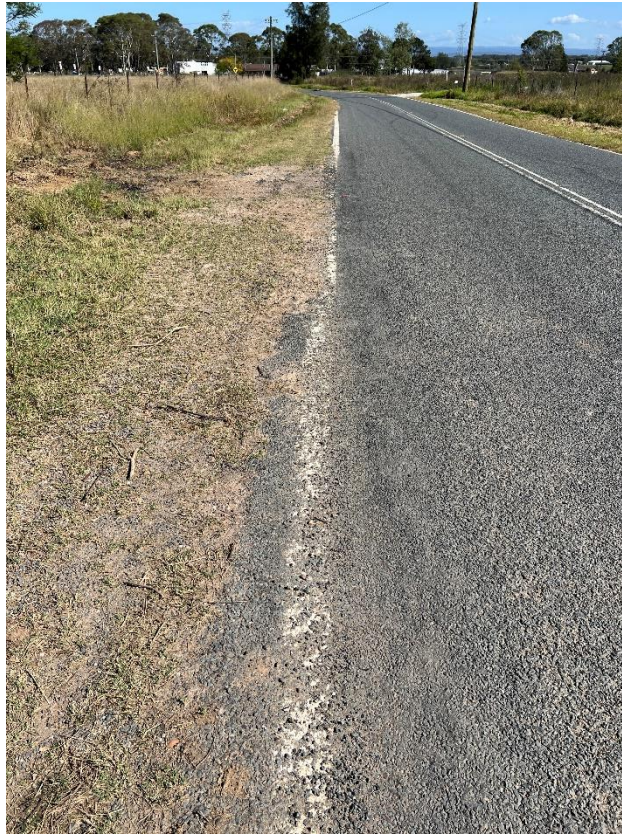
Figure 177 – Crack propagation to the road.
