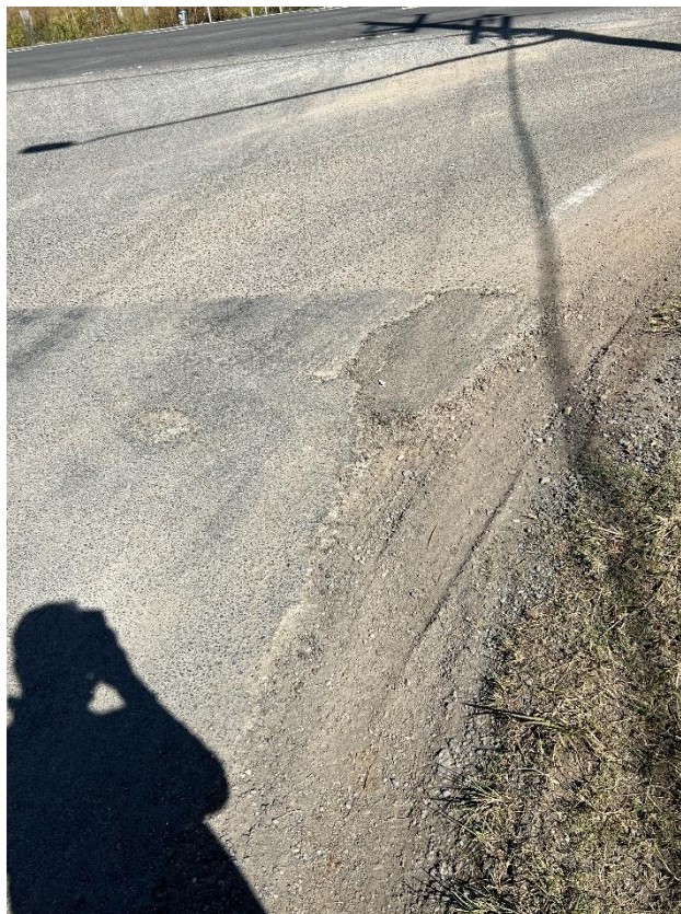
Figure 124 – Crack propagation to the road.
