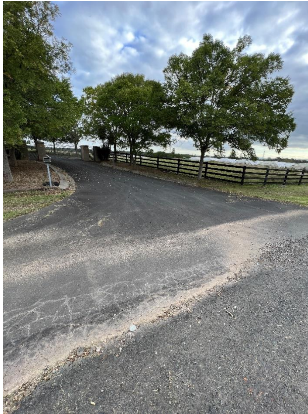
Figure 45 – Crack propagation to the driveway.
