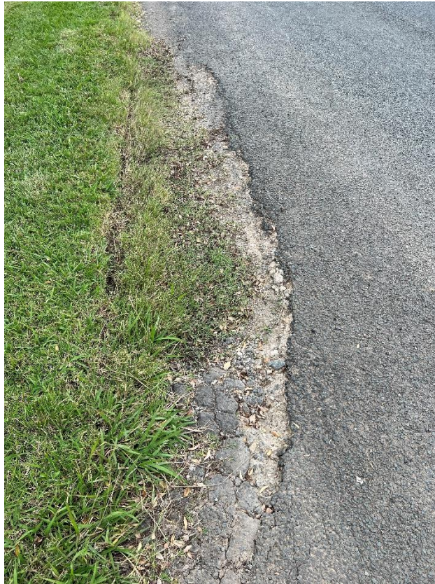
Figure 47 – Crack propagation to the driveway.
