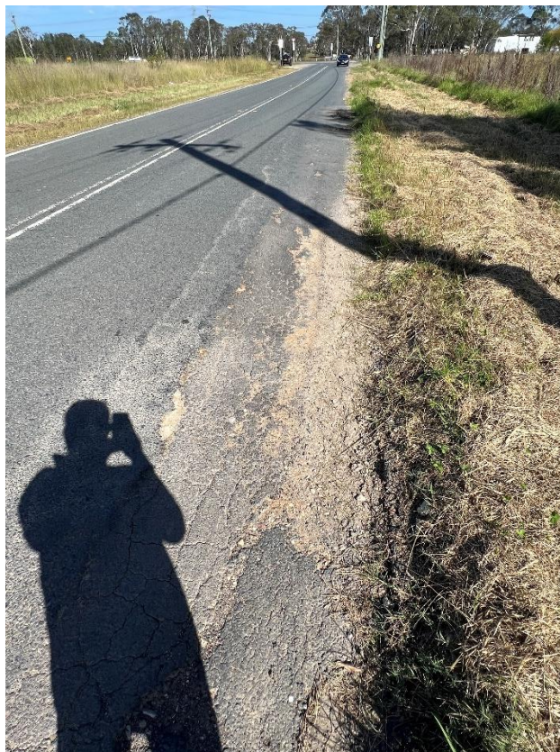
Figure 108 – Crack propagation to the road.
