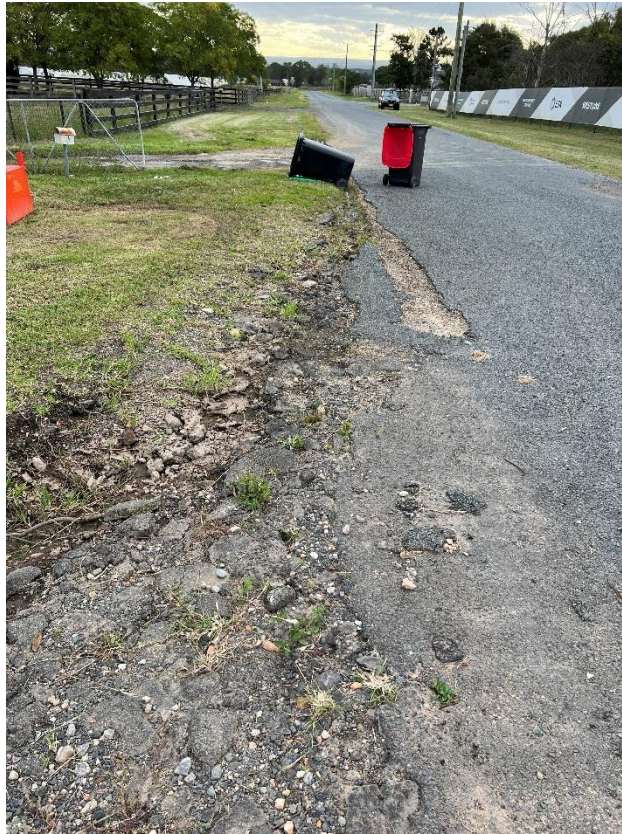
Figure 31 – Crack propagation to the road.
