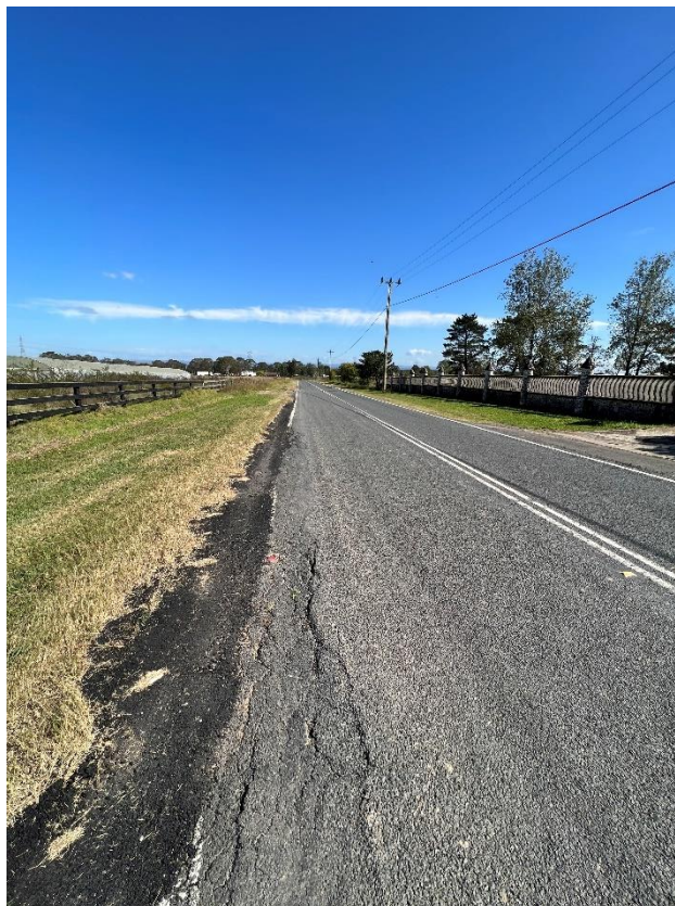
Figure 200 – Crack propagation to the road.
