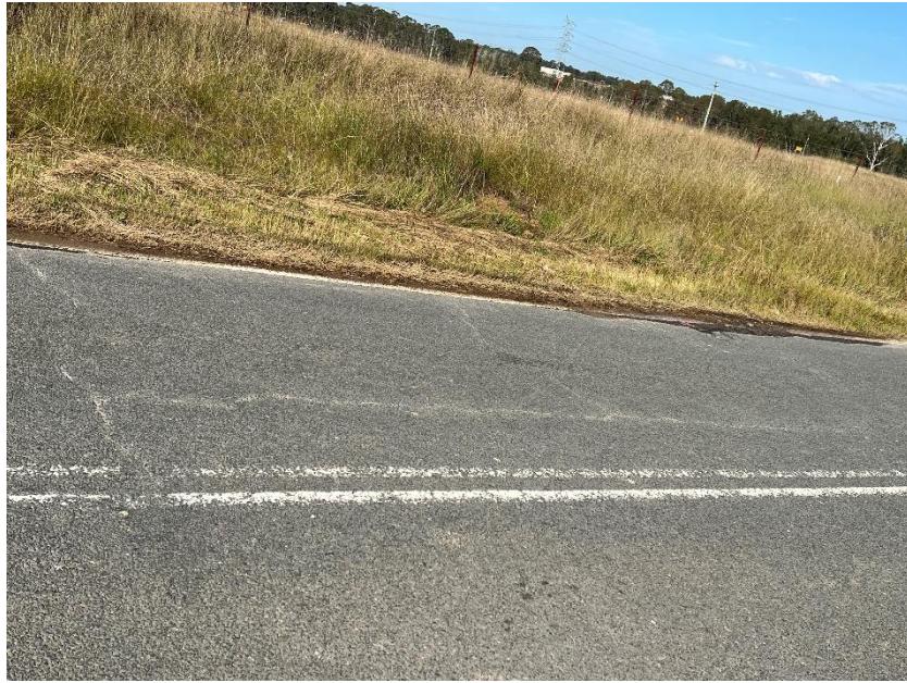
Figure 101 – Crack propagation to the road.
