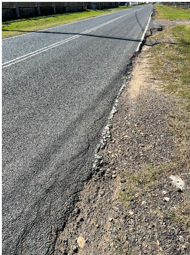
Figure 190 – Crack propagation to the road.
