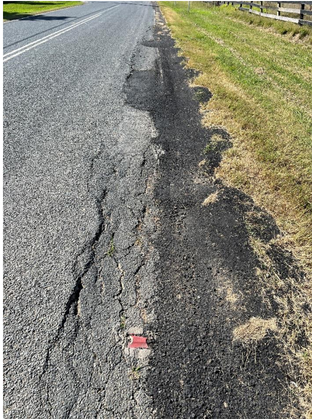
Figure 199 – Crack propagation to the road.
