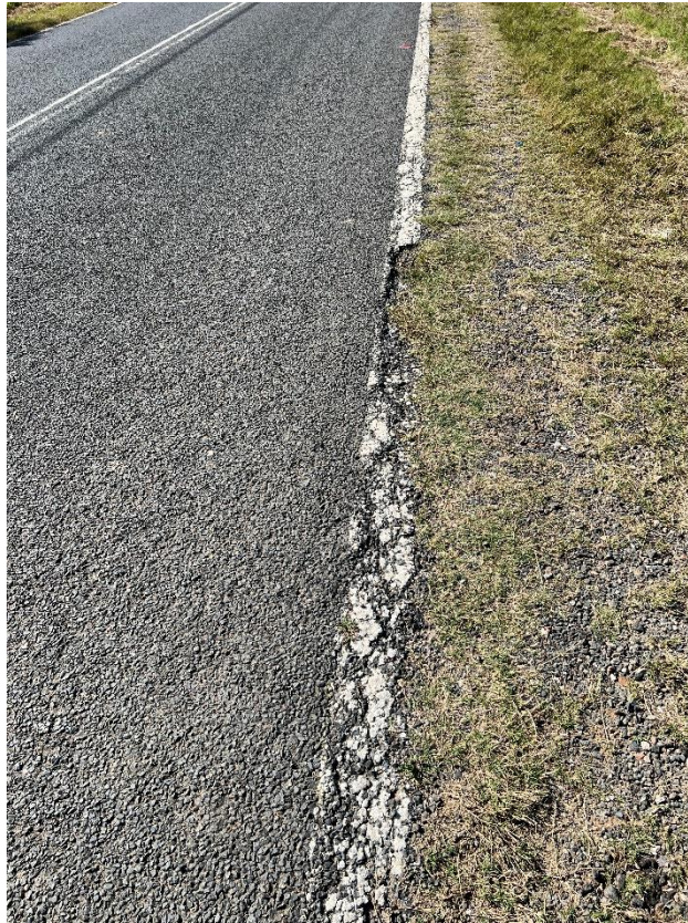
Figure 181 – Crack propagation to the road.
