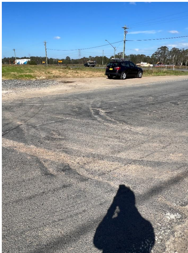
Figure 120 – Crack propagation to the road.
