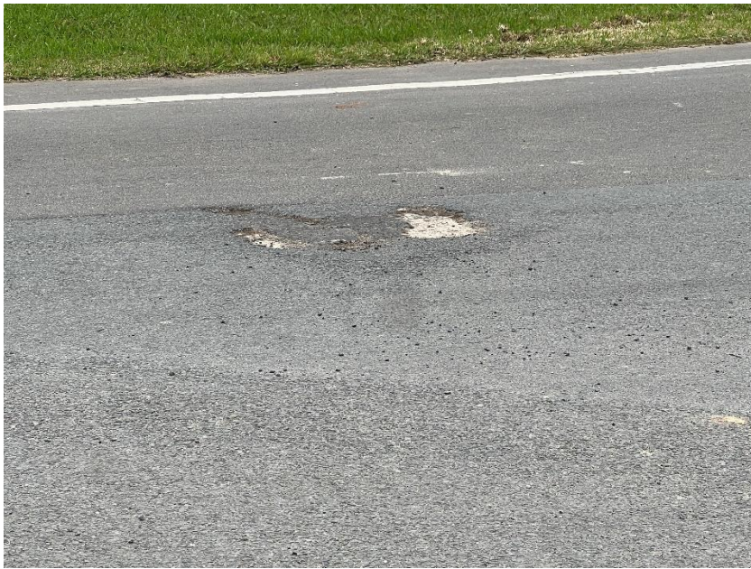
Figure 54 – Crack propagation to the road.
