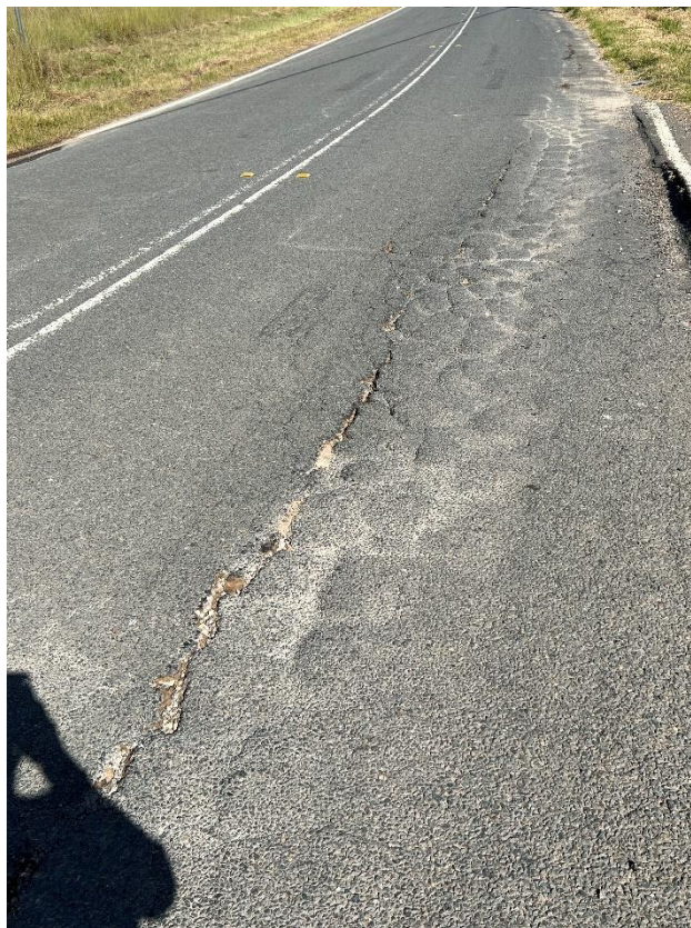
Figure 100 – Crack propagation to the road.
