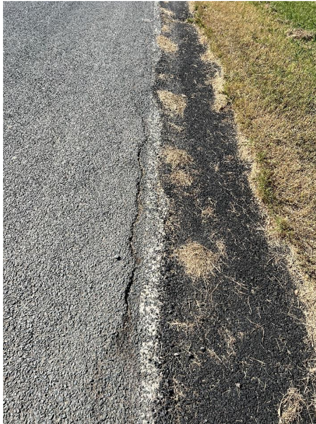
Figure 203 – Crack propagation to the road.
