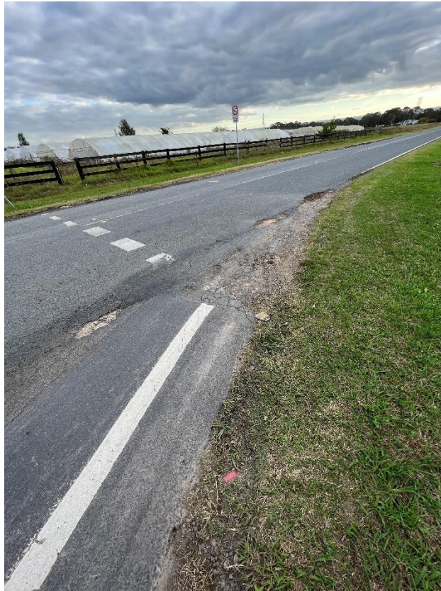
Figure 57 – Crack propagation to the road.
