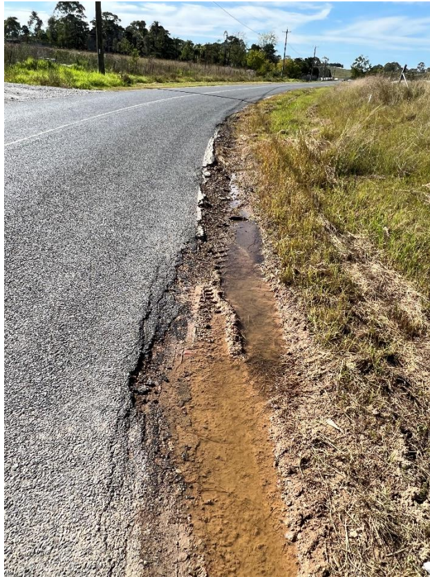
Figure 163 – Crack propagation to the road.
