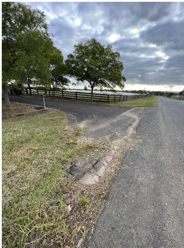
Figure 44 – Crack propagation to the driveway.
