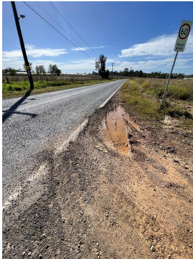
Figure 144 – Crack propagation to the road.
