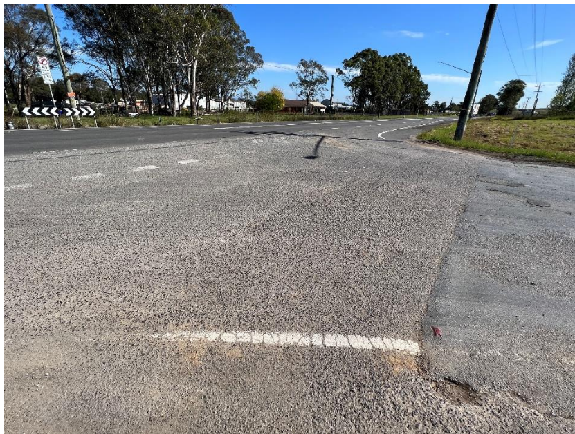
Figure 132 – Crack propagation to the road.
