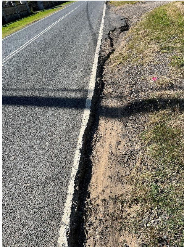
Figure 193 – Crack propagation to the road.
