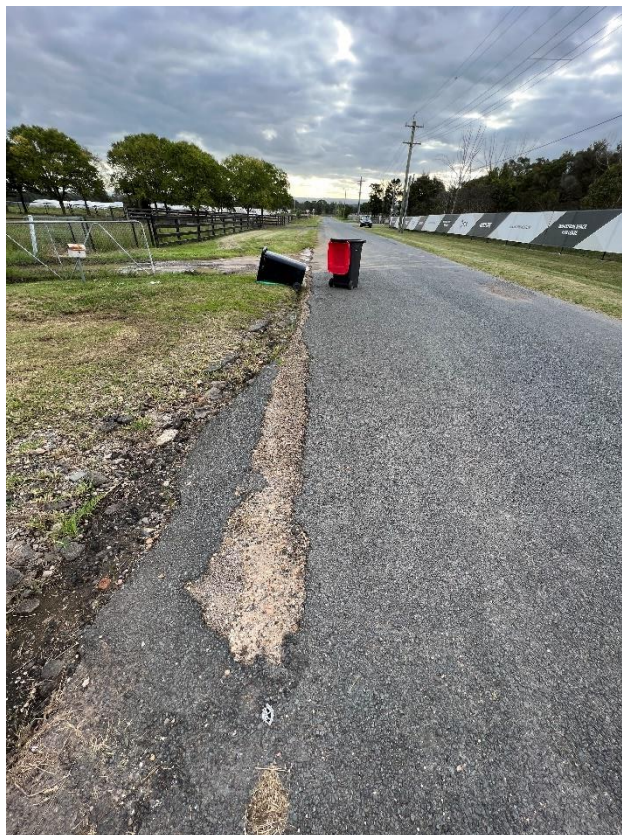
Figure 32 – Crack propagation to the road.
