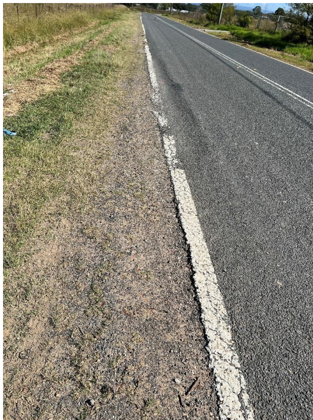
Figure 186 – Crack propagation to the road.
