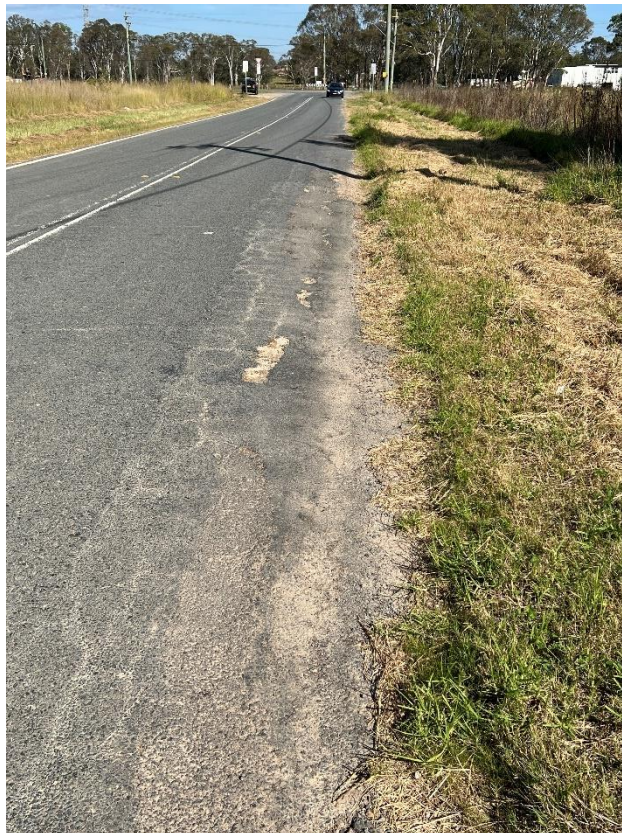
Figure 106 – Crack propagation to the road.
