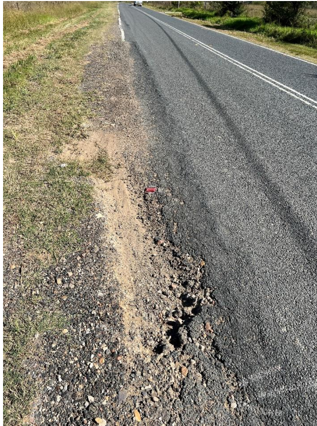
Figure 189 – Crack propagation to the road.
