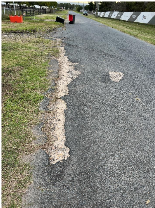
Figure 30 – Crack propagation to the road.
