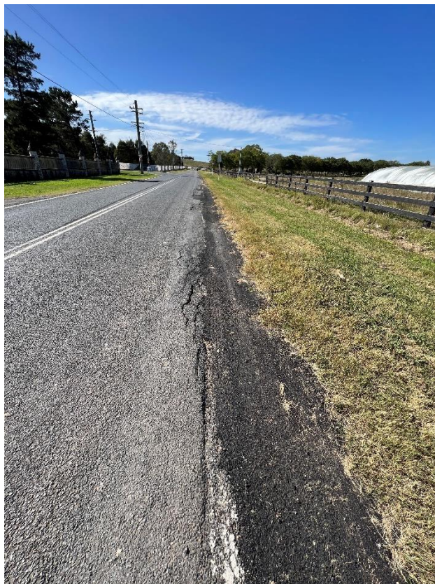
Figure 198 – Crack propagation to the road.
