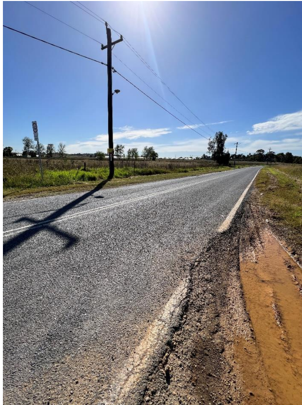
Figure 147 – Crack propagation to the road.
