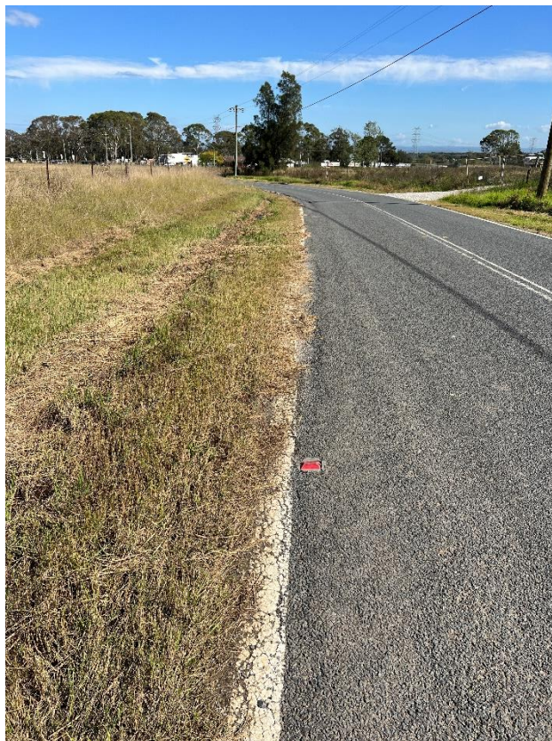
Figure 172 – Crack propagation to the road.
