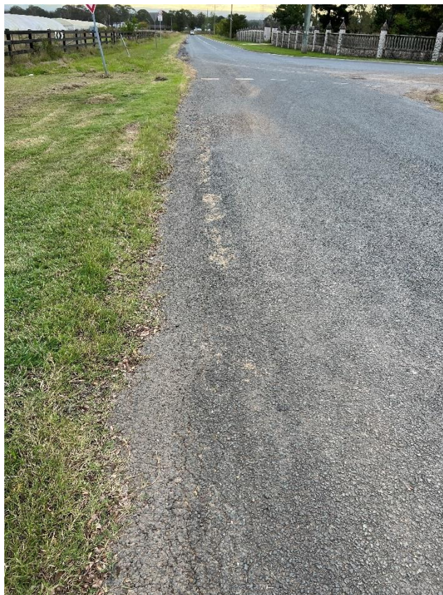
Figure 48 – Crack propagation to the road.
