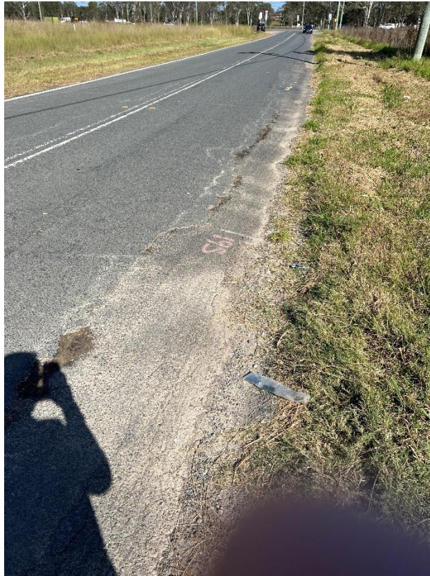
Figure 105 – Crack propagation to the road.
