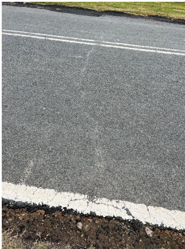
Figure 62 – Crack propagation to the road.
