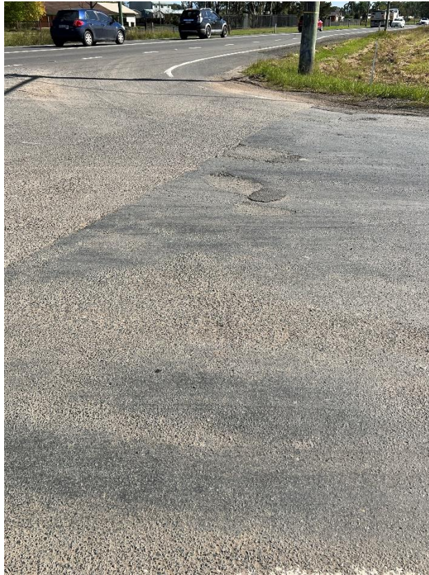
Figure 137 – Crack propagation to the road.
