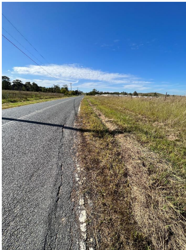
Figure 168 – Crack propagation to the road.
