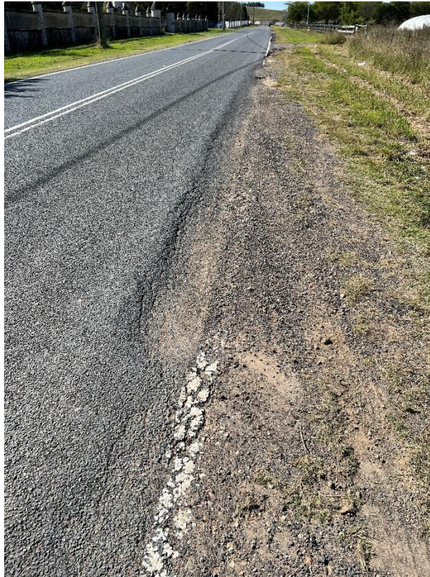
Figure 187 – Crack propagation to the road.
