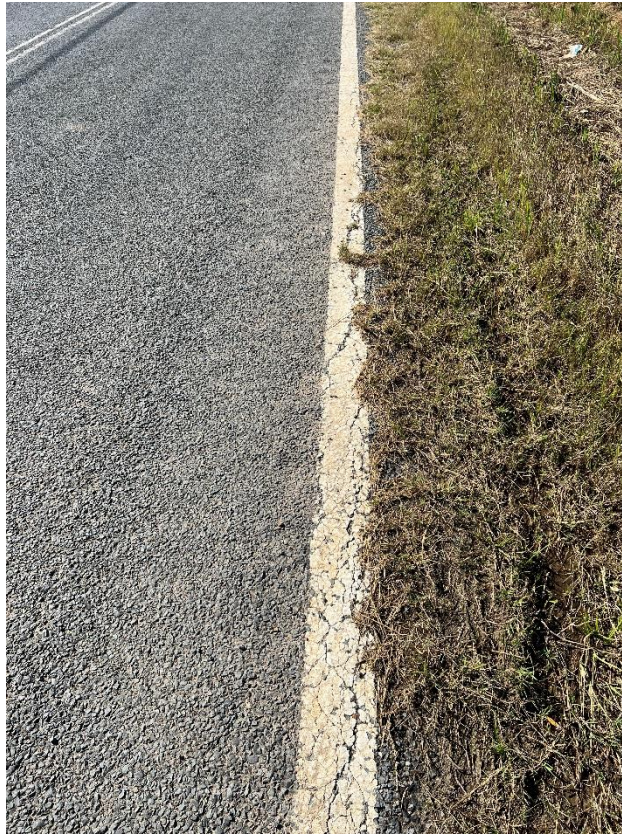
Figure 171 – Crack propagation to the road.
