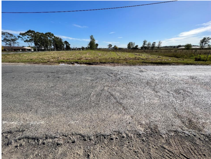
Figure 143 – Crack propagation to the road.
