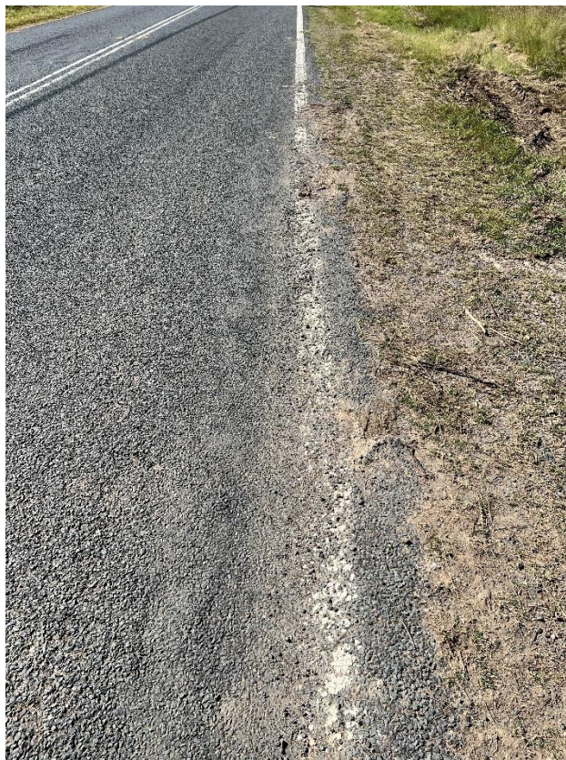
Figure 176 – Crack propagation to the road.
