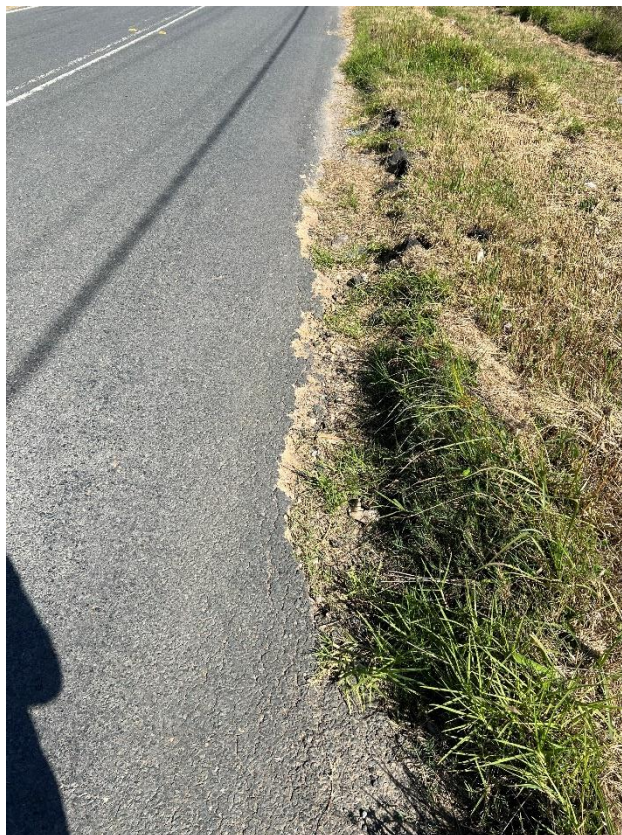
Figure 110 – Crack propagation to the road.
