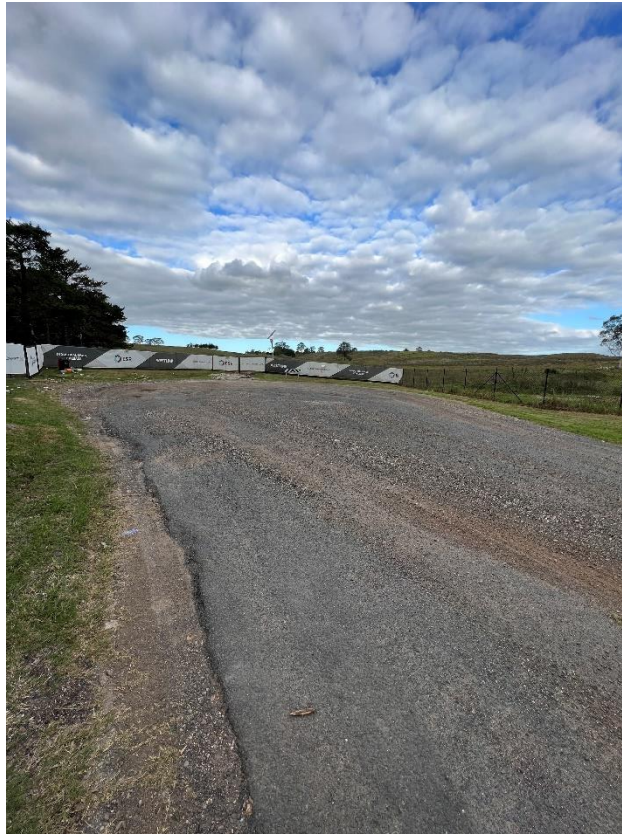
Figure 15 – Crack propagation to the road.
