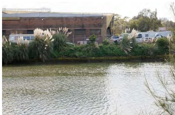
Figure 9. Alexandria Canal wall adjacent to 30 Burrows Road (Source: LOGOS, 2022)
