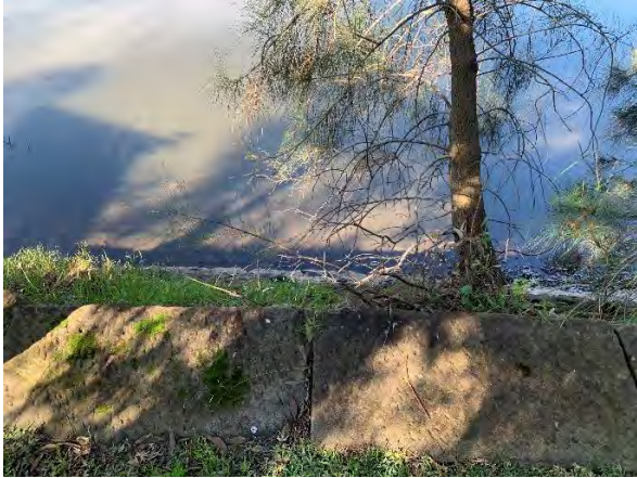
Figure 4. Sandstone capstone of Alexandria Canal Sandstone wall (Source: Artefact, 2022)
