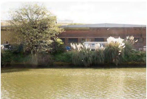
Figure 8. Alexandria Canal wall adjacent to 30 Burrows Road (Source: LOGOS, 2022)
