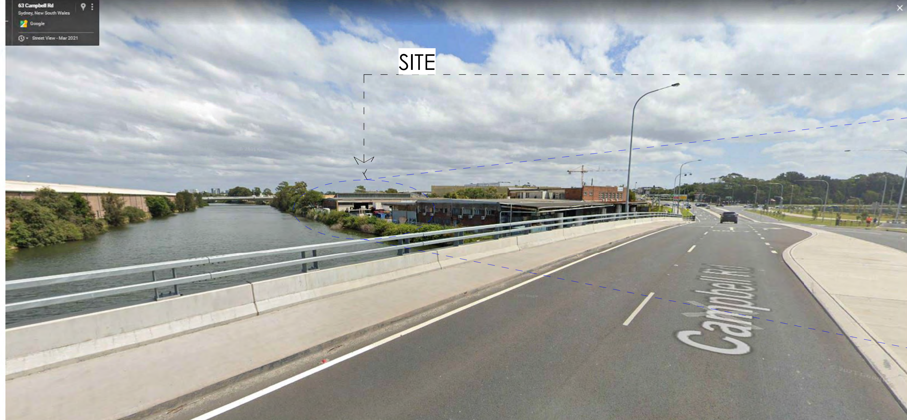
VIEW FROM NEW CAMPBELL BRIDGE TO SITE
