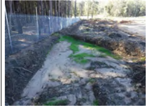
Example photo of a compacted mulch berm on steeper grade with an upslope facing groyne
