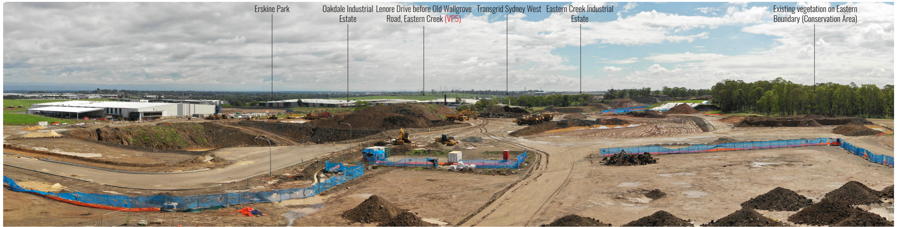
Figure 15: Drone at 104.1m RL Position 4 - Looking North
