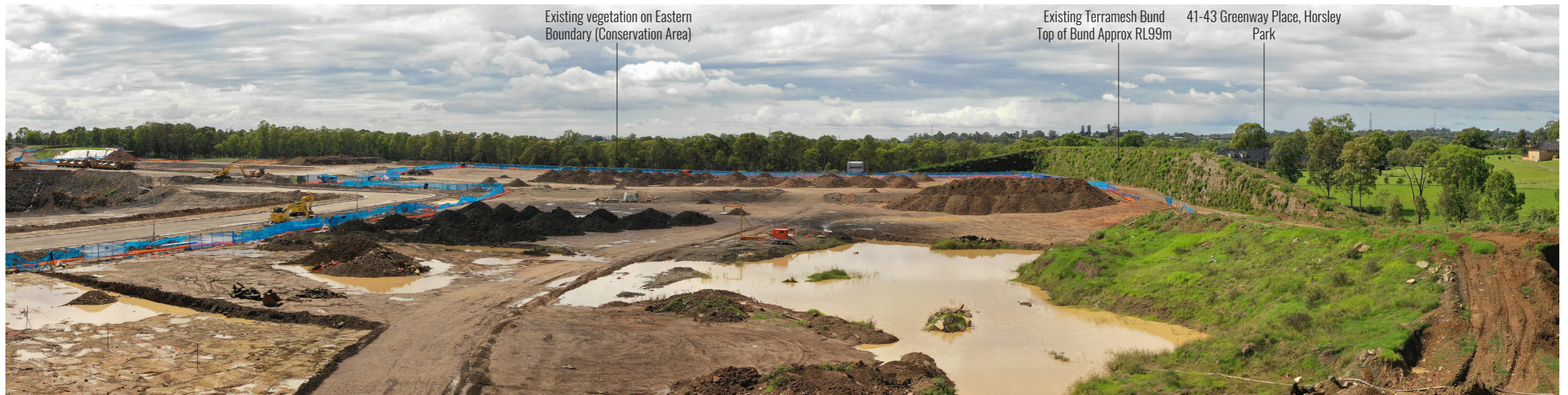
Figure 12: Drone at 101.5m RL Position 3 - Looking East
