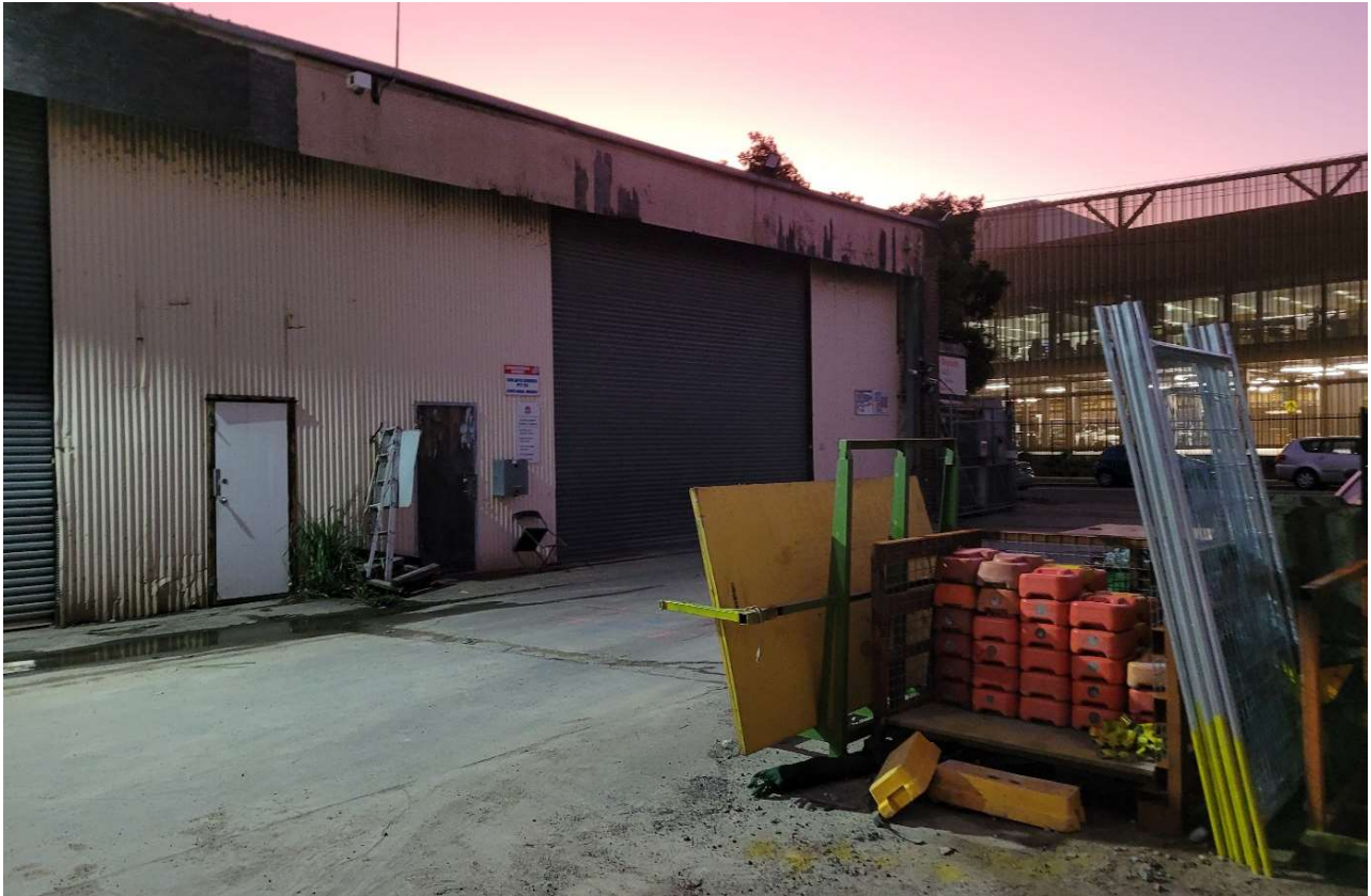
Photo 7 - General site photo looking North (26/07/2022)
