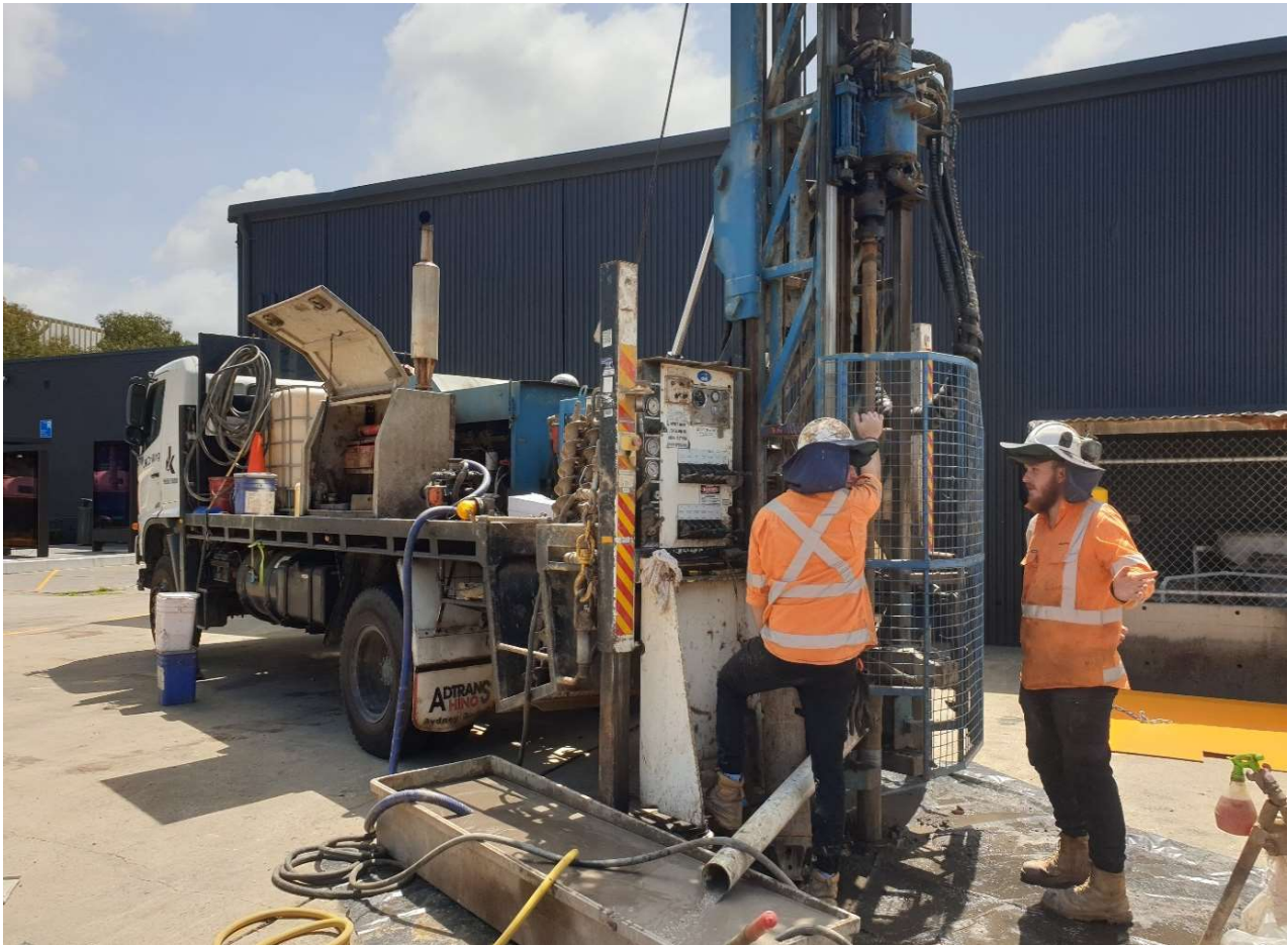
Photo 3 - Drill rig setup on BH01 (20/12/2021)
