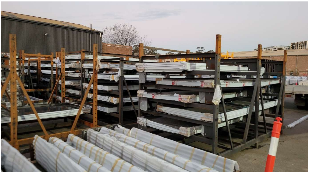
Photo 10 - Materials stored on site observed on 25/07/2022
