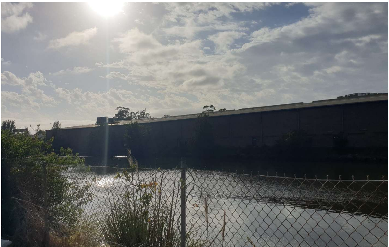
Photo 1 - Alexandra Canal near the southern boundary of the site (20/12/2021)
