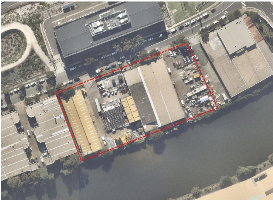
Inset 1: Nearmap Aerial Photograph of the site conditions on 17 May 2022 (Site boundary in Red)
