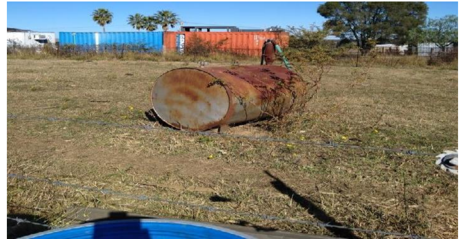
Photograph 26: Rusty above ground diesel storage tank, Lot 11
