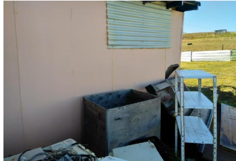
Photograph 10: Shed walls of corrugated metal and PACM, Lot 11
