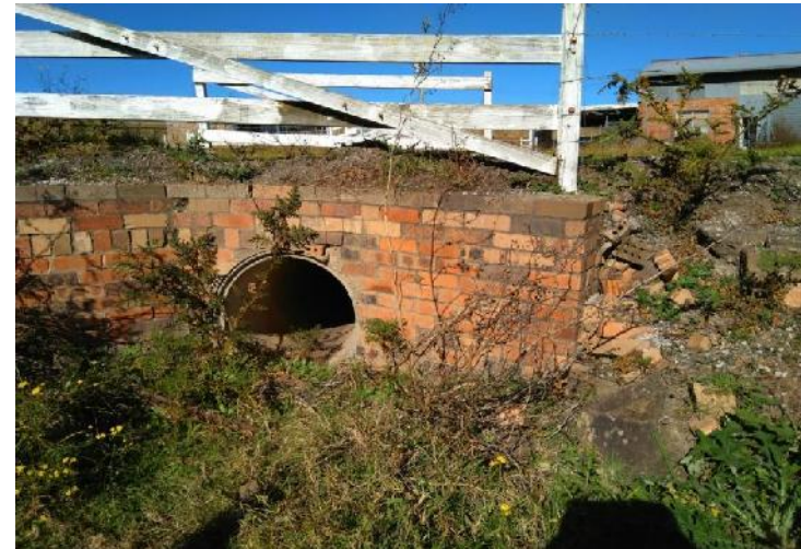
Photograph 50: A concrete drainage pipe and some surface debris of construction and demolition waste, located on Lot 12
