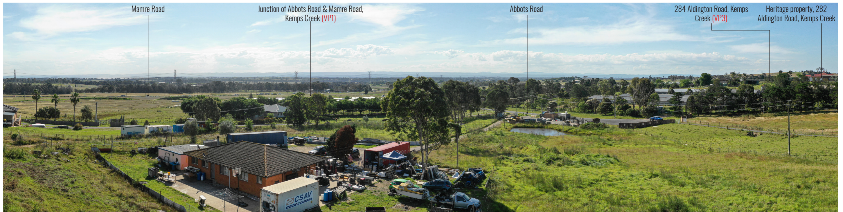
Figure 18: Drone at Position 4 - 14.6m APL - Looking West
