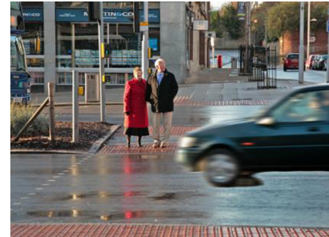
The five metre wide crossings provide adequate space on the central median to allow the crossings to be aligned with the pedestrian desire lines without the need for staggered crossings or guardrails. The crossings have restored a direct visual and psychological link across the busy road. Credit: Stephen McLaren.
