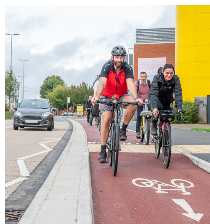
Protected cycle track along Multi-lane connector street.
