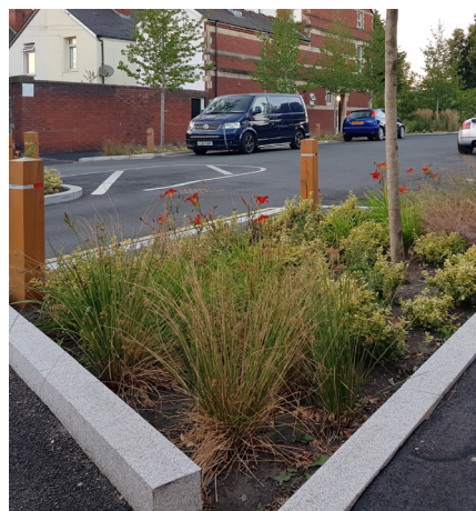
Rain garden. Credit: Mott Macdonald.
