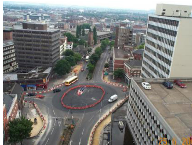
The selected design involved completely filling the subways and sunken plaza with concrete. Credit: Nottingham City Council
