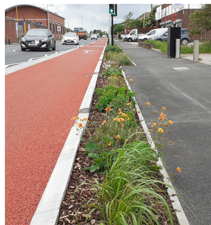
Rain gardens along cycle track.
