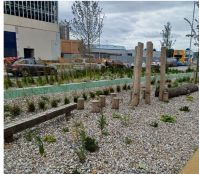
Kingsway, Stretford. Credit: United Utilities
