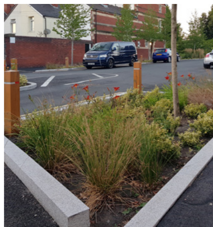
Rain garden. Credit: Mott Macdonald.
