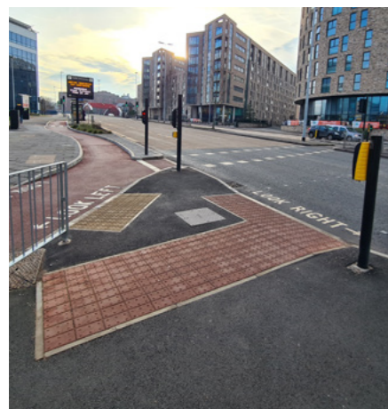
Crossings over a Multi-lane Connector Street and protected cycle track.
