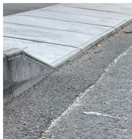
Ramped entrance kerb keeps footway at consistent level.
