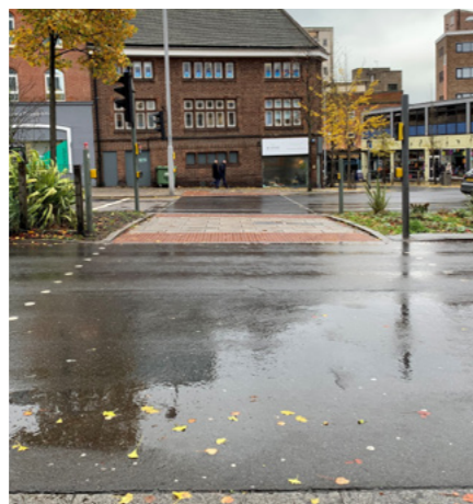
Wide crossing on desire line. Credit: Mott Macdonald.
