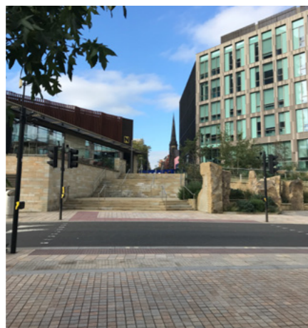
Wide controlled crossing on pedestrian desire line.
