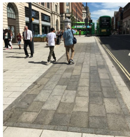
Footway level taxi bay.
