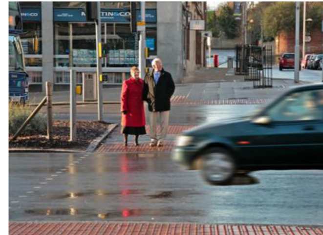
The five metre wide crossings provide adequate space on the central median to allow the crossings to be aligned with the pedestrian desire lines without the need for staggered crossings or guardrails. The crossings have restored a direct visual and psychological link across the busy road. Credit: Stephen McLaren.
