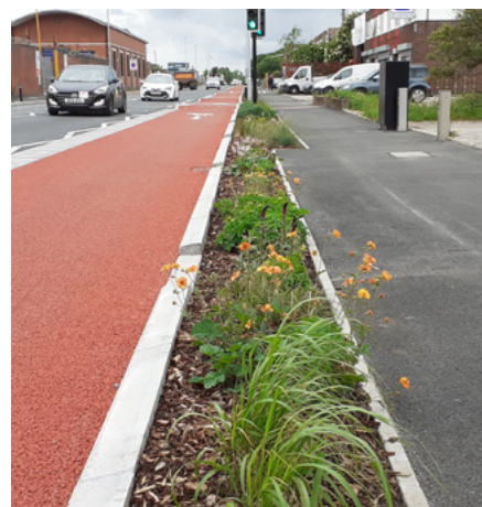
Rain gardens along cycle track.
