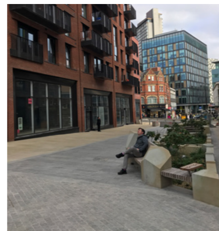
Street furniture integrated into SuDS features.
