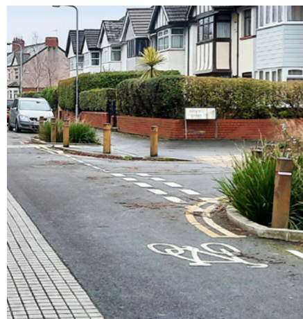
Local Connector Street / Neighbourhood gateway. Credit: Mott Macdonald.
